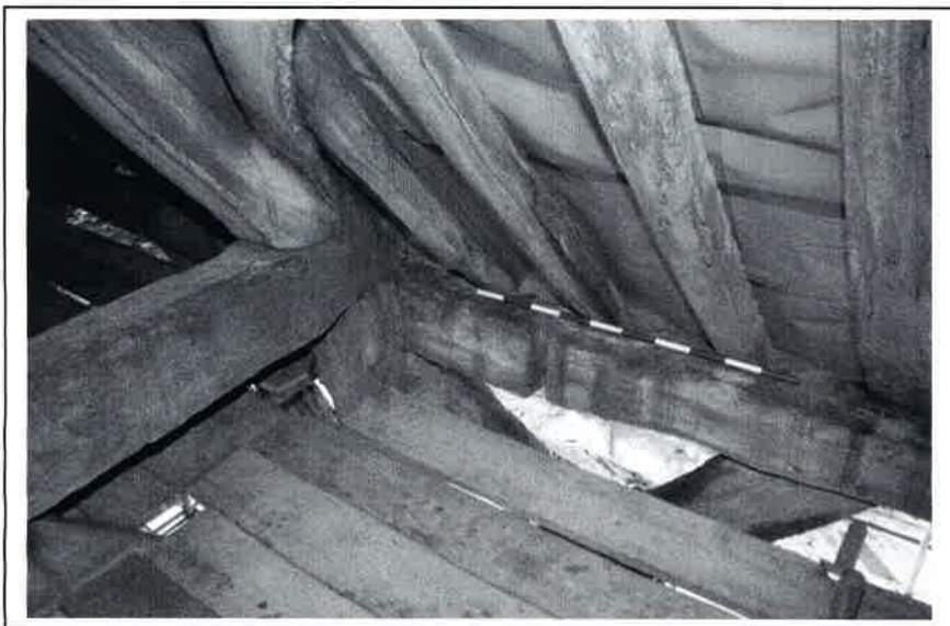
Plate 21: Mortise in upper face of west aisle tie. Frame III Plate 23: Detail at junction of tie-beam, arcade post, principal rafter South face of Frame II. Scarf to west of arcade plate.
