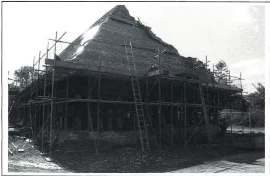
Plate 1: Barn during works viewed from north.
