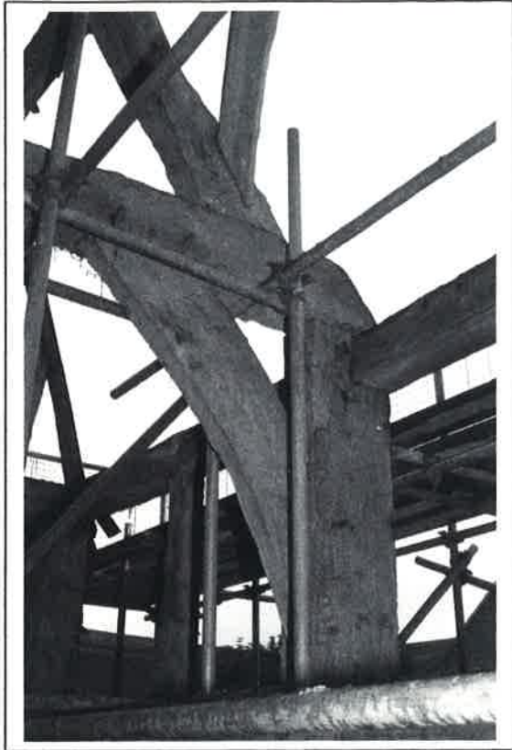
Plate 9: Aisle post, tie, rafter, brace at east end of Frame I
