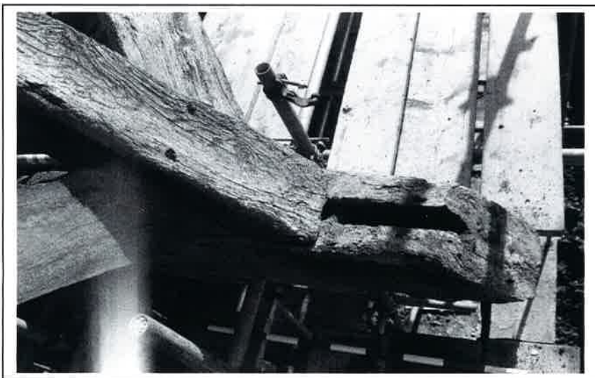
Plate 21: Mortise in upper face of west aisle tie. Frame III Plate 23: Detail at junction of tie-beam, arcade post, principal rafter South face of Frame II. Scarf to west of arcade plate.
