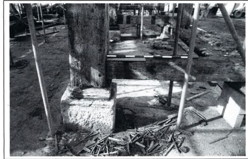
Plate 8: Stone base of main arcade post and lower tie to aisle. Frame III south face.
