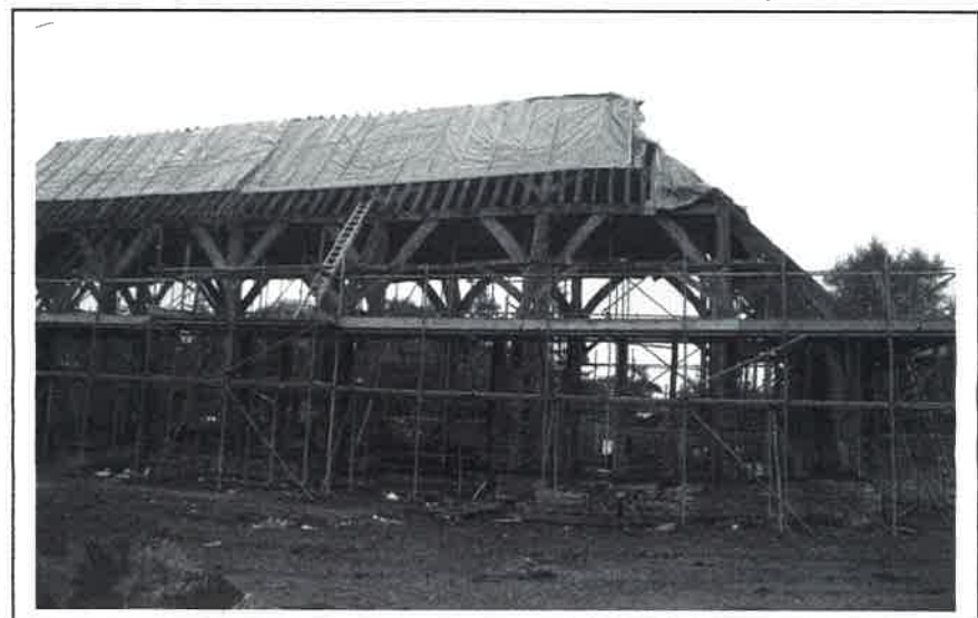
Plate 4: North end of east elevation during dismantling of aisles
