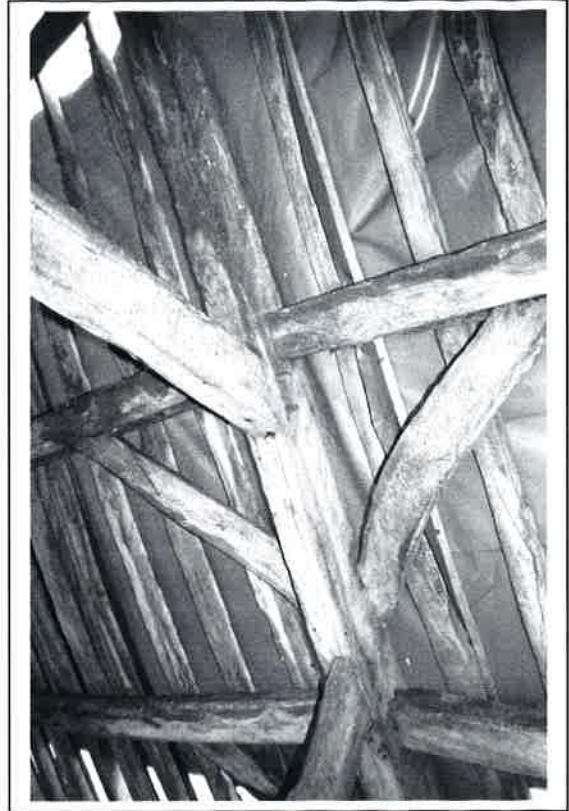
Plate 18: Detail at Frame V. Collar, 2 sets of purlins, principal rafter, strut, 2 wind braces.
