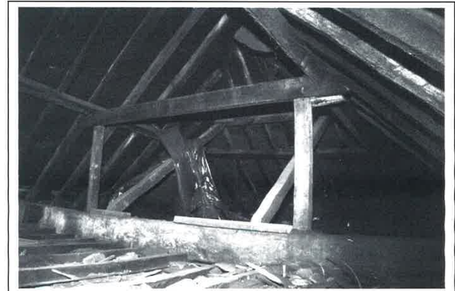
Plate 14: Queen post roof truss at south end of building
