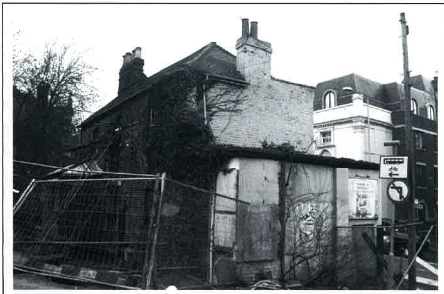
Plate 5: South elevation with secondary extension in foreground
