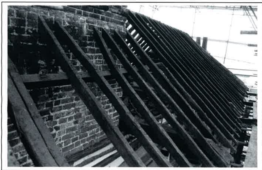
Plate 21: Trimming to rafters on west side of inserted chimney stack
