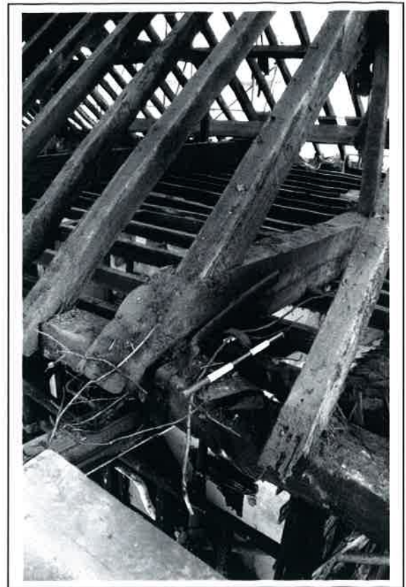
Plate 16: Tie-beam lapping over wall plate on west side of building.
