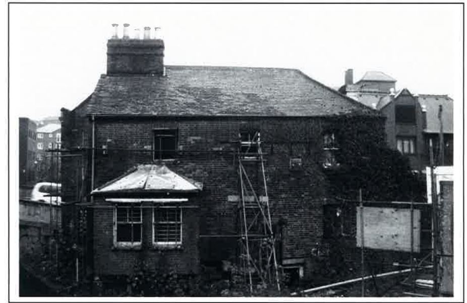
Plate 4: Rear (west) elevation
