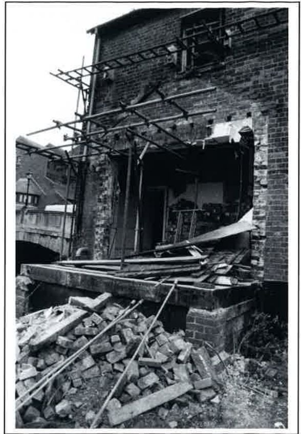
Plate 8: Outline of secondary bay which projected from west elevation after demolition
