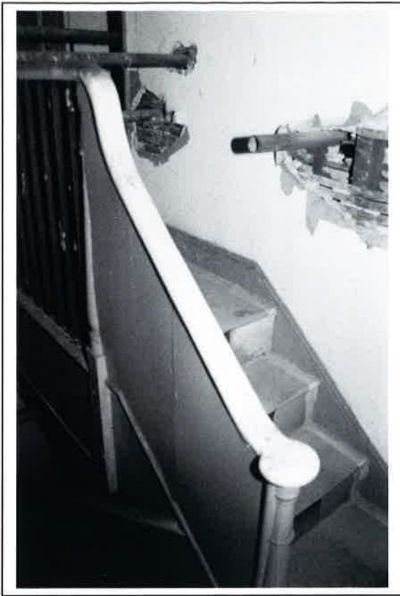
Plate 15: Swan-necked handrail and button-headed newel post within building
