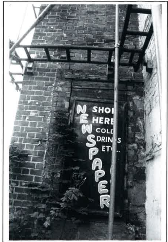
Plate 10: Outline of former lean-to, above shop sign in recess at north-west corner of building
