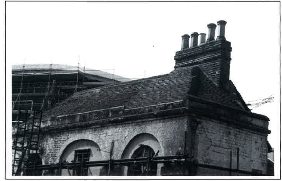
Plate 6: Roof from north-east showing off-centre chimney stack
