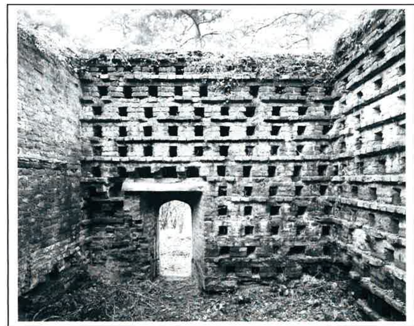
Plate 2: East elevation of smaller dovecote. Note rebuilt corner to left. Plate 4: Interior of smaller dovecote. Secondary wall to left
