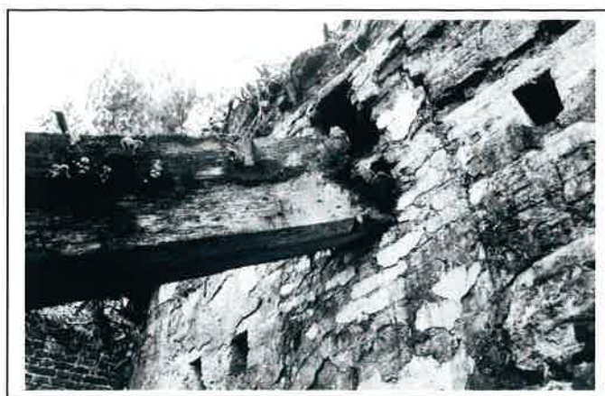
Plate 8: Chamfered underside of first floor principal joist
