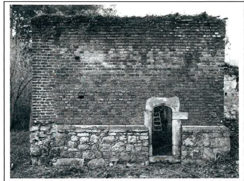
Plate 2: East elevation of smaller dovecote. Note rebuilt corner to left. Plate 4: Interior of smaller dovecote. Secondary wall to left
