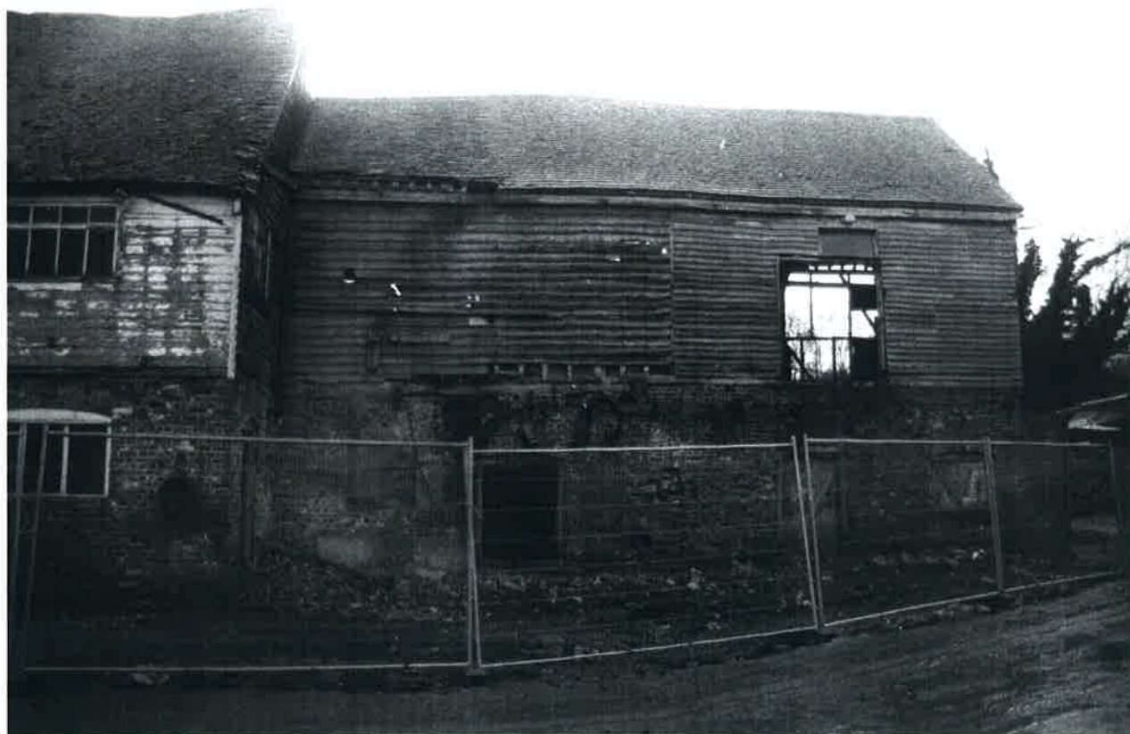
Plate 7 West elevation of barn.
