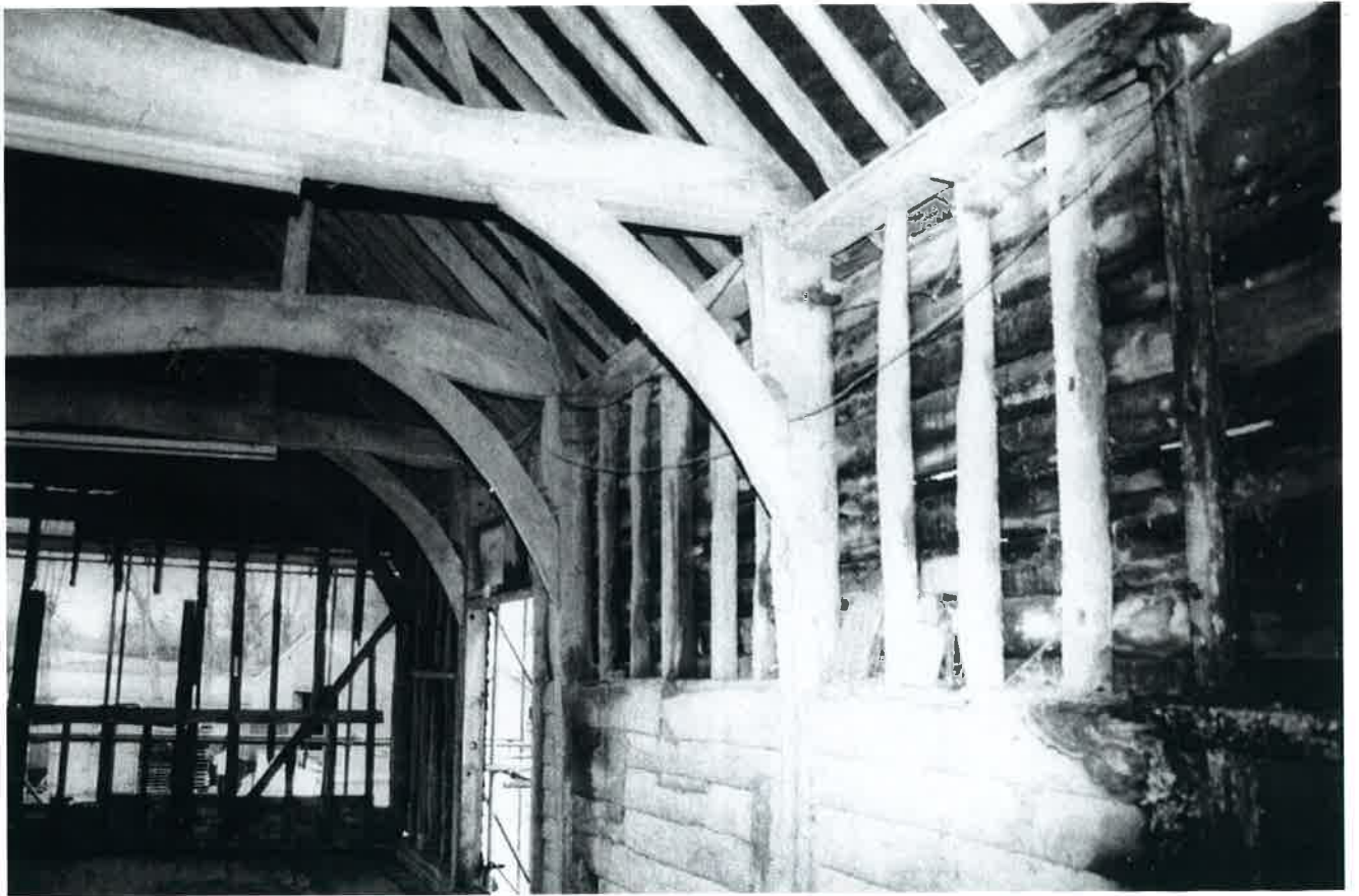
Plate 27 Wall framing and truss post within barn.
