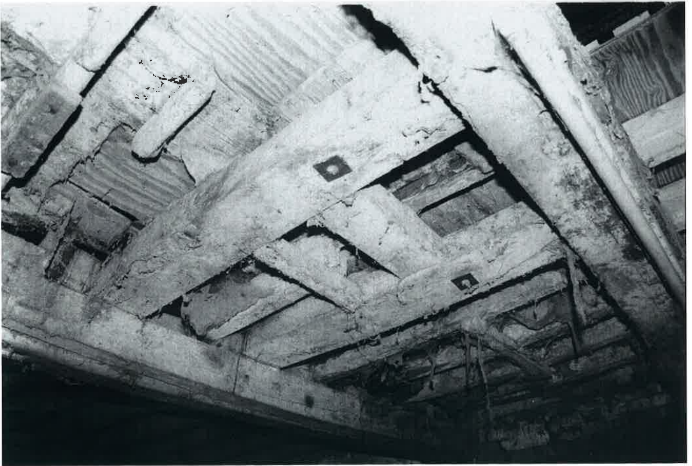
Plate 10 Underside of mill stone bearers within mill.
