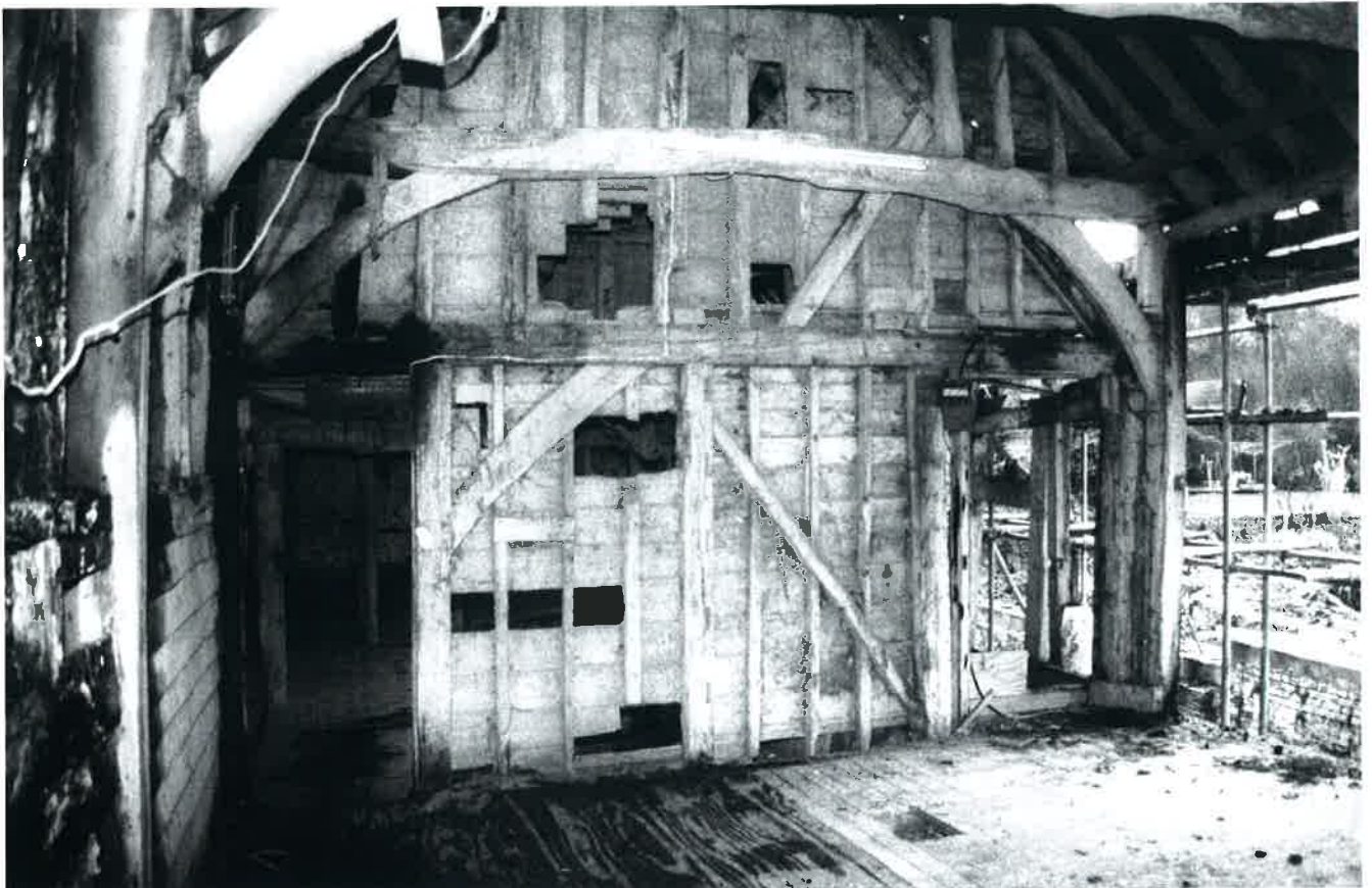
Plate 28 North end cross frame within barn (F10).
