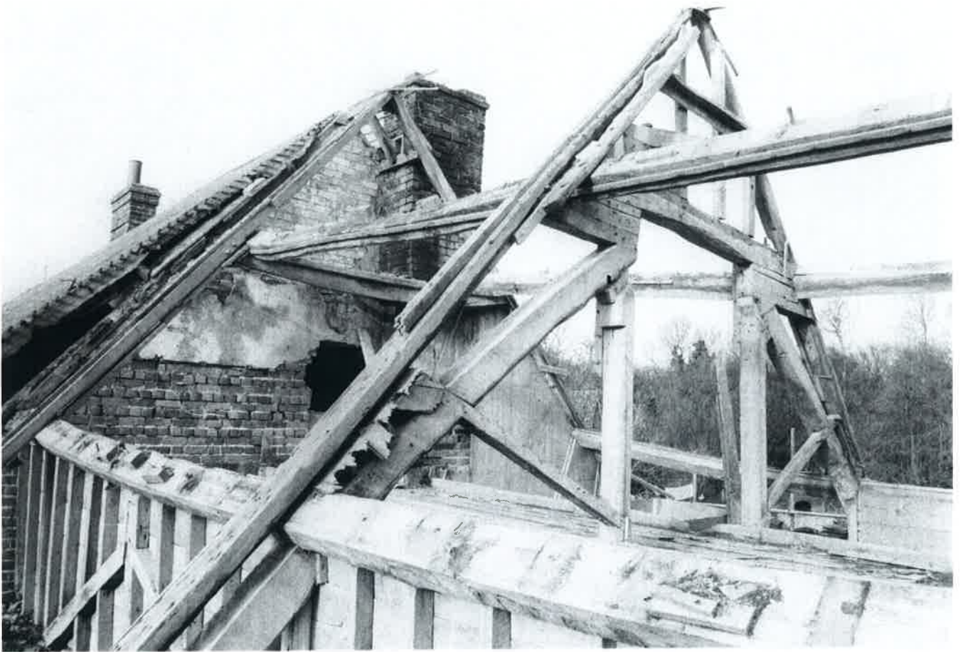
Plate 19 Truss above mill during roof works.
