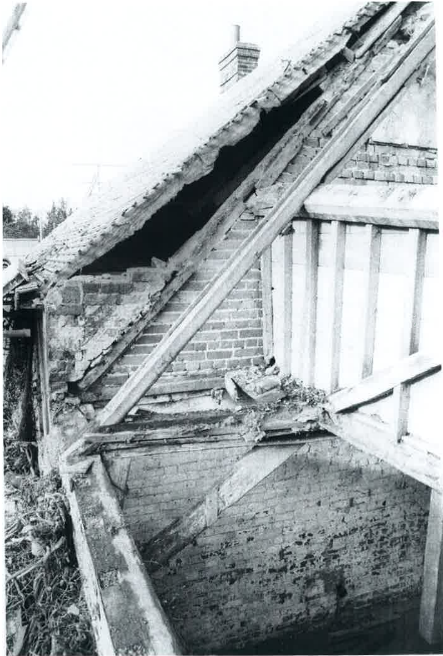
Plate 18 View during removal of mill roof.
