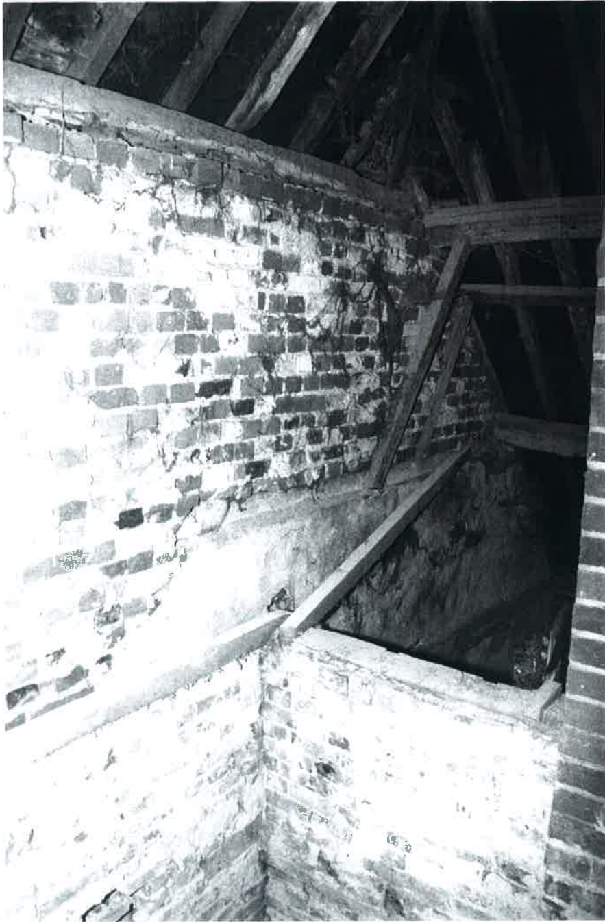
Plate 21 Imprint of former roof on north wall of mill house.
