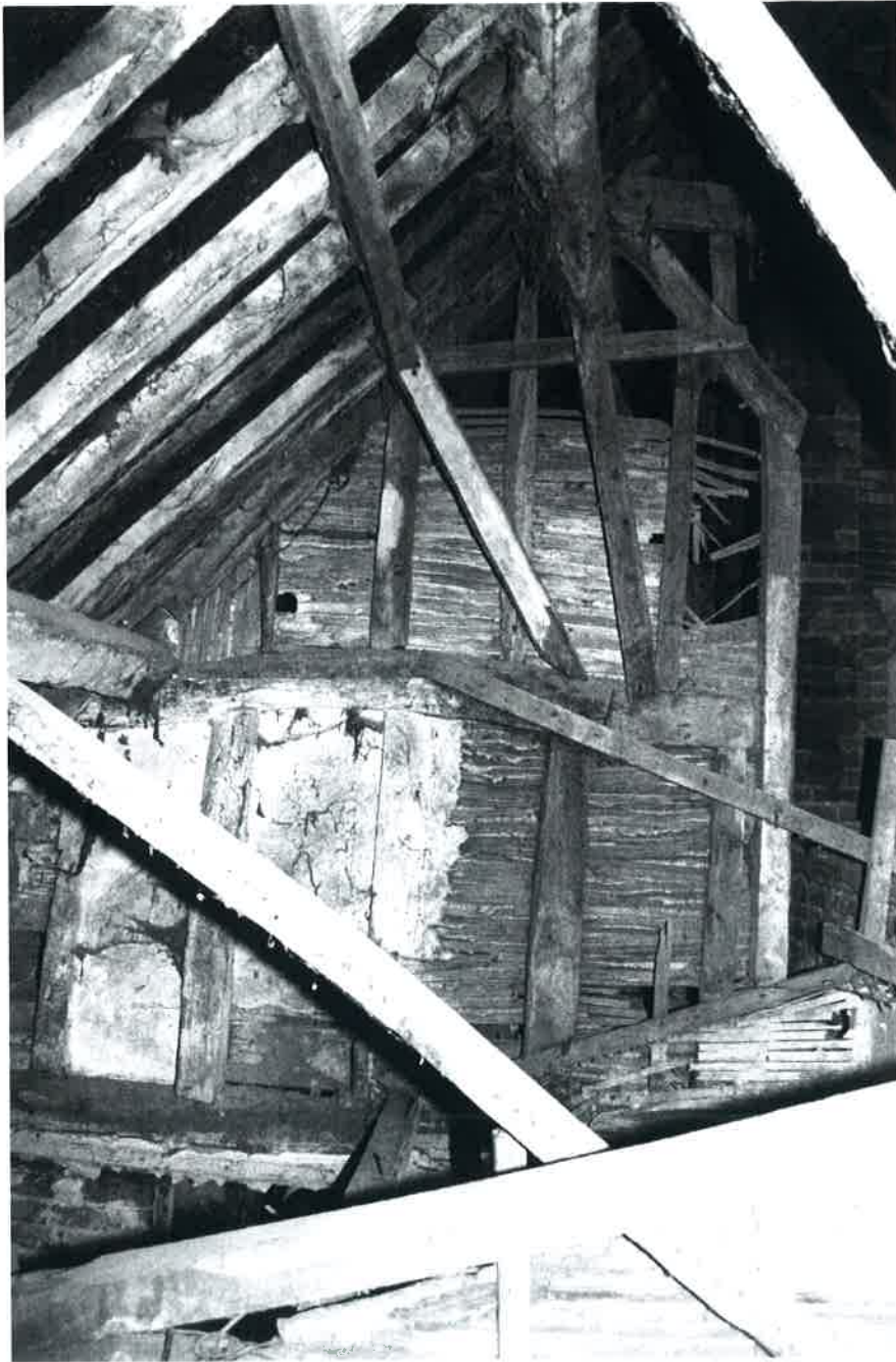
Plate 22 Surviving truss and cross frame above wall between F7 and F8.
