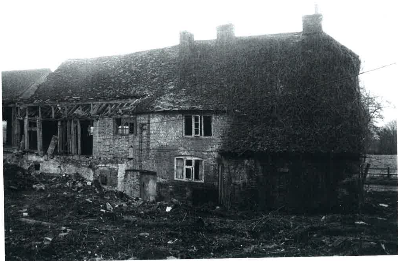
Plate 5 East elevation of mill house.
