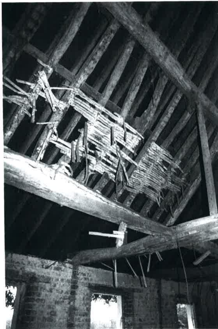
Plate 24 Rafters of earlier building enclosed within roof of mill house
