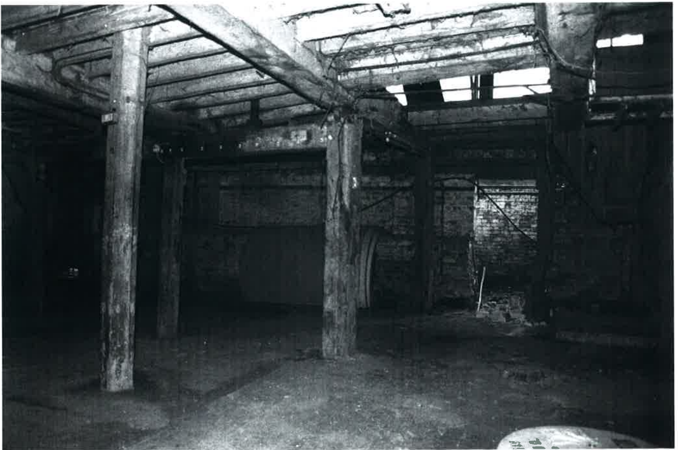
Plate 11 General view from west within ground floor of mill (G9)
