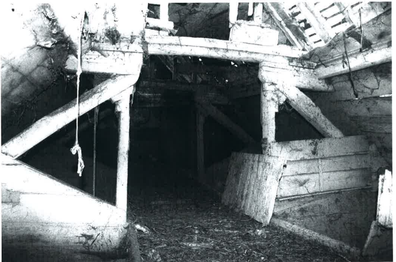
Plate 17 Second floor of mill.
