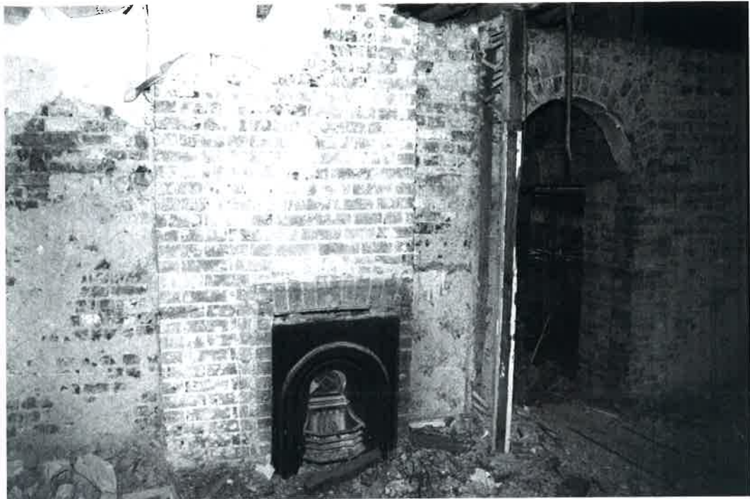
Plate 23 First floor fireplace within secondary spine in mill house
