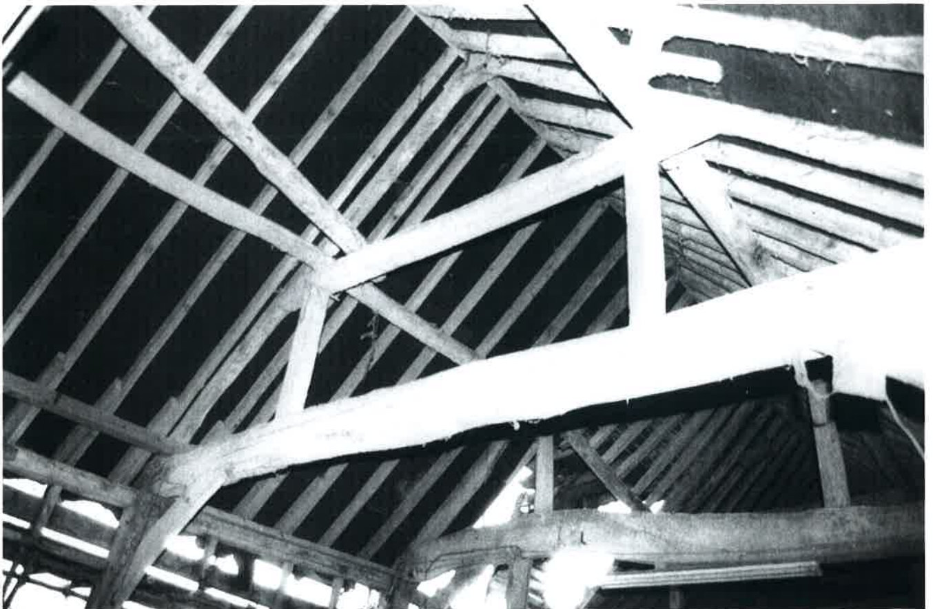
Plate 26 Typical truss within barn (F10).
