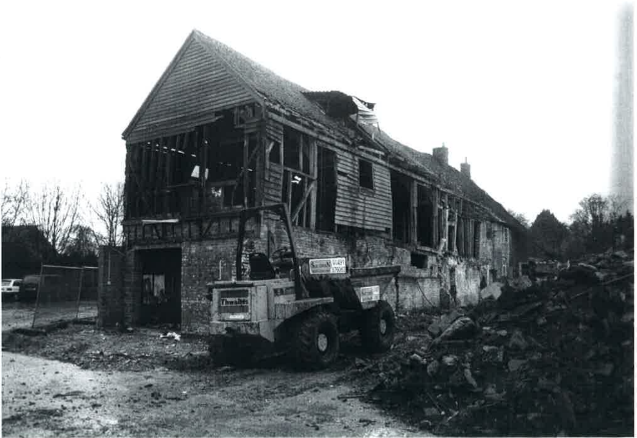
Plate 1 General view from south-east.
