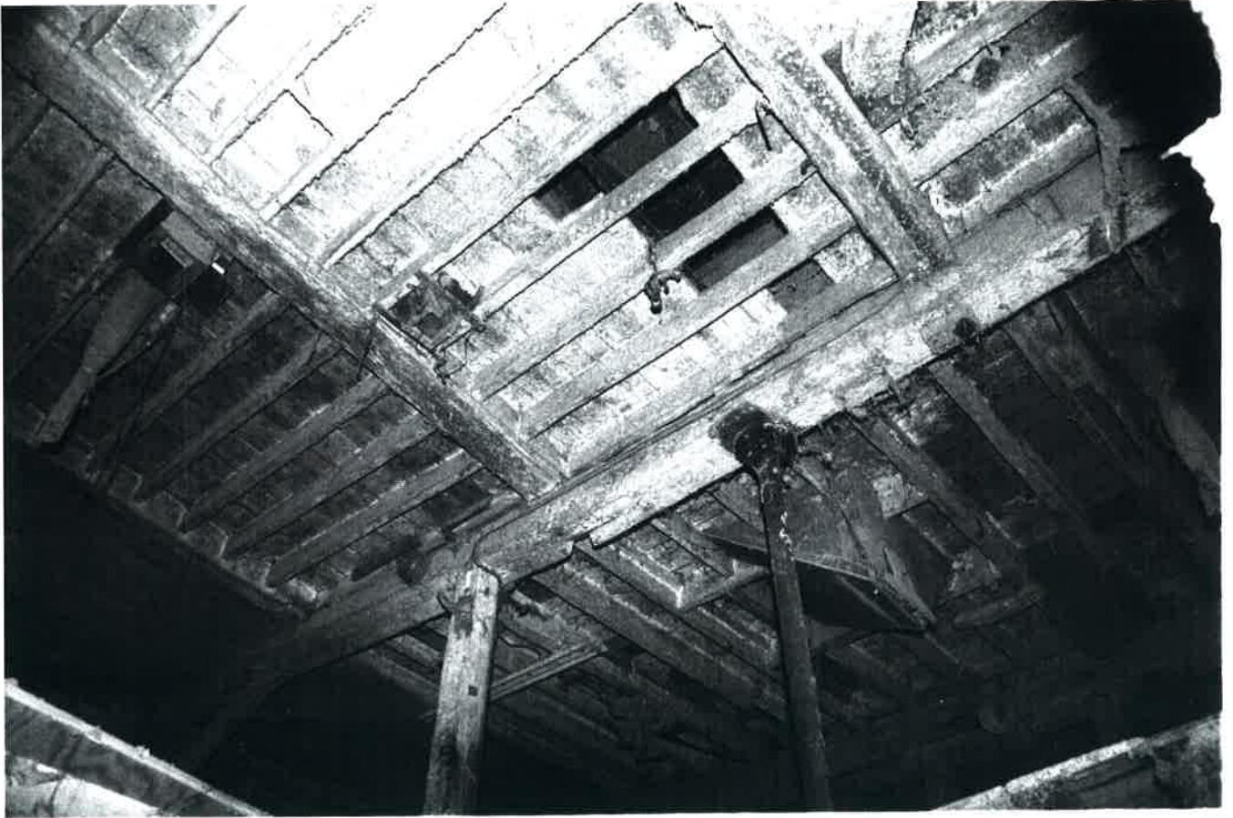
Plate 16 Underside of second floor of mill. Note top shaft reused as prop.
