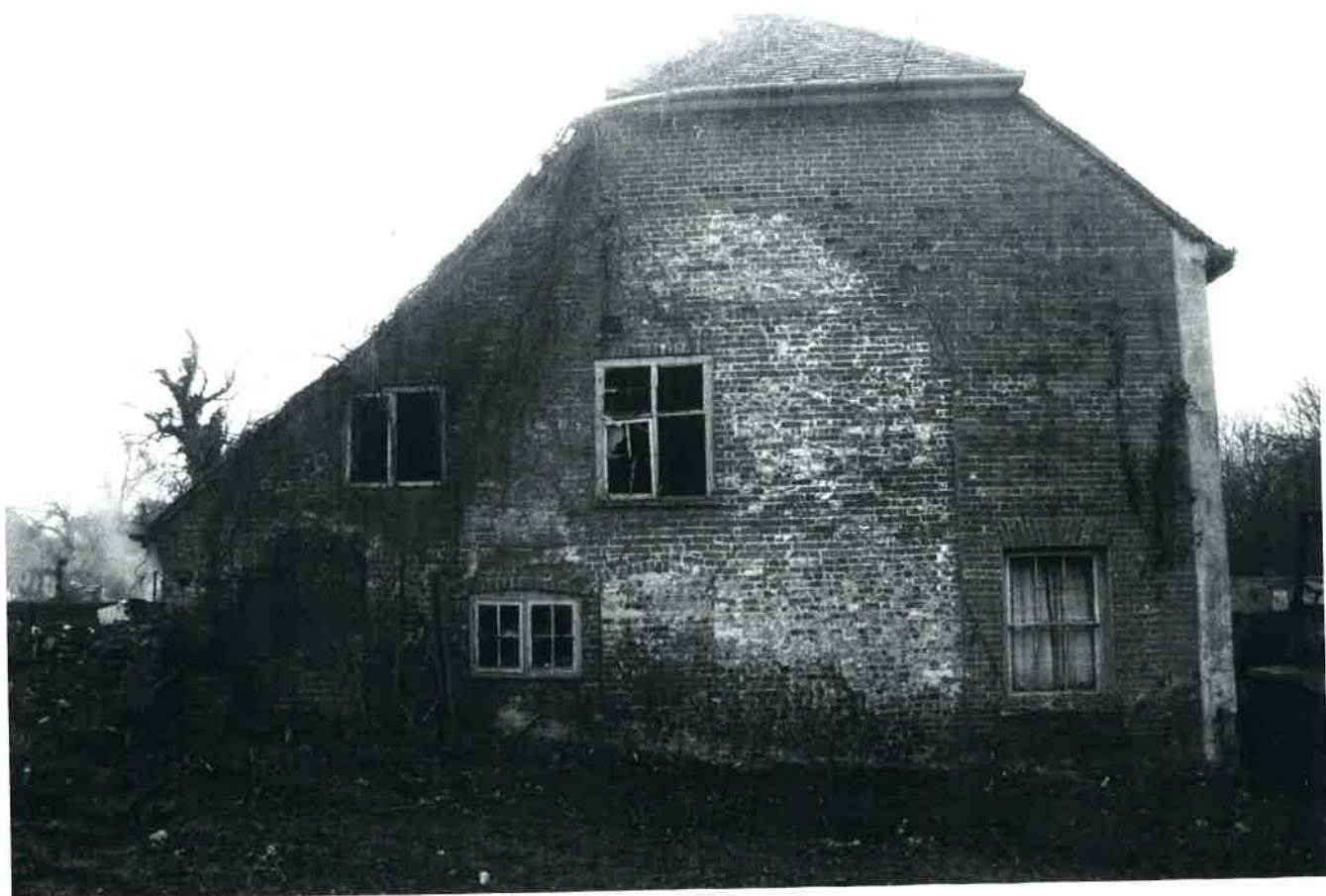
Plate 6 North elevation of mill house.
