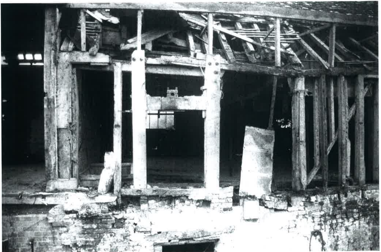
Plate 4 Power shaft bearing frame in east wall of mill.
