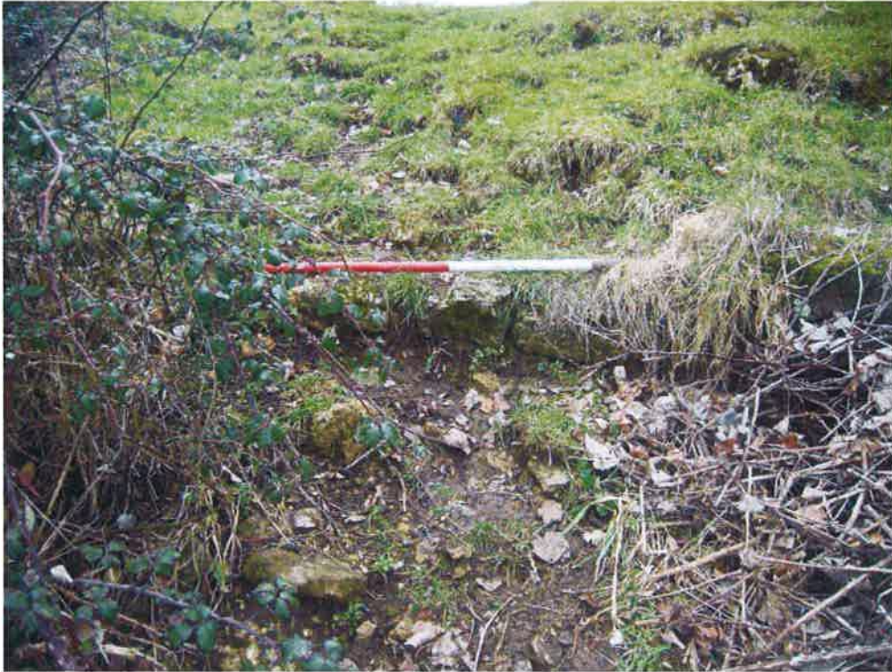
Photograph 9: Pathway erosion on feature 17, revealing coursed stonework.
