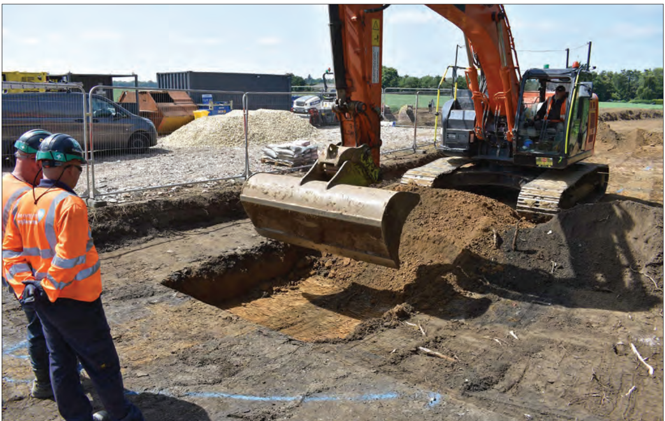
Plate 4: Digging for the manhole
