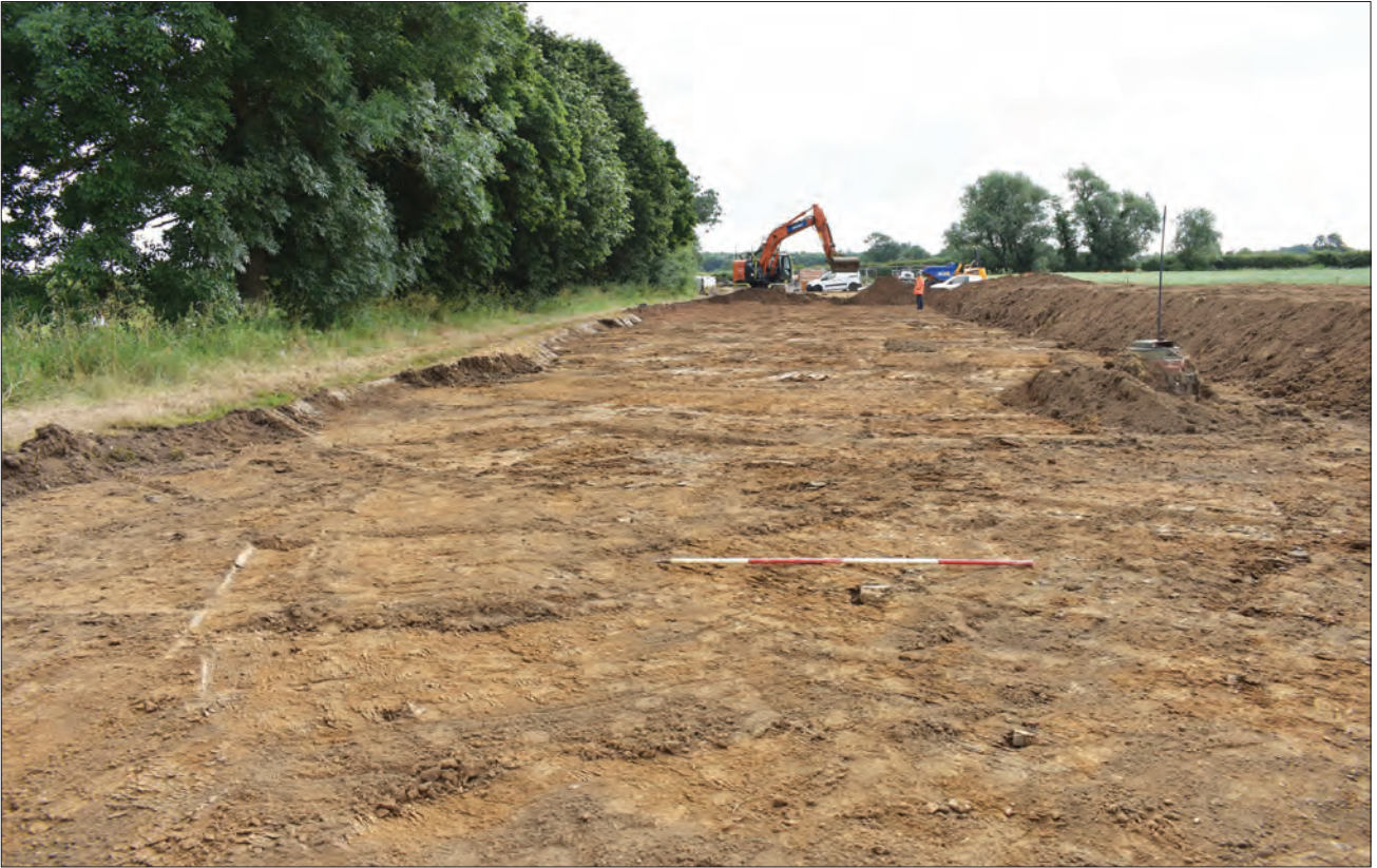
Plate 1: Topsoil stripping
