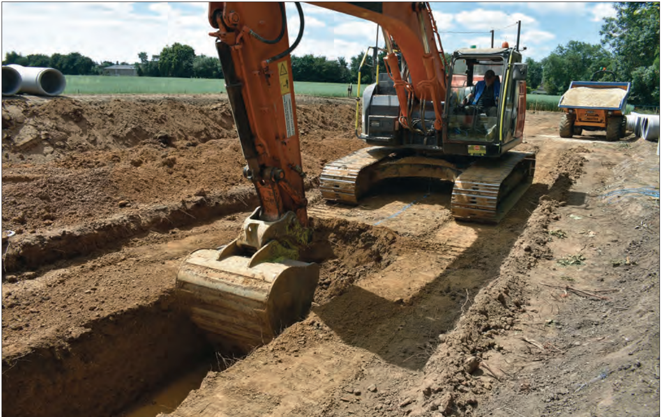
Plate 3: Digging the line of the pipe trench
