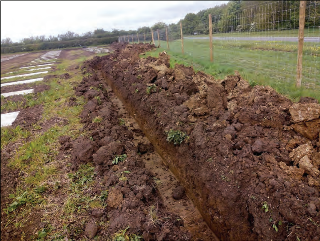
Plate 1: Cable trench adjacent to B661, looking north-west
