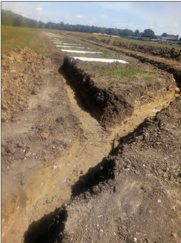
Plate 2: Cable trench on southern side of site, looking south-east
