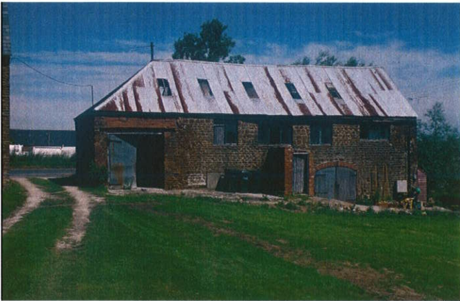
Plate 6: Block F from the south
