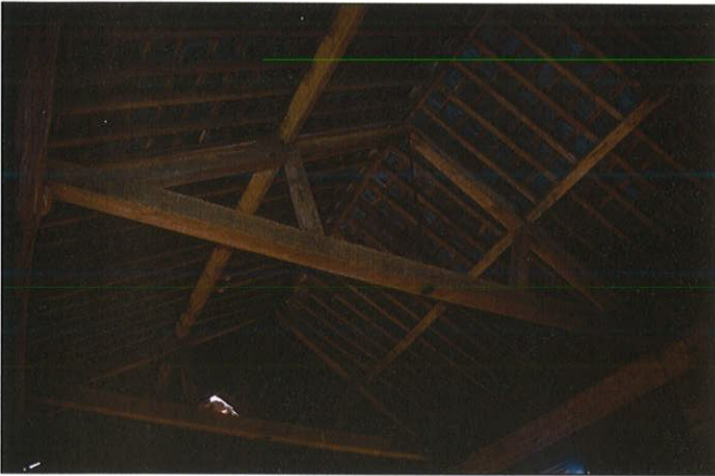
Plate 2: Internal view of Block A truss
