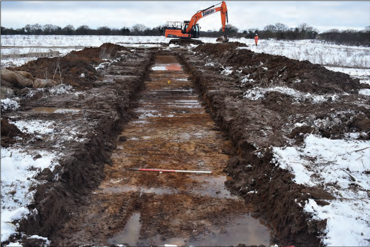
Plate 5: Trench 55 from the north-east
