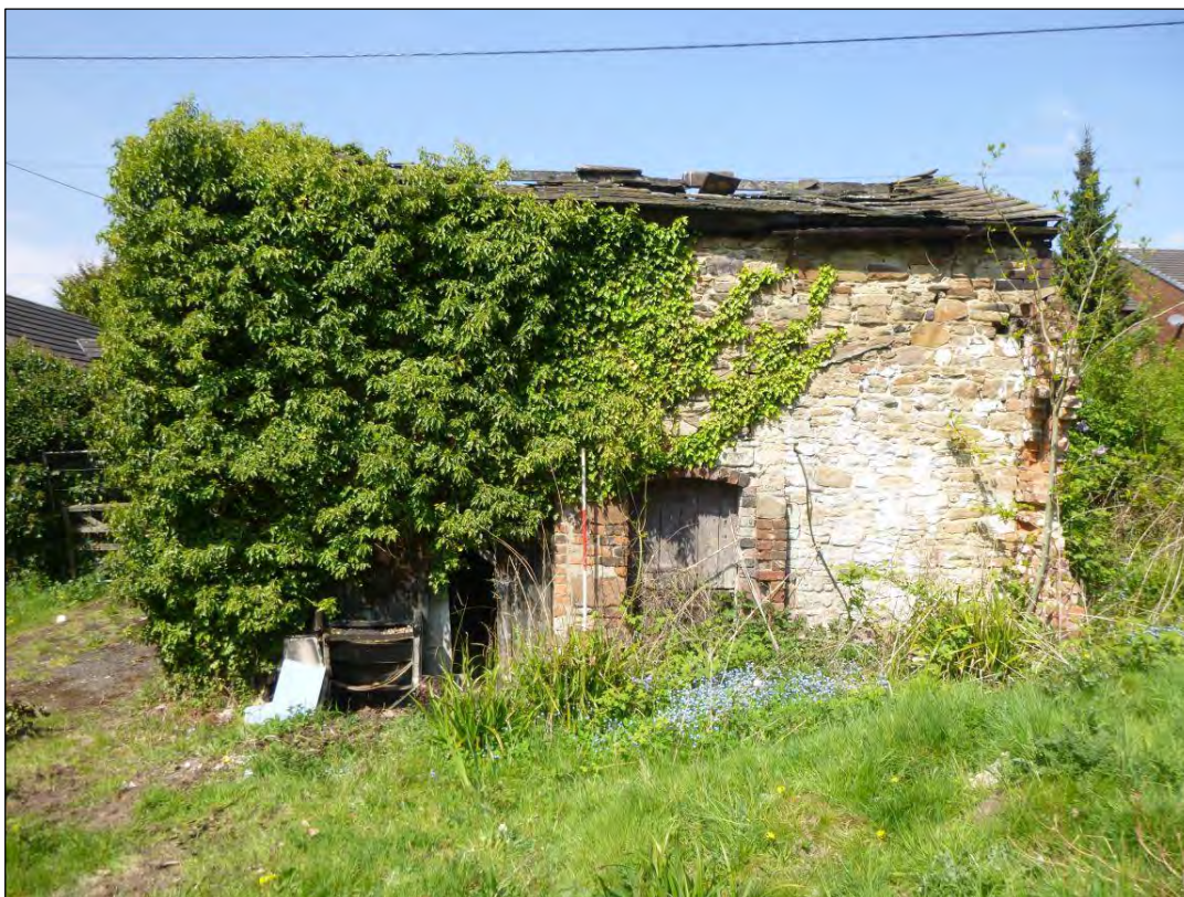
Plate 9: Eastern elevation of Carr Cottage outbuilding, scale 2m
