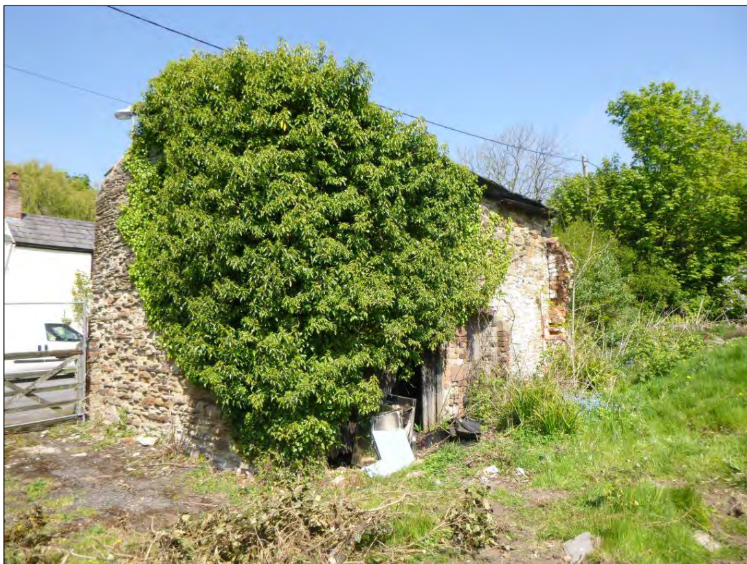
Plate 6: Overview of the Carr Cottage outbuilding, looking north
