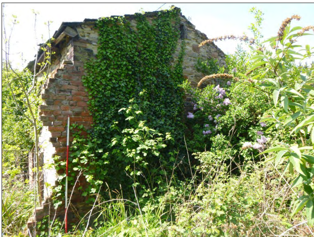
Plate 12: Northern elevation looking south-west, scale 2m
