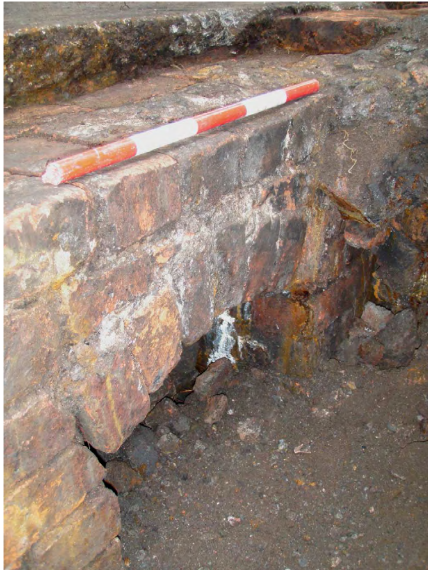
Plate 22: Trench 11, showing arched-brick aperture 1114 within wall 1106
