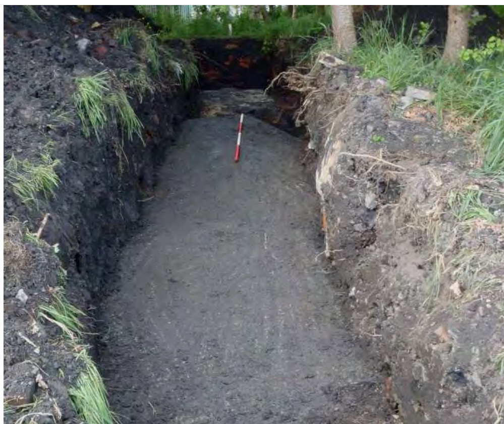
Plate 20: Trench 10, showing surface 1002 at the south-western end of the trench
