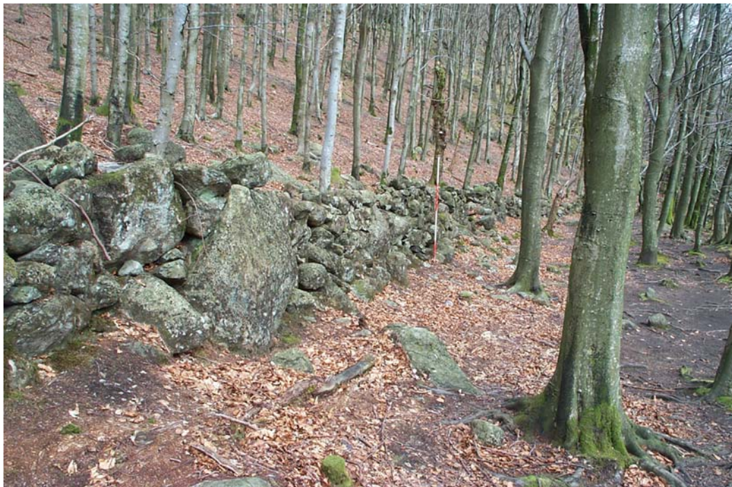
Plate 8: A section of orthostatic dry-stone wall (Site 53)
