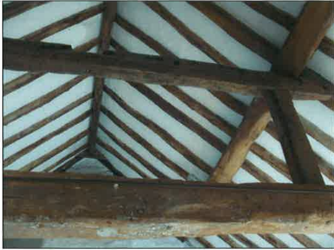
Plate 19: Back hall, main roof truss
