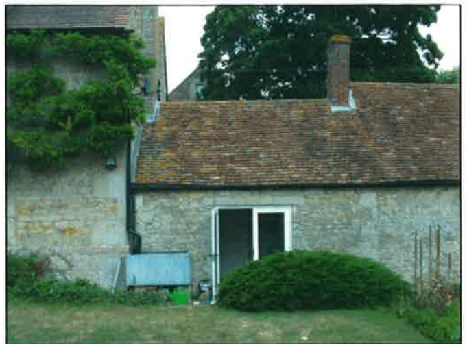
Plate 4: Back hall, rear elevation
