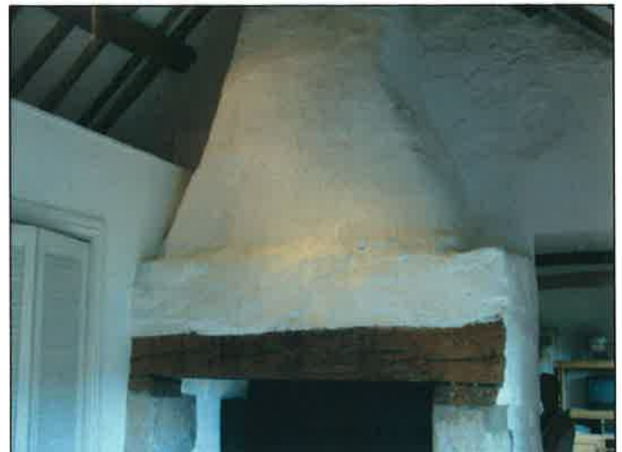
Plate 18: Back hall, tapering chimney breast
