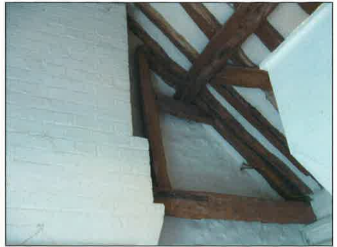
Plate 20: Back hall, later chimney and truncated and altered roof truss
