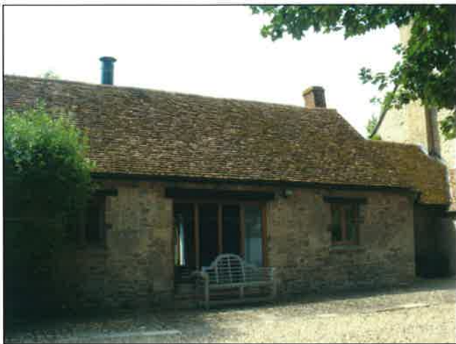
Plate 3: Former barn or stable, front elevation
