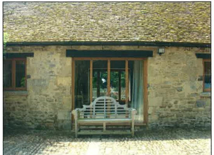
Plate 6: Former barn or stable front door opening
