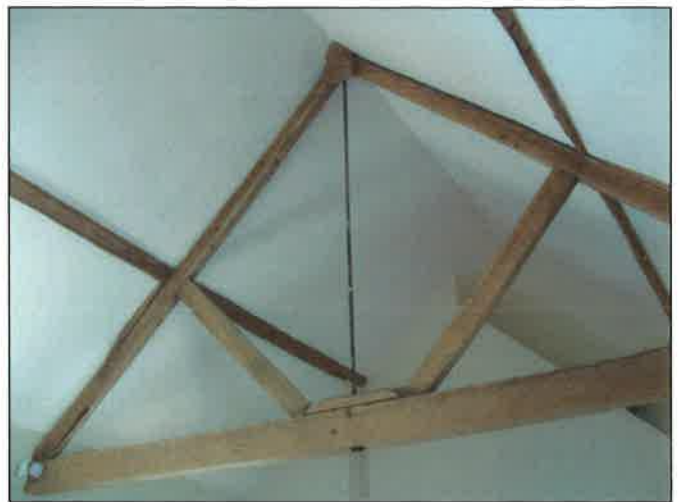
Plate 22: Former barn or stable, roof truss
