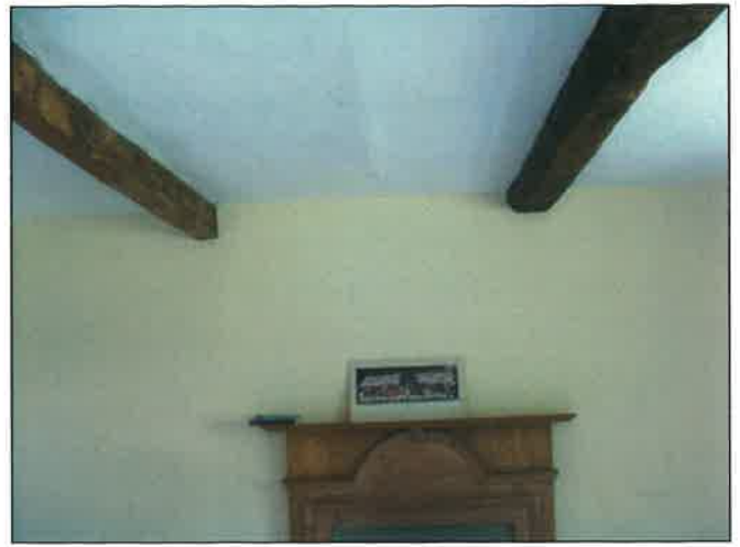
Plate 14: Breakfast room, repositioned and inserted beams
