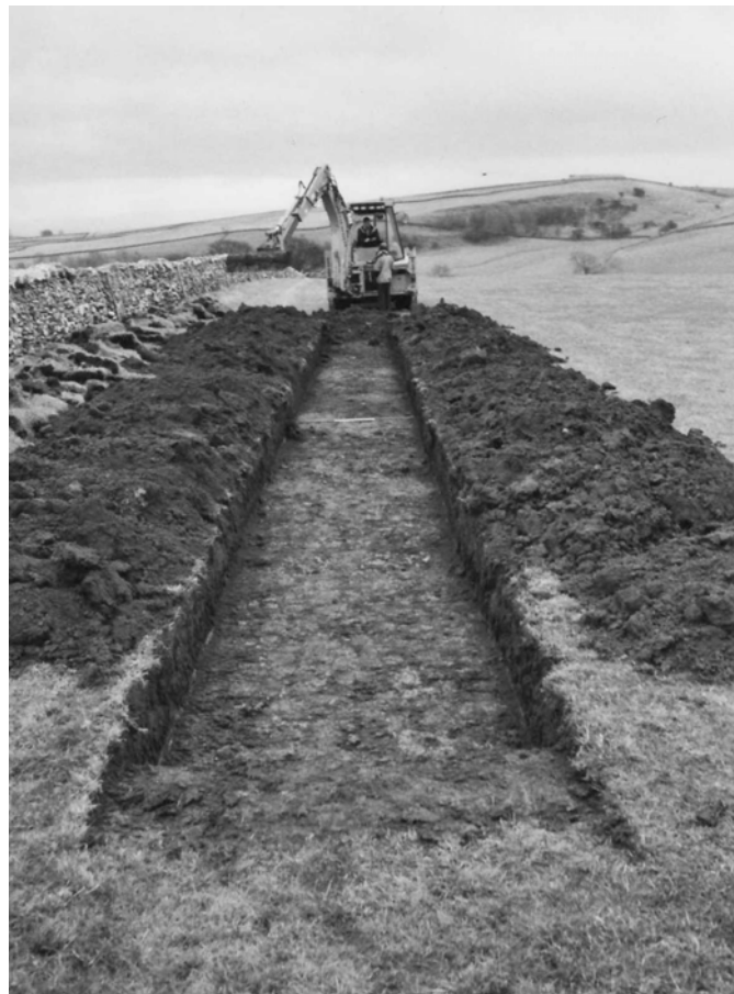
Plate 8: General view of Trench 8, looking east
