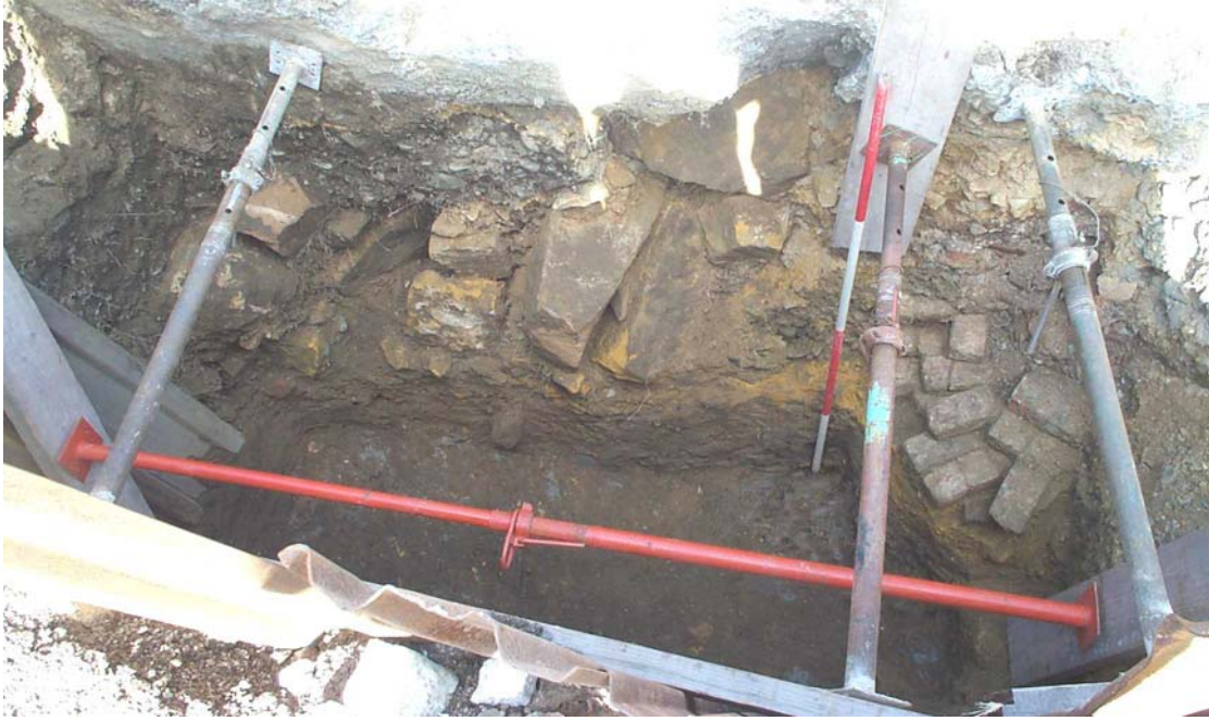
Plate 7: View of wall 1294 looking north
