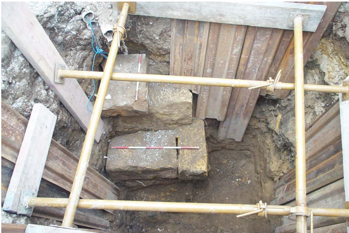
Plate 6: View of wall 1279 looking west
