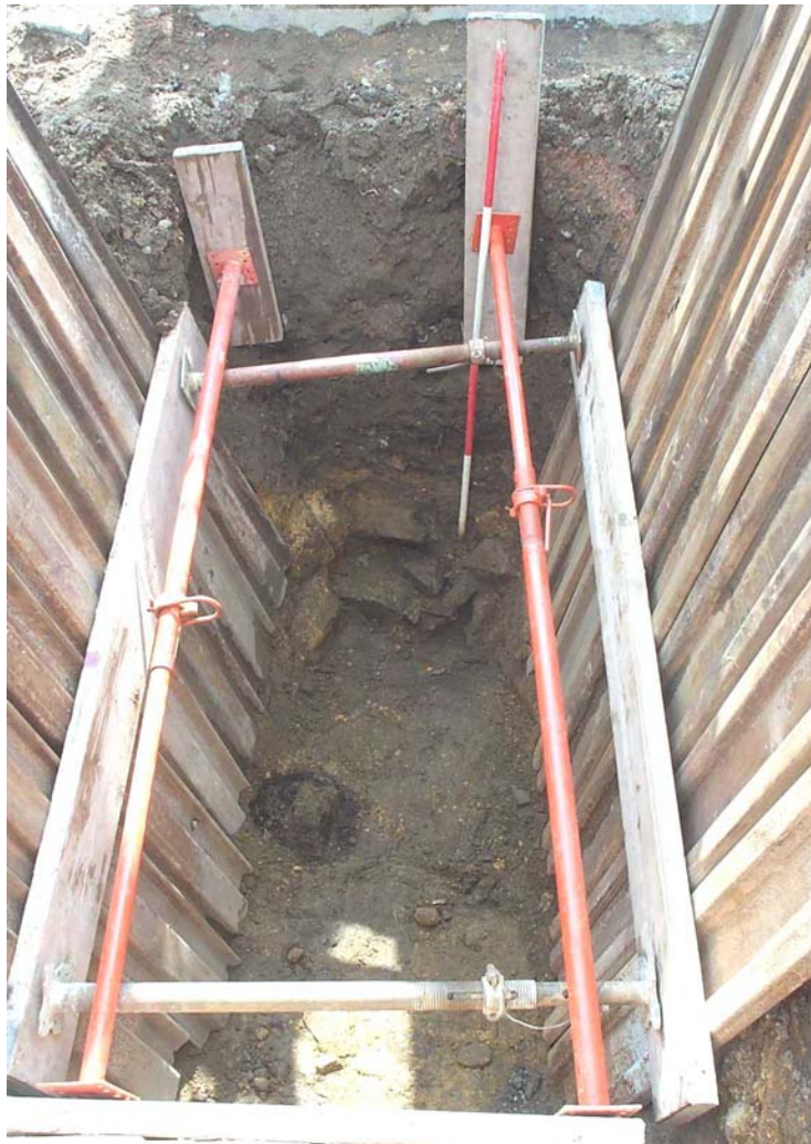
Plate 8: View of timber structure 2314 with east-facing section of wall 2315
