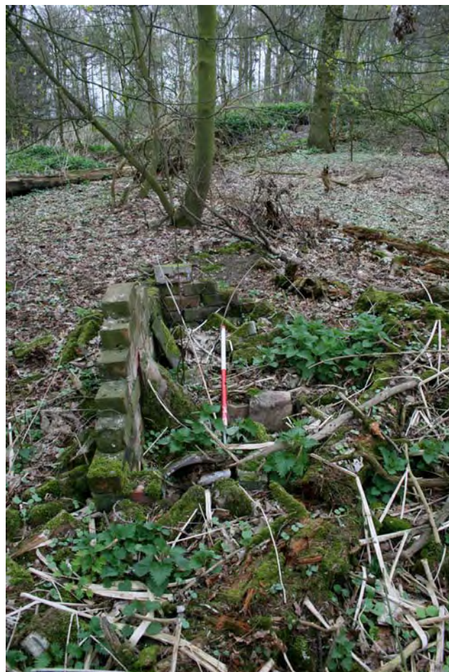
Plate 26: Site 16 , brick structure, looking east-north-east
