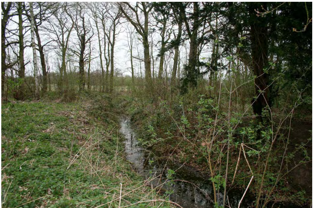
Plate 18: Site 01 , north-west pipe, looking south
