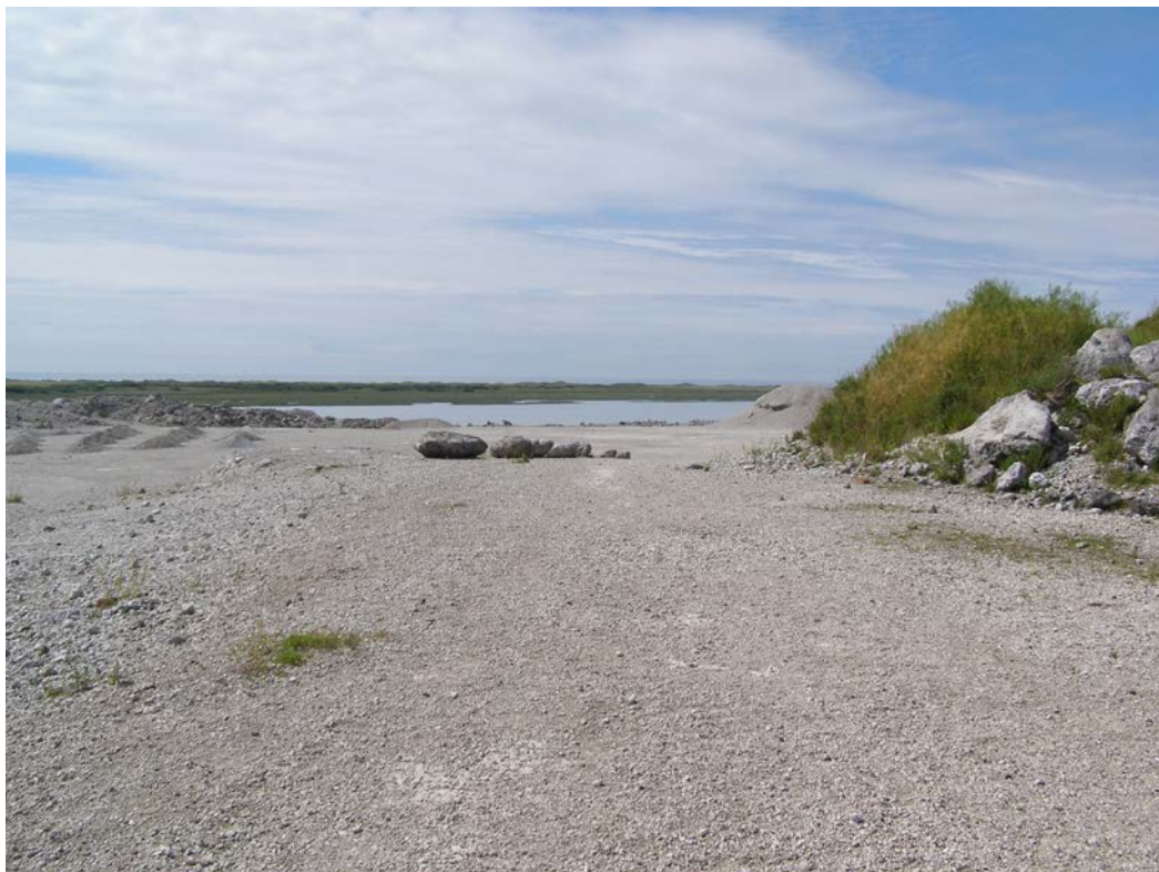
Plate/Shot 46: General view from the current access road onto the slag heap, looking west-south-west
