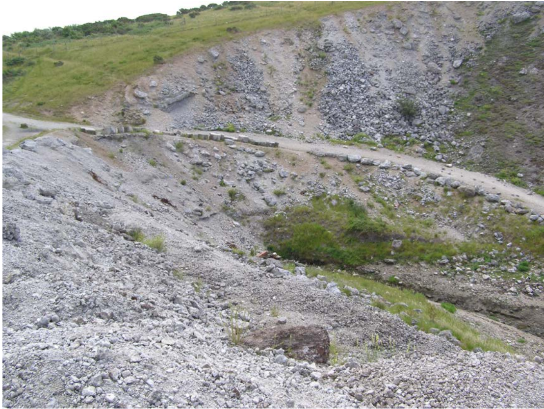
Plate 9: Drainage gully on the south end of the slag heap, looking south-east
