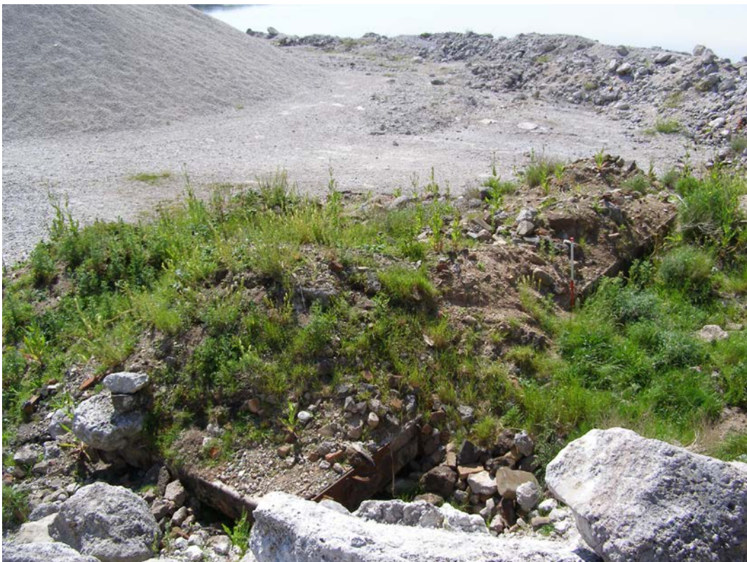
Plate/Shot 44: Detail view of a ruinous wood and metal structure at the north end of site, looking south-west
