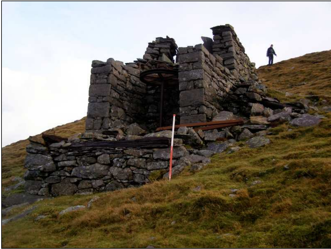
Plate 7: Elidir Fach winder house (NMR 270073)
