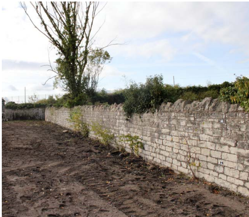
Plate 2: Wall after vegetation clearance.
