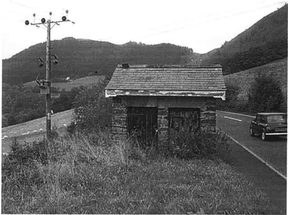
Plate 31 Weigh bridge at Y Bwthyn toll house (Site 601)
