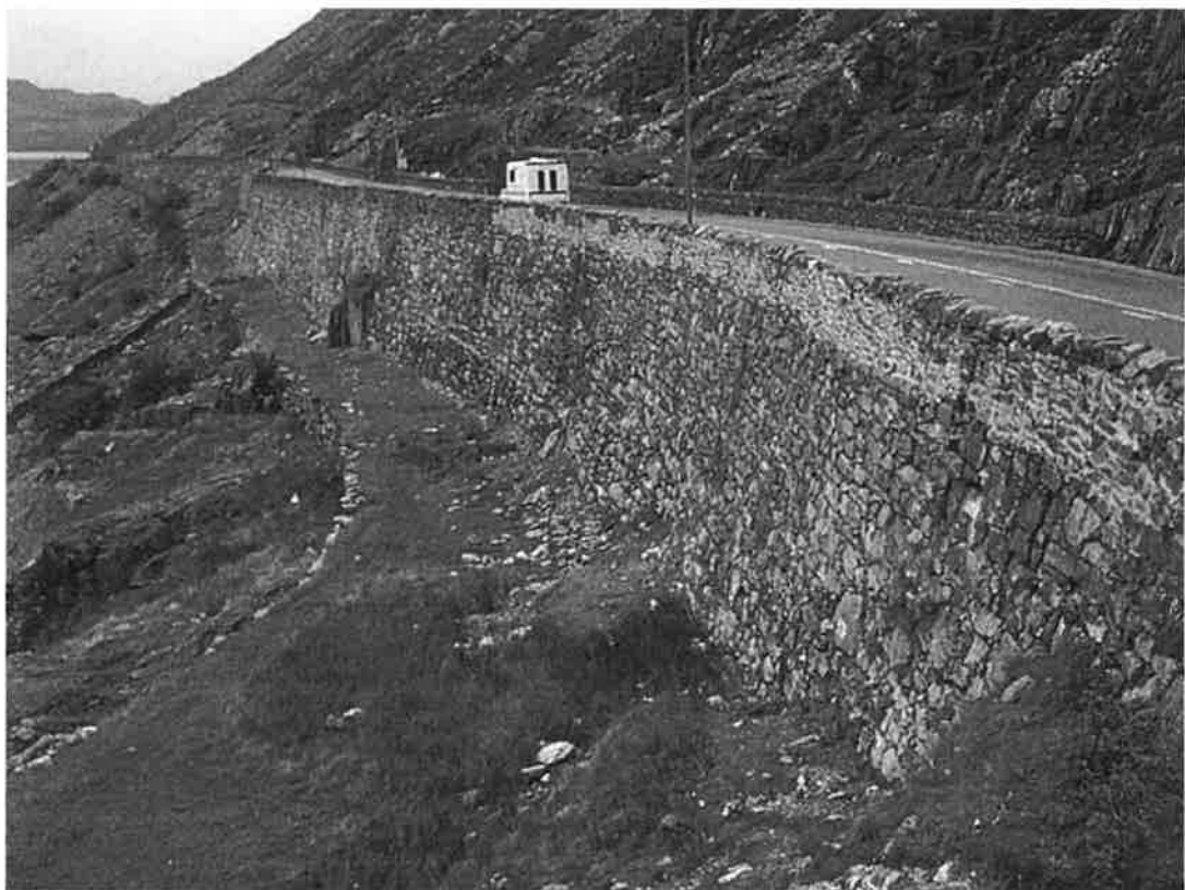
Plate 6 Embankment at Nant Ffrancon and the adjacent earlier turnpike (Site 802)
