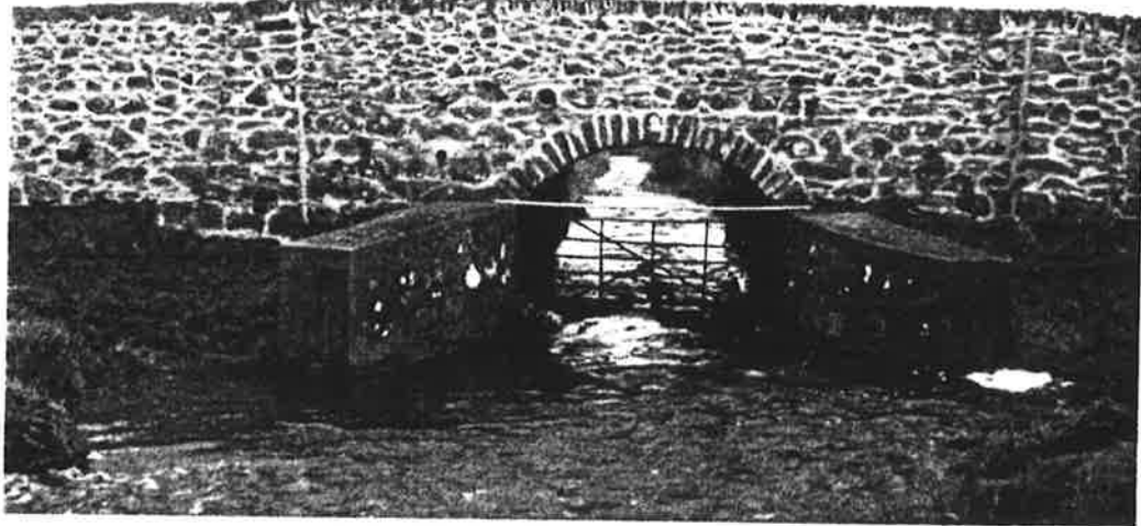
Plate 8 Treban Farm bridge (Site 059)
