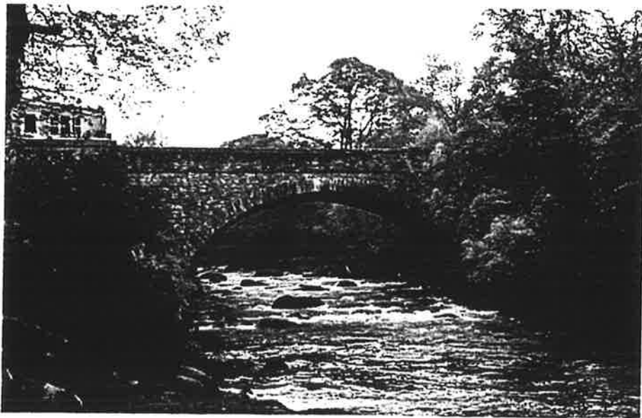
Plate 10 Halfway Bridge (Site 233)
