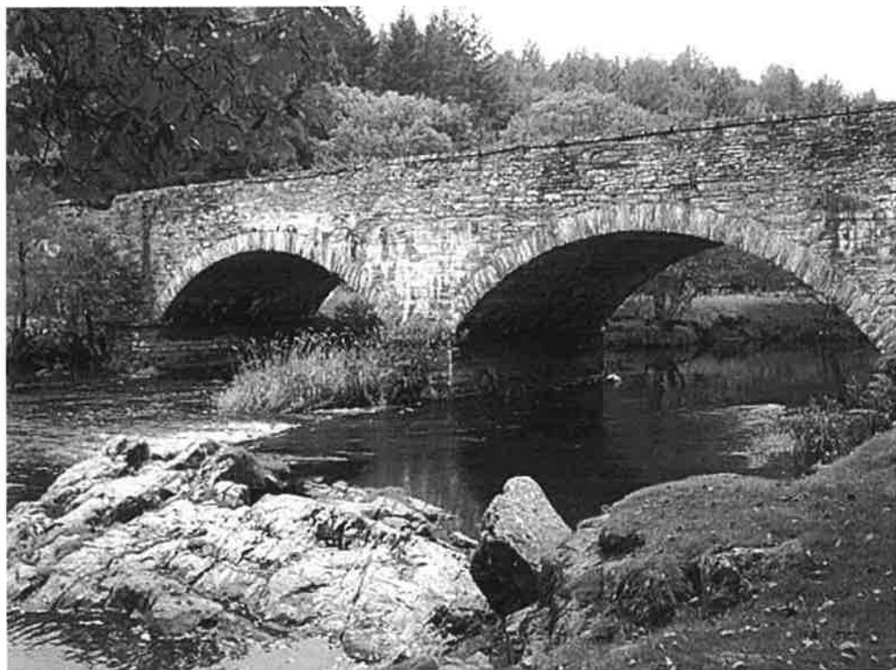
Plate 16 Double arched bridge at Llyngwy (Site 395)
