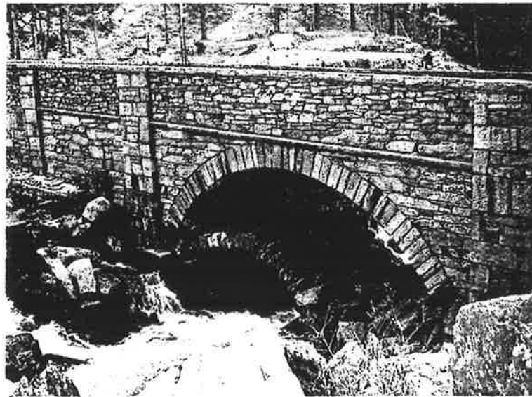
Plate 13 Pont y Benglog bridge in Nant Ffrancon valley (Site 307) from the north- eastern side
