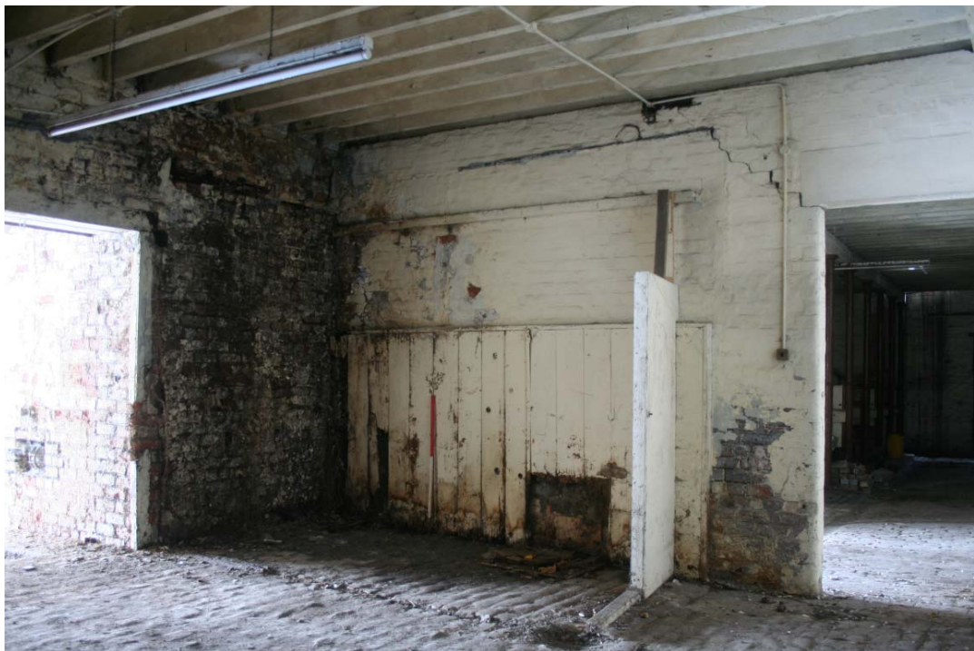
Plate 25: Ante-Room/Tack Room ( 14 ), 71 Smithdown Lane
