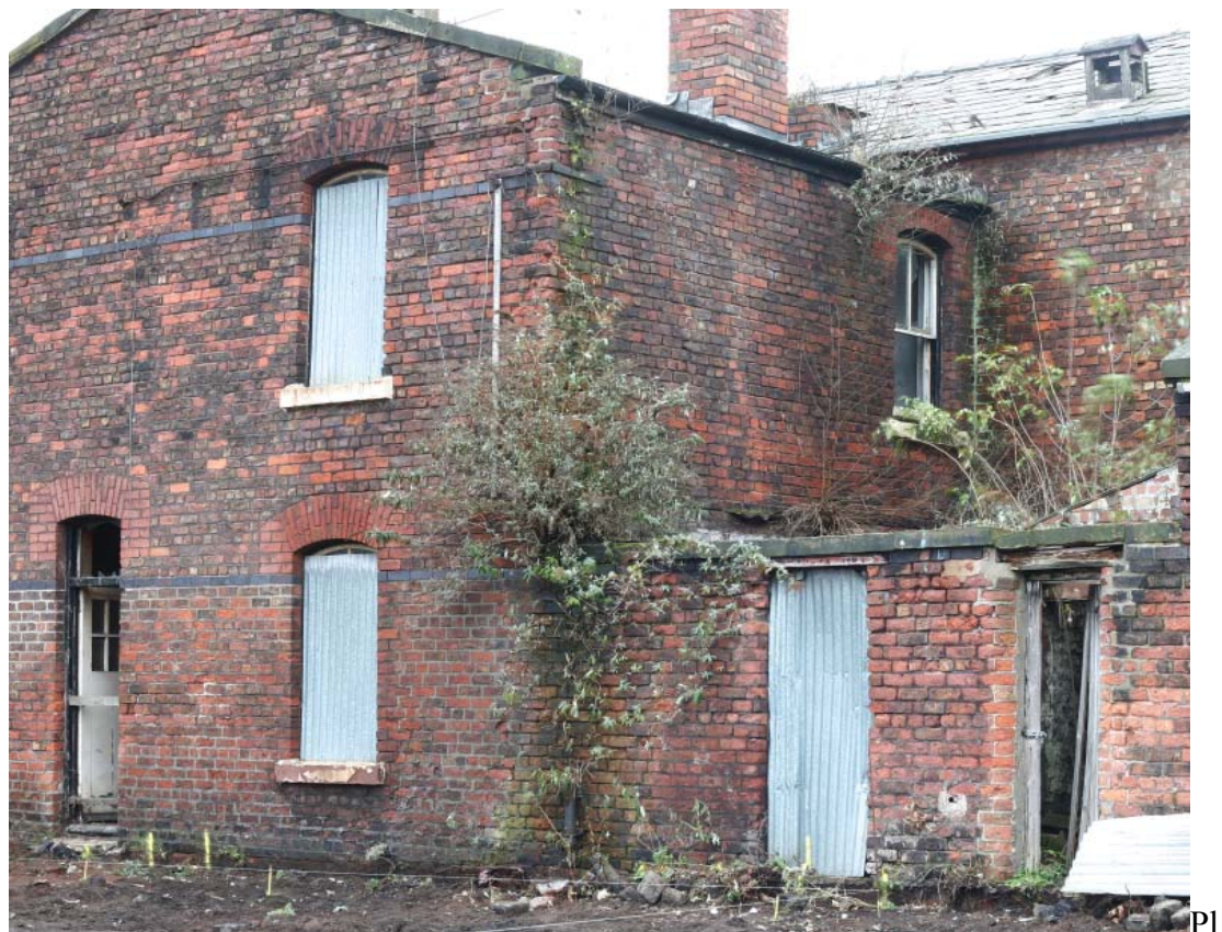
Plate 5: East-facing elevation of 69 Smithdown Lane
