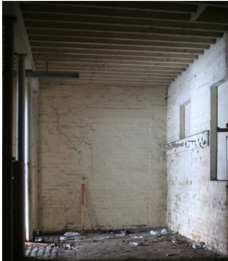
Plate 22: Blocked doorway in western wall of stables ( 11 )
