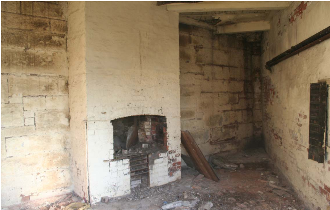
Plate 13: Interior of cook house (5)
