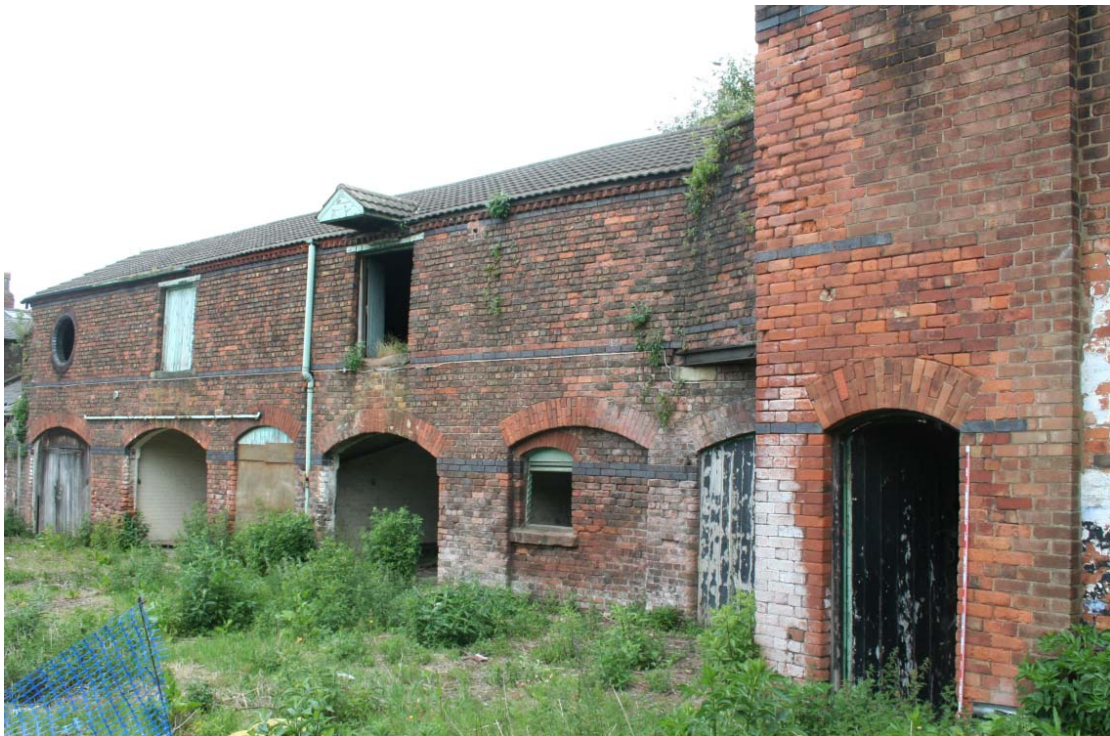
Plate 11: South-facing elevation, 71 Smithdown Lane
