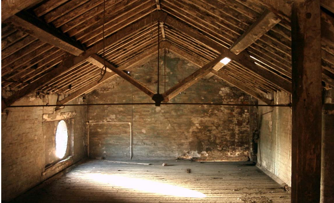
Plate 28: Roof detail within hayloft (Image Courtesy of D Bridston)
