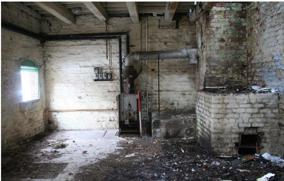
Plate 15: Boiler room (6), 71 Smithdown Lane
