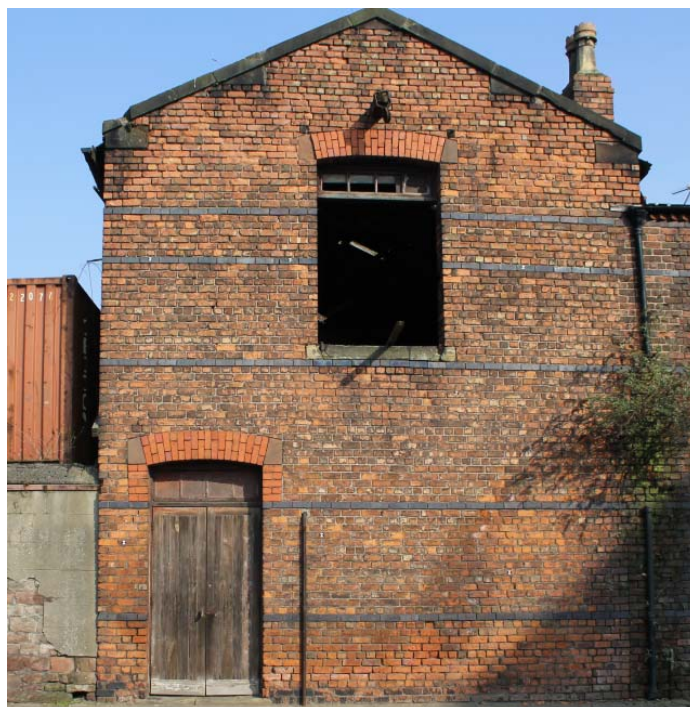
Plate 3: West-facing elevation of stable, 71 Smithdown Lane
