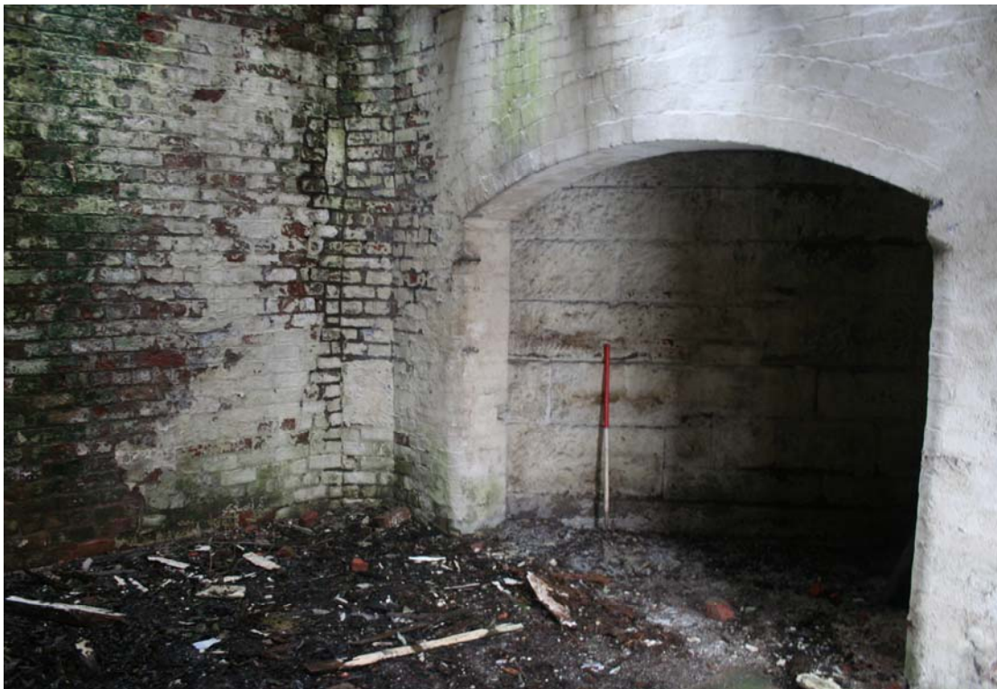
Plate 17: Small ante-room at the east side of boiler room (6)
