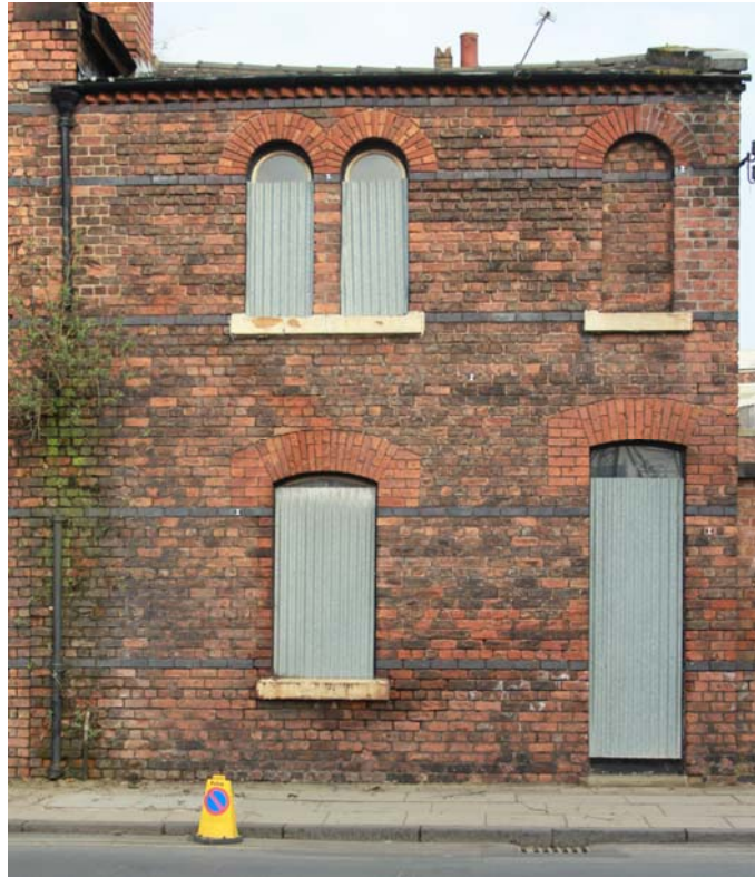
Plate 2: West-facing elevation of two-storey domestic dwelling, 69 Smithdown Lane
