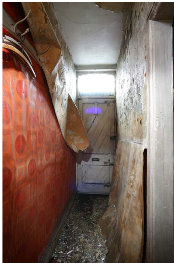
Plate 7: Hallway (2), ground floor 69 Smithdown Lane
