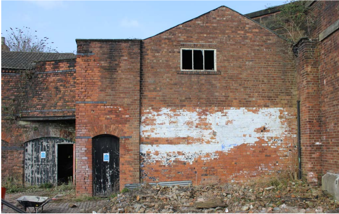
Plate 12: Exterior of cook house (5), 71 Smithdown Lane
