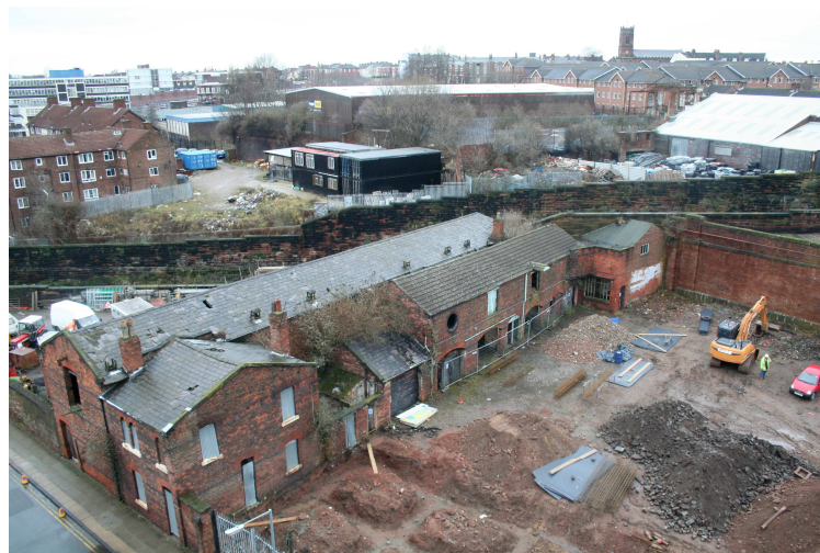
Plate 1: Aerial view showing south- and west-facing elevations of the surviving north block of Smithdown Lane Corporation Stable Yard
