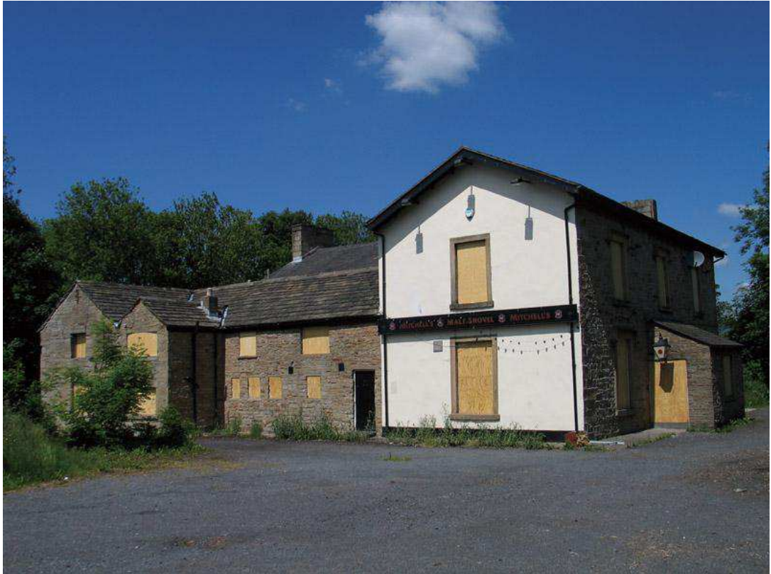
Plate 2: The Malt Shovel Public House (Site 03) prior to being converted into apartments
