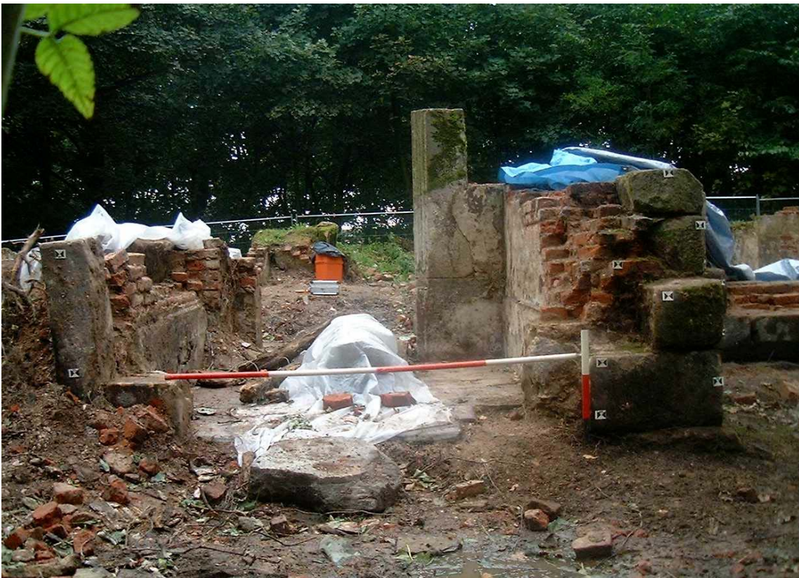
Plate 8 View of the porch, looking west, at the outset of consolidation
