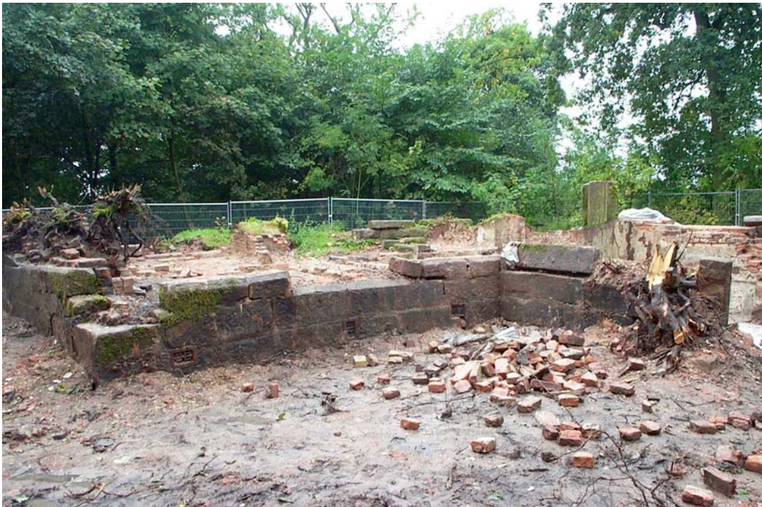
Plate 10: Southern part of Clayton Hall, including the porch, viewed from the south-east at the outset of the consolidation
