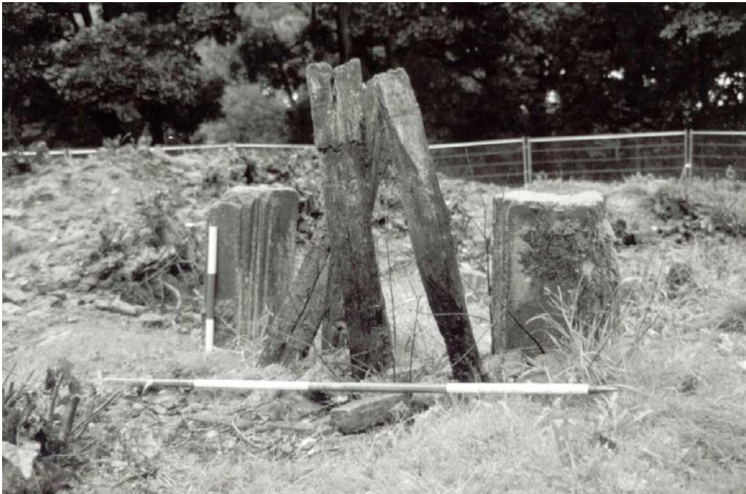
Plate 6: Main eastern entrance prior to clearance excavation, looking west
