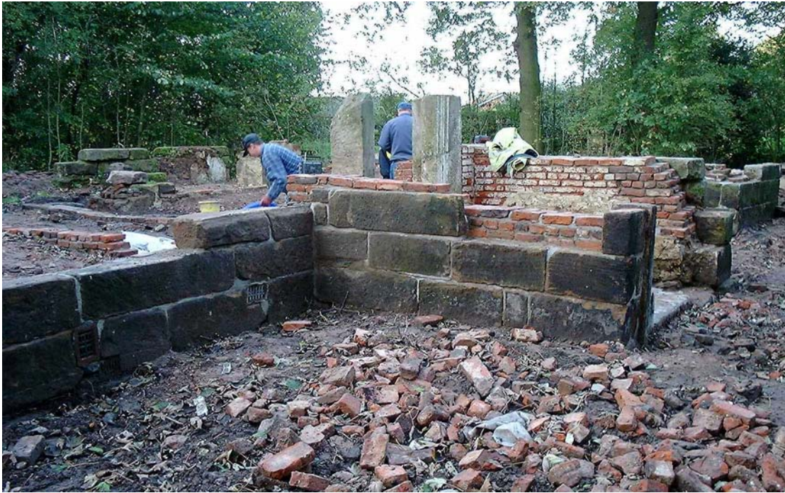
Plate 9: The porch following consolidation, viewed from the south-east
