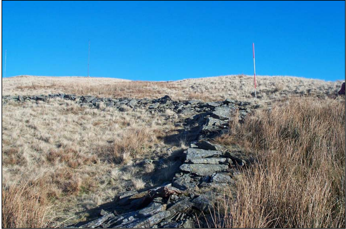
Plate 1: Borrowdale Edge, boundary wall (Site 33), facing north-east.
