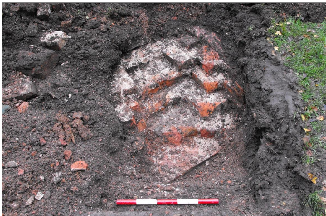
Plate 6: Wall footings in tunnelling pit CP7B
