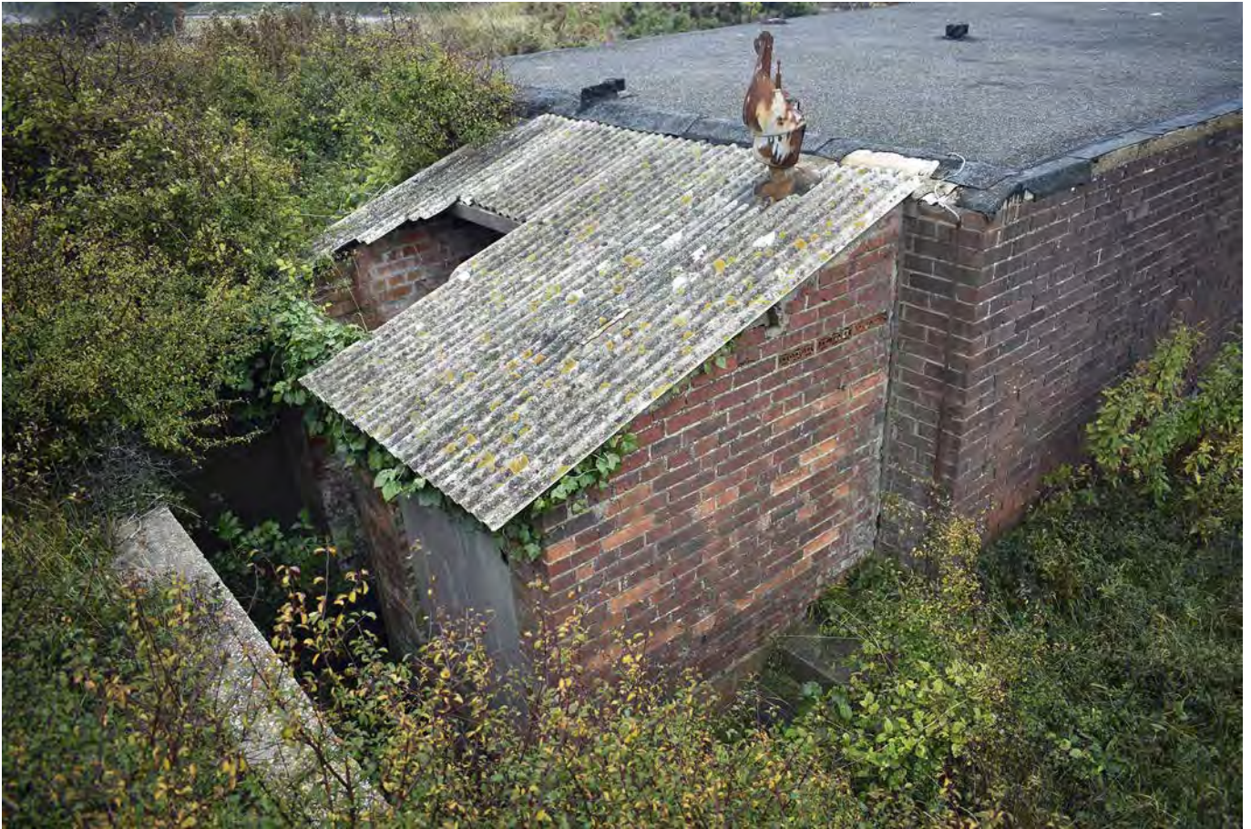
Plate 47: Radar building, external view of north end
