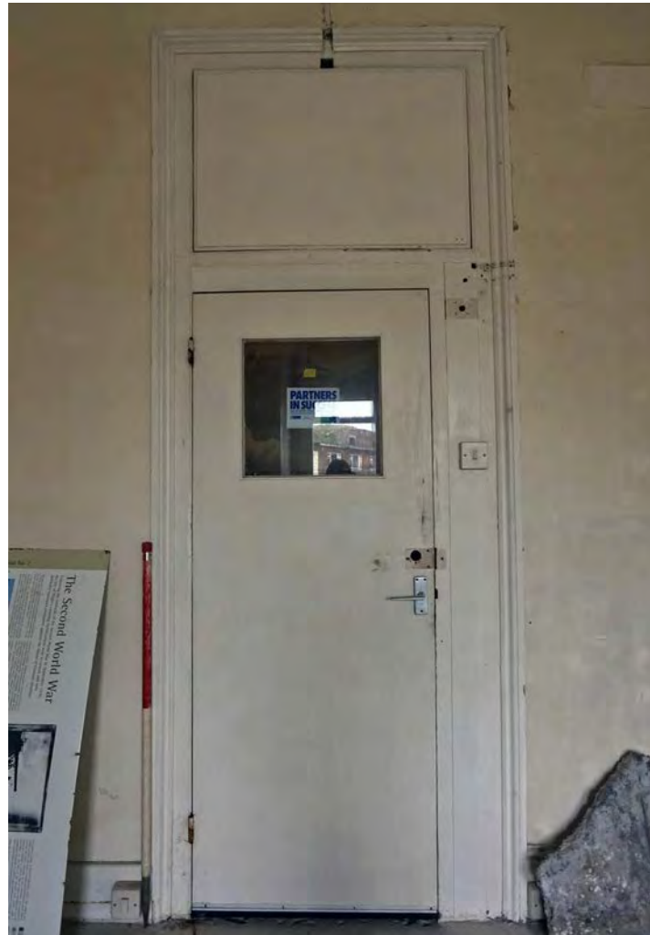
Plate 40: Bay G, door on east wall to connecting corridor
