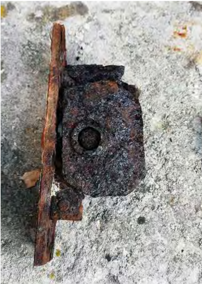
Plate 12: Cast-iron axle-pulley removed from window (A2), dating from the 1862-67
