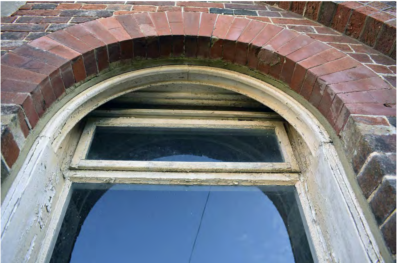
Plate 38: Bay G, external view of opening G19
