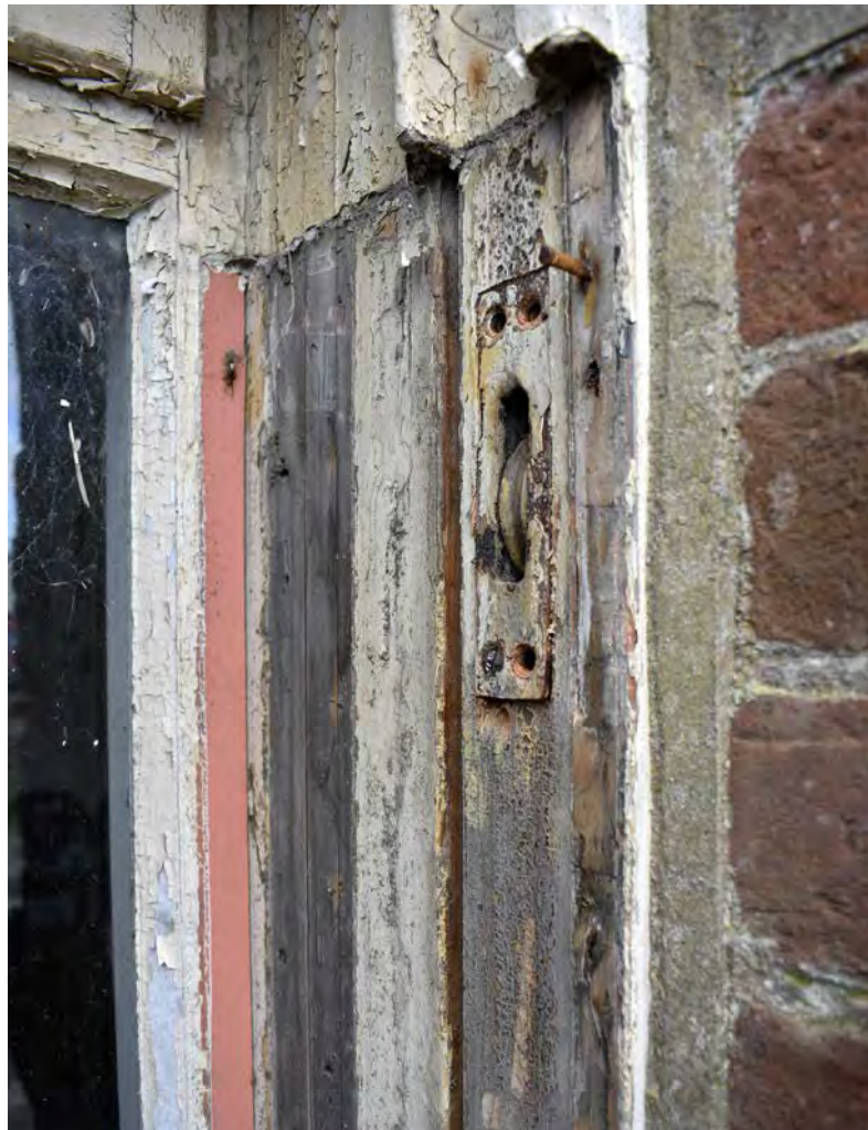
Plate 42: Bay H, external view of opening H20 with panel removed
