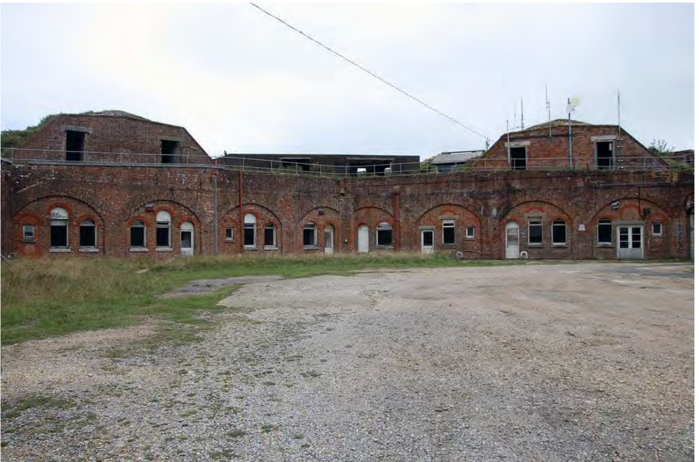
Plate 4: East facing view of Officer's Quarters
