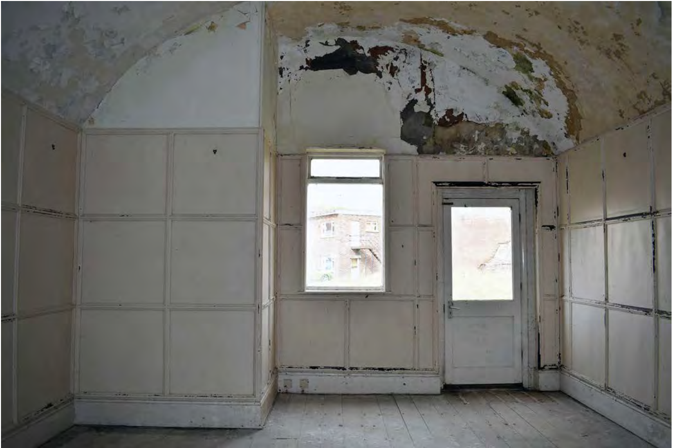
Plate 35: Bay F, internal view
