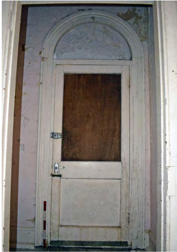
Plate 29: Bay D, internal view of opening D11
