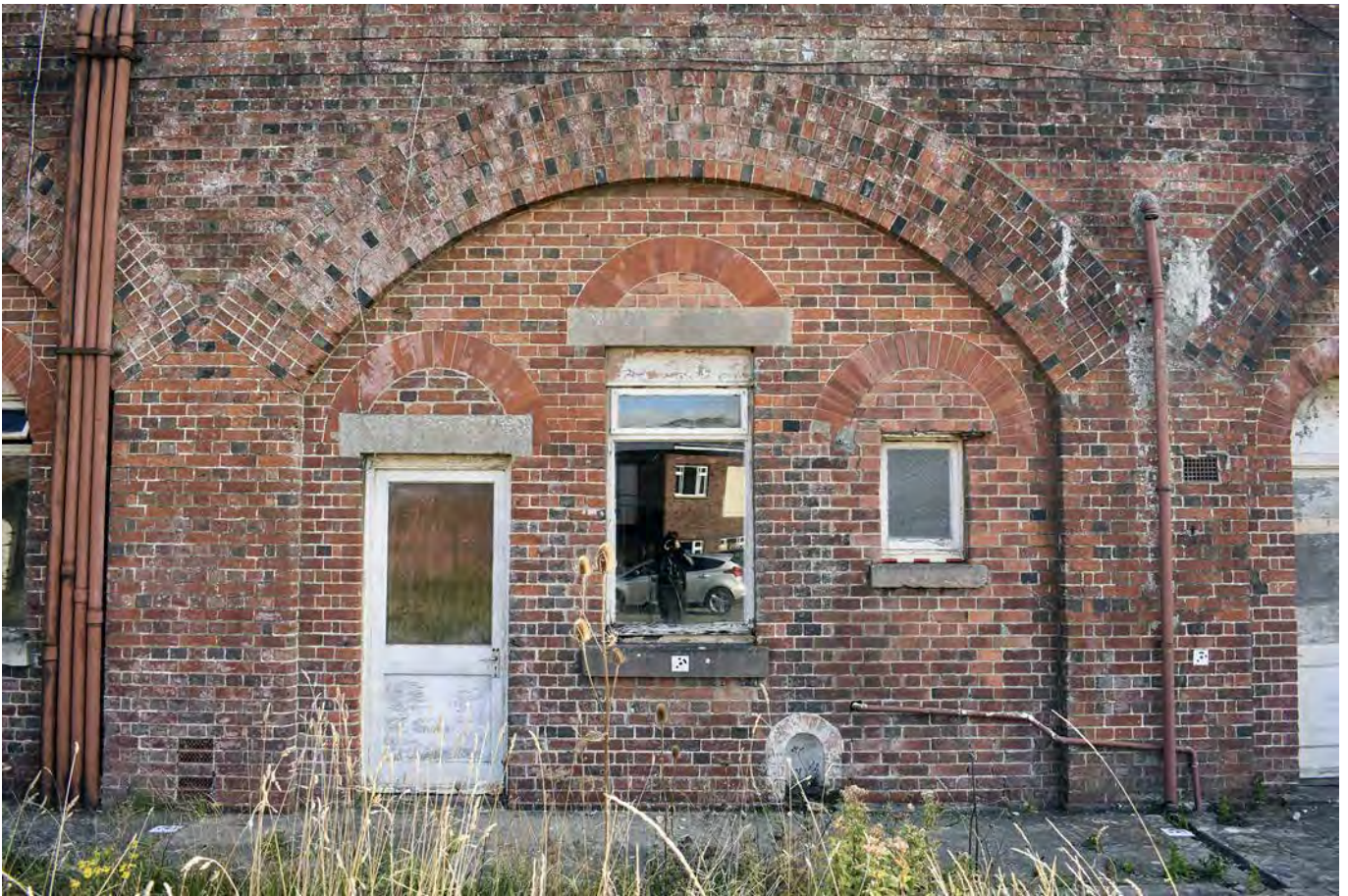
Plate 33: Bay F, external view
