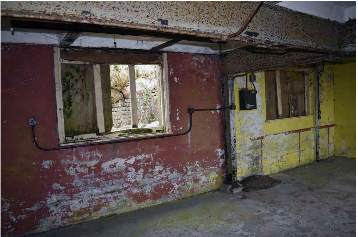
Plate 46: Radar building, internal view showing re-used sash window and roof support
