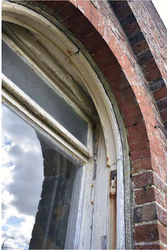
Plate 11: Bay C, opening C9, showing inferior type of sash window
