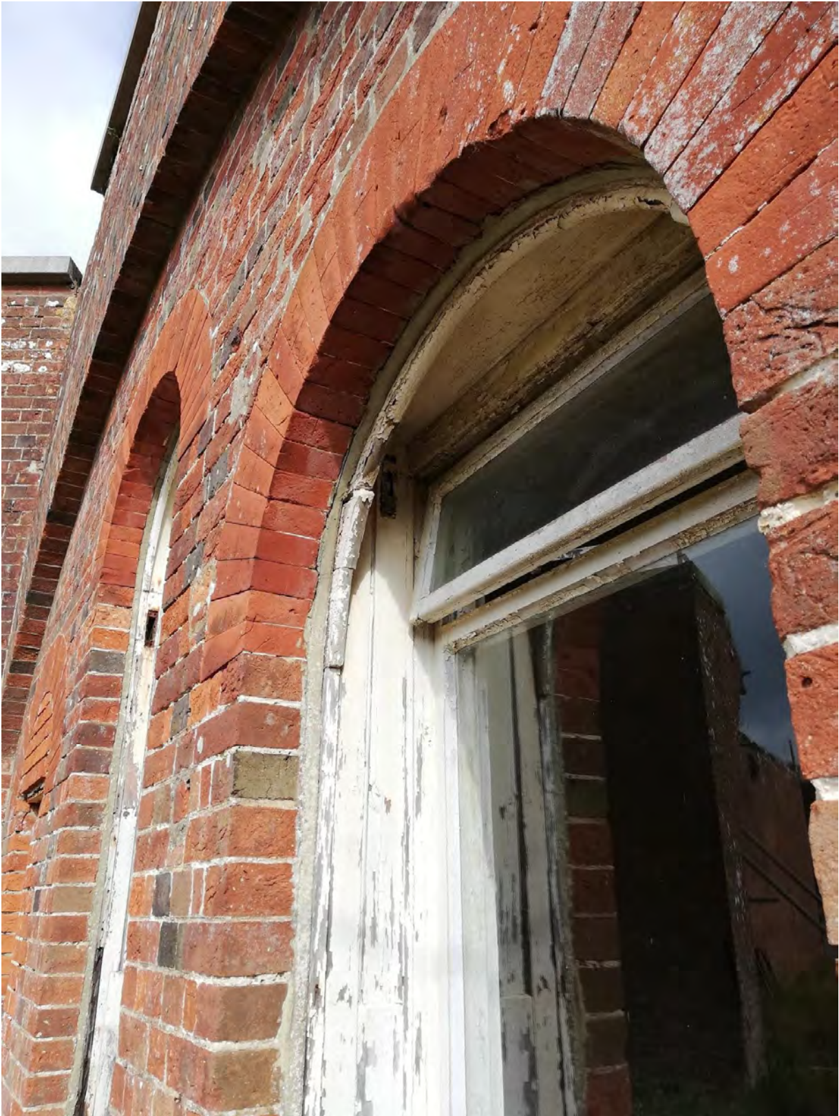
View of window (A3) with cheaper (more common) arched head construction.
