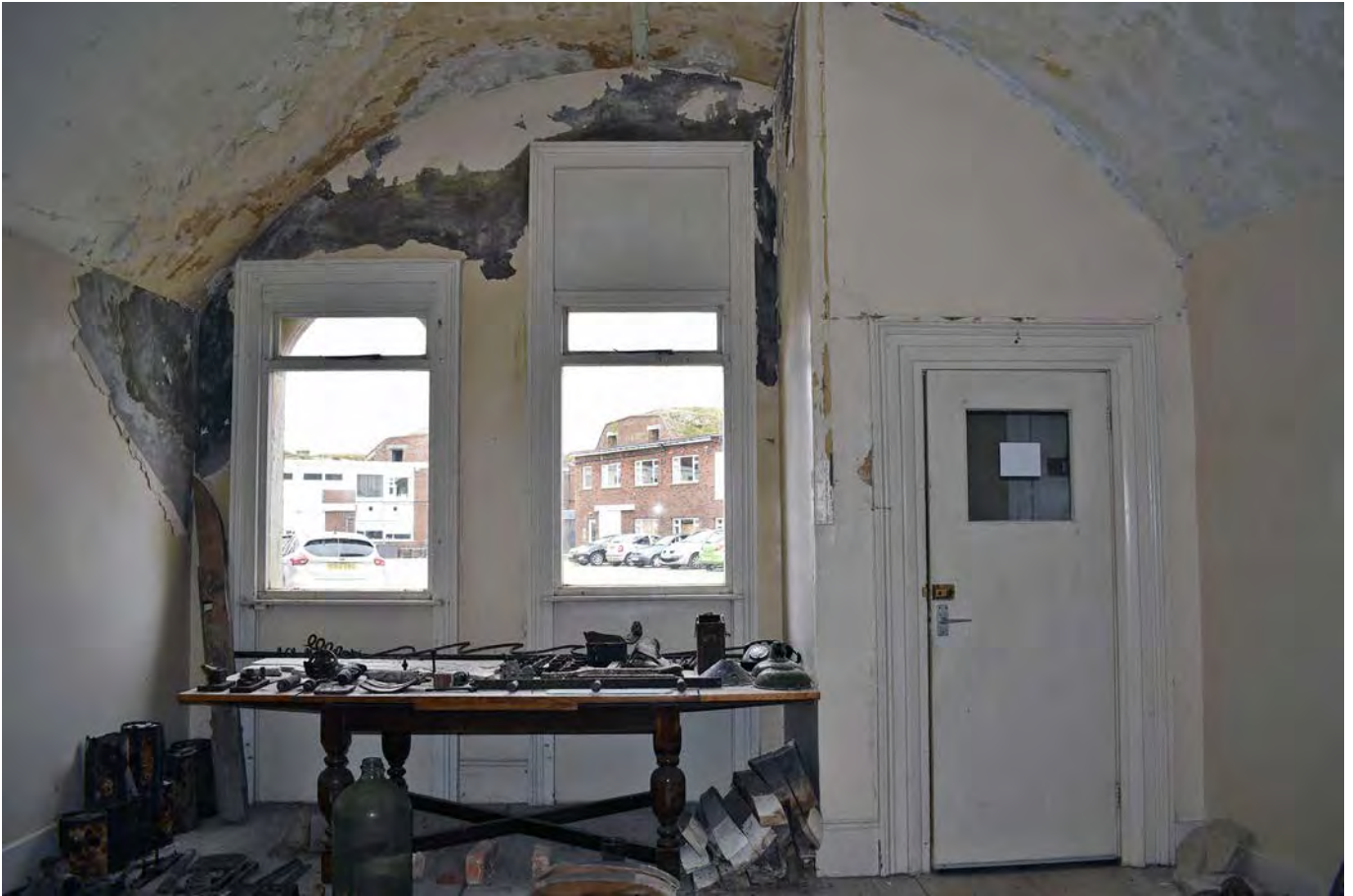
Plate 39: Bay G, internal view
