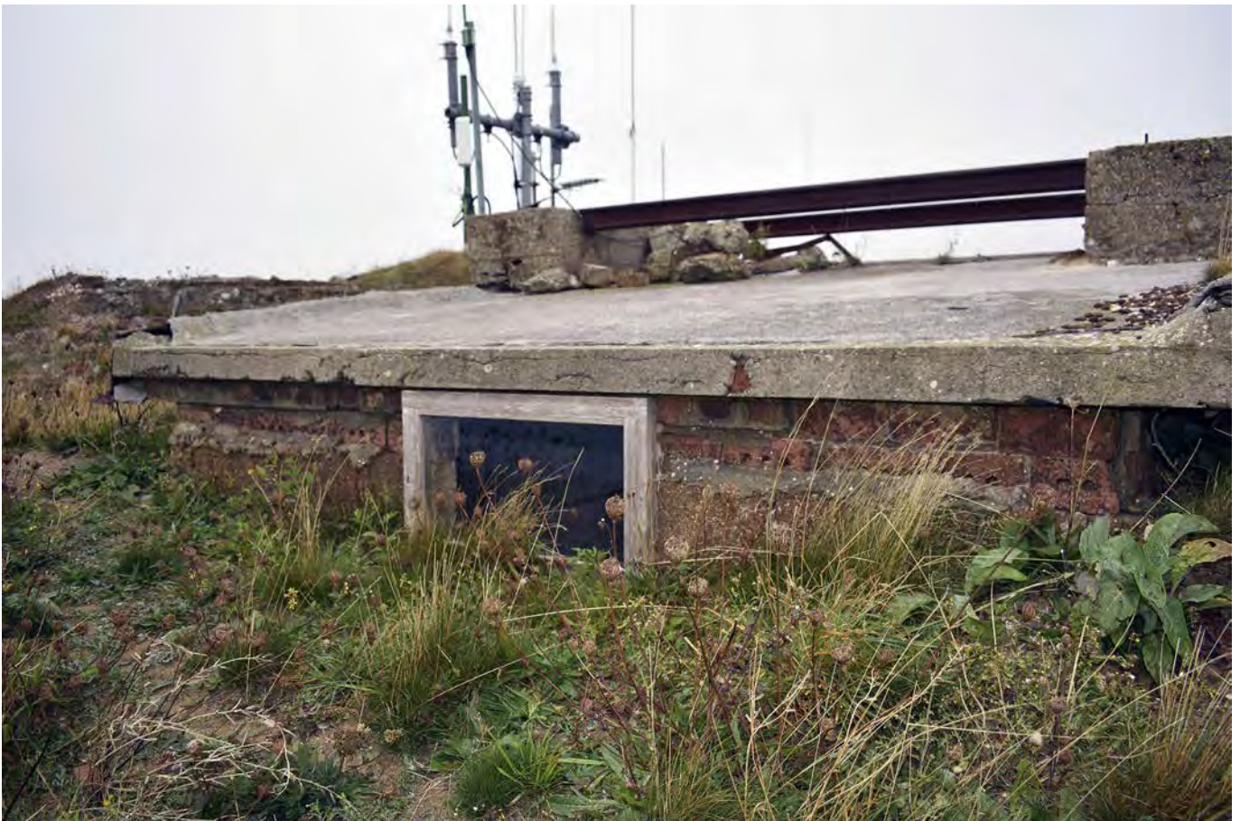
Plate 54: Position Finding Cell, external view of rear elevation and roof
