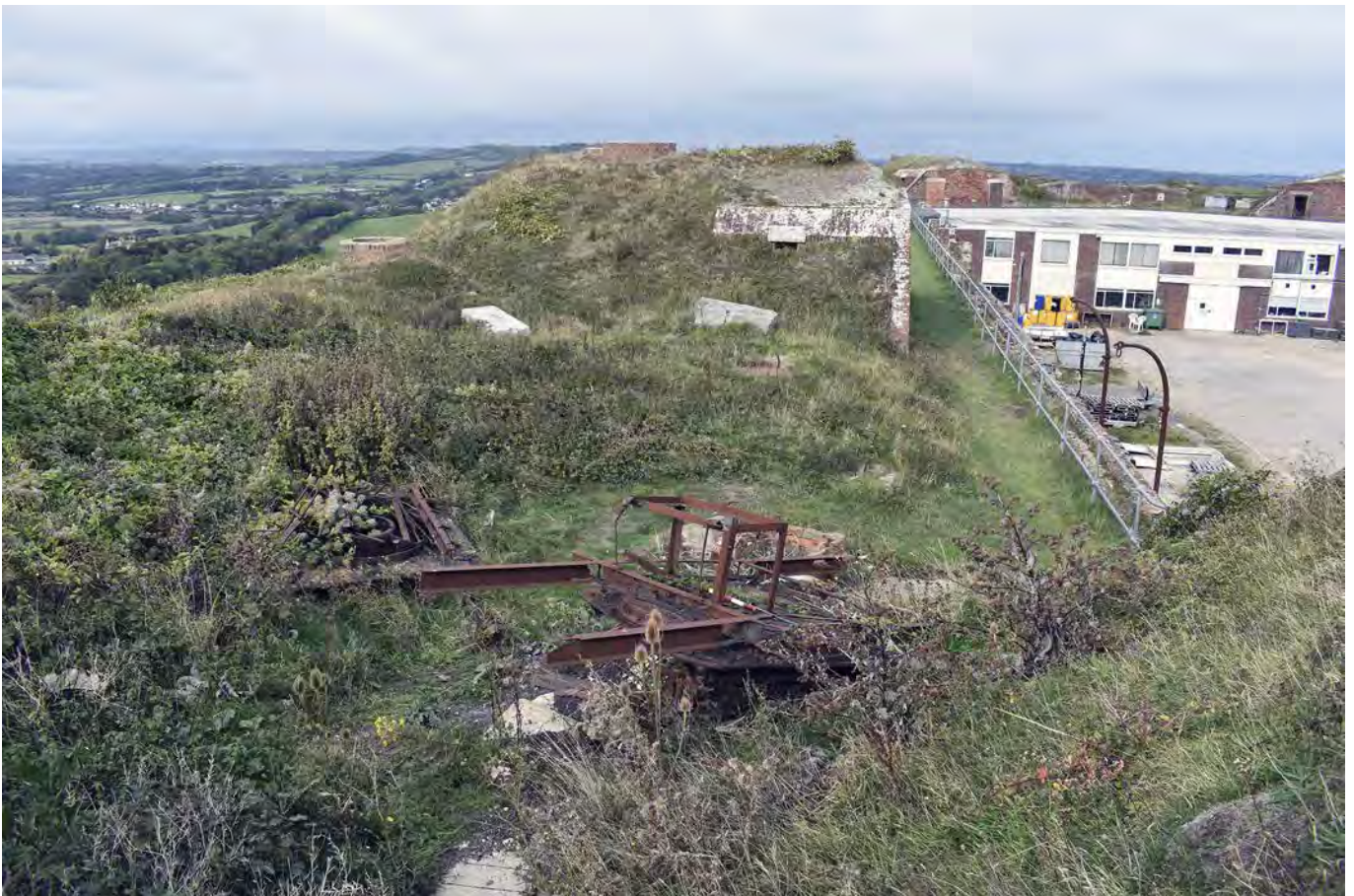
Plate 50: Remains of both radar supports
