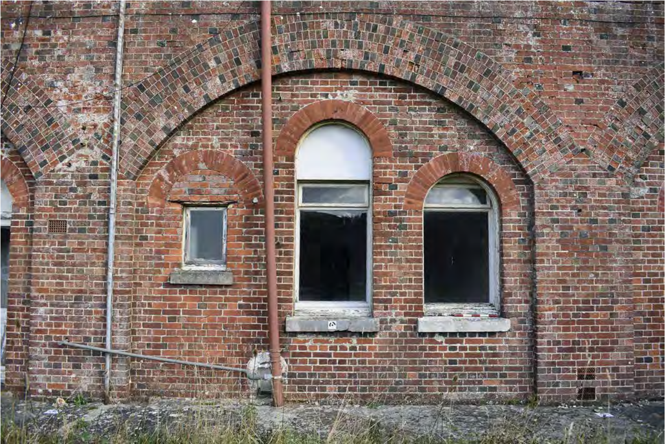
Plate 24: Bay C, external view
