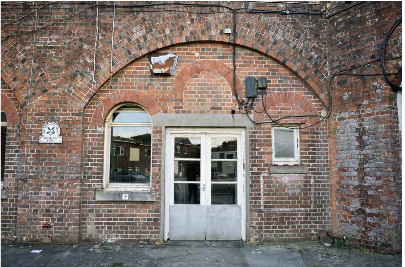
Plate 6: Bay H, showing later infill and insertion of door
