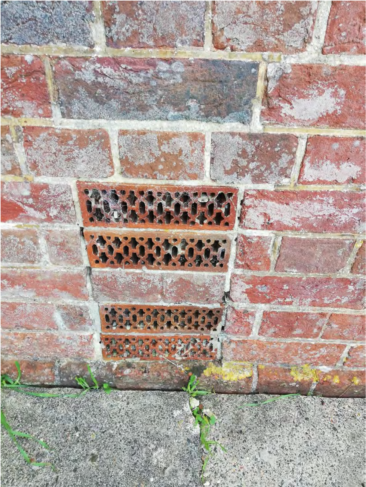
Detail of original air-bricks, typical of ornamental mid-Victorian designs.
