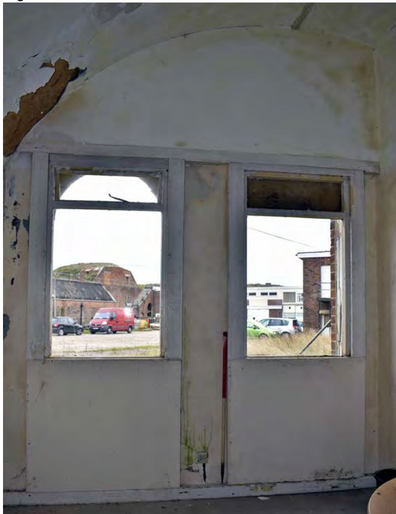
Plate 19: Bay A, internal view of openings A2 and A3
