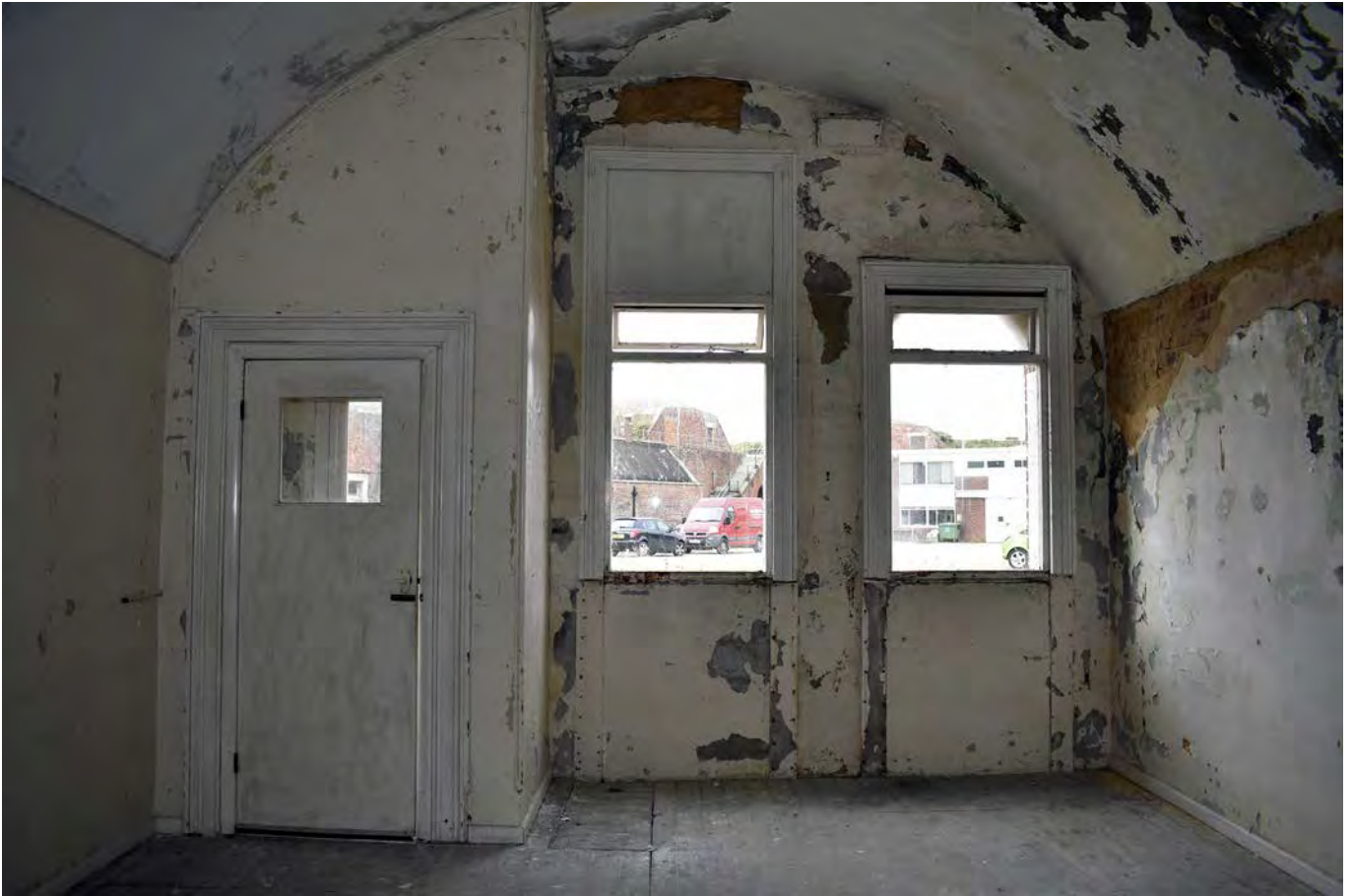
Plate 22: Bay B, internal view
