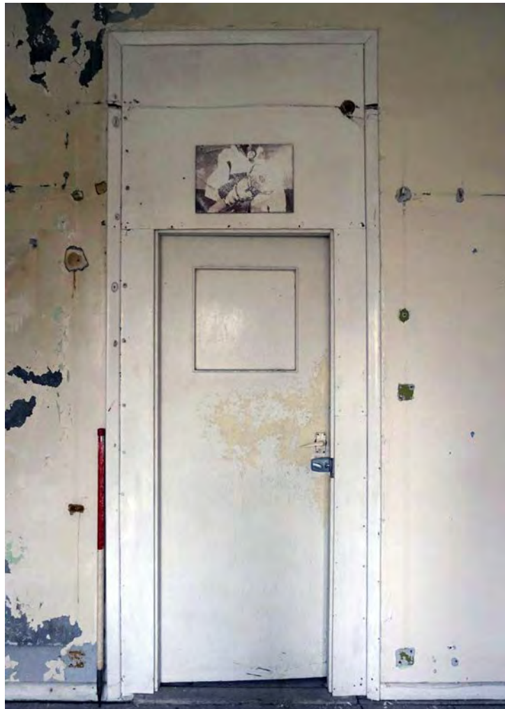
Plate 23: Bay B, internal door on east wall leading to connecting corridor
