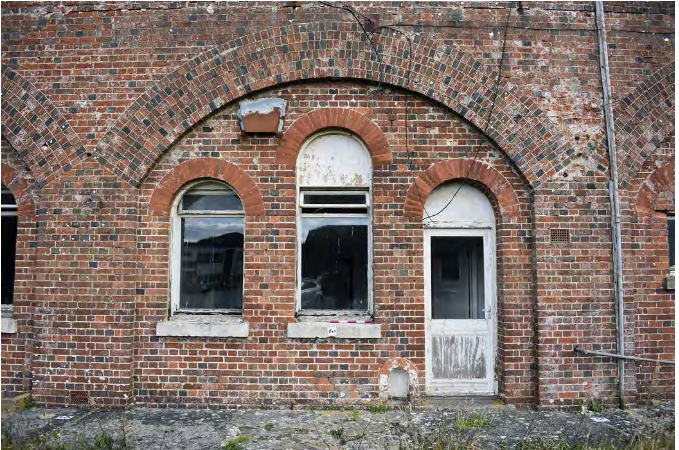
Plate 5: Bay B, showing original construction
