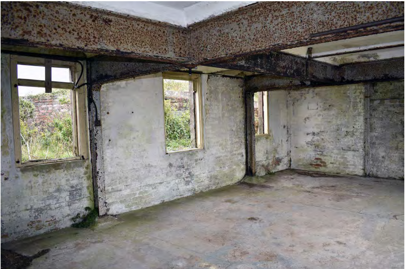
Plate 48: Radar building, internal view of south end
