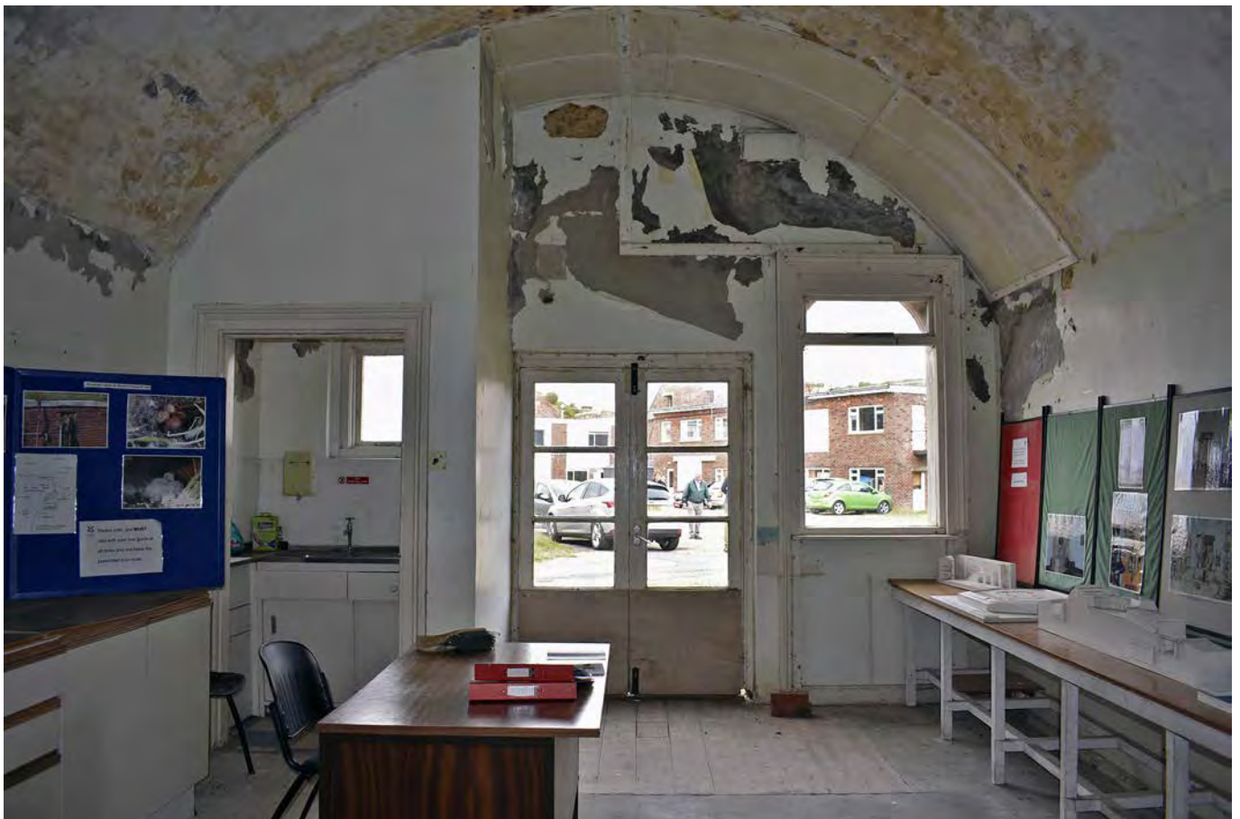
Plate 44: Bay H, internal view
