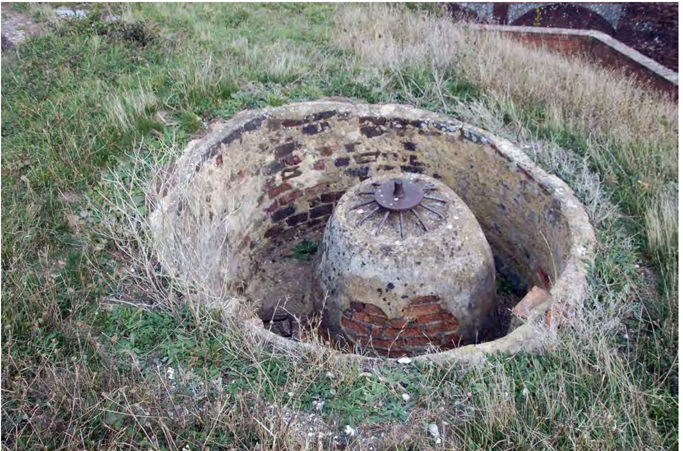
Plate 60: Spigot Mortar emplacement (east)
