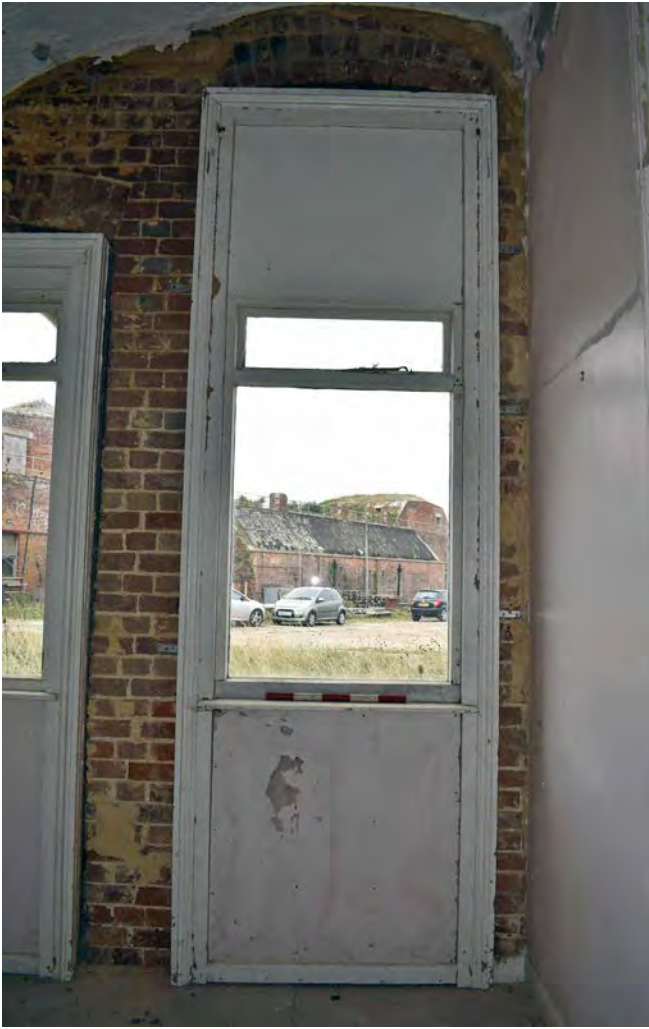
Plate 26: Bay C, internal view of sash frames
