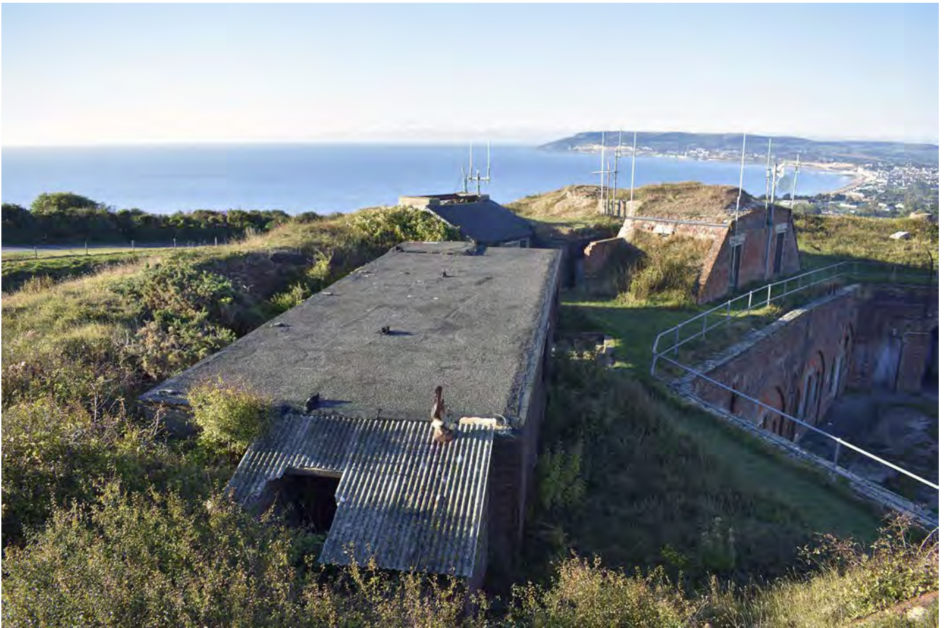
Plate 49: Radar building, roof, looking south
