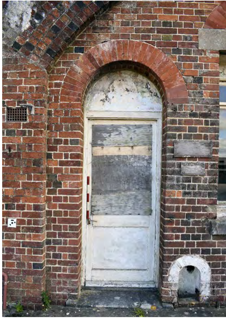
Plate 37: Bay G, external view of opening G17
