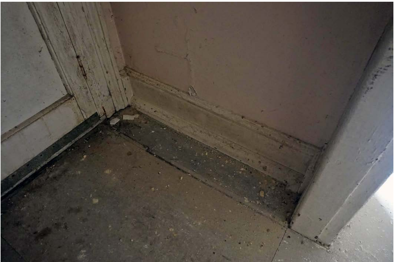
Plate 30: Bay D, skirting board
