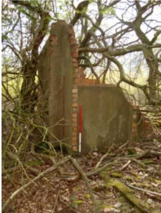
Plate 27: West end of brick structure, Site 103 , looking east
