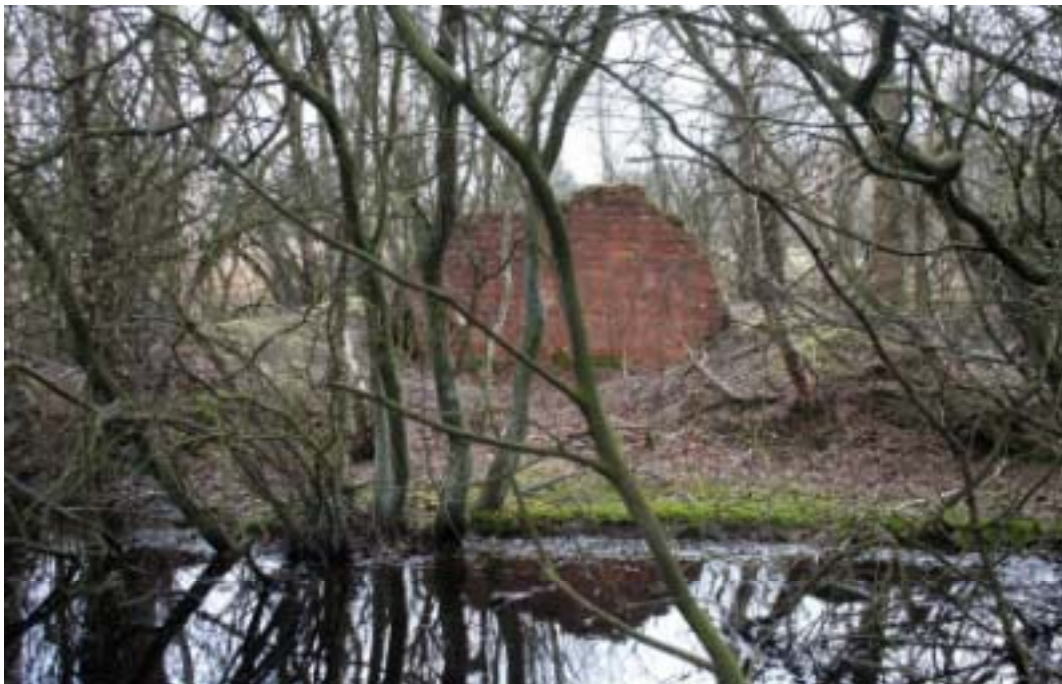
Plate 26: 'Component Store', Site 84 , looking south
