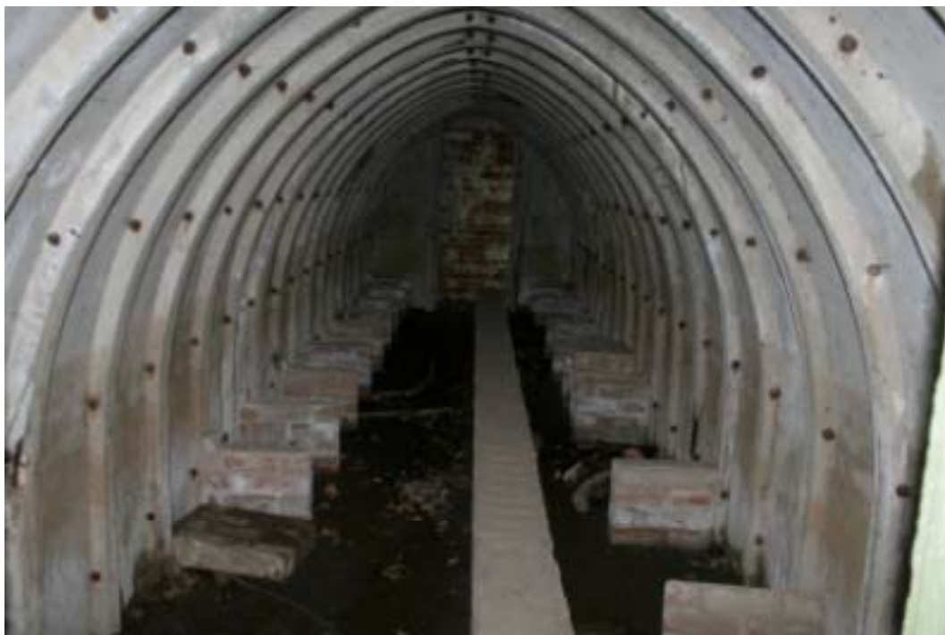
Plate 18: Interior of air raid shelter, Site 49
