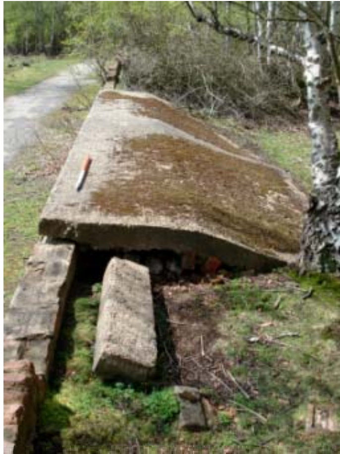
Plate 25: Concrete ramp of bomb store, Site 25 , looking west
