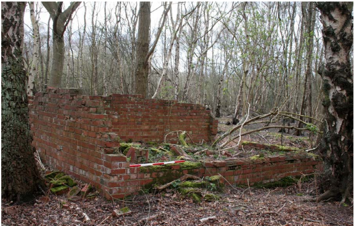
Plate 20: Brick built structure, Site 44 , looking west
