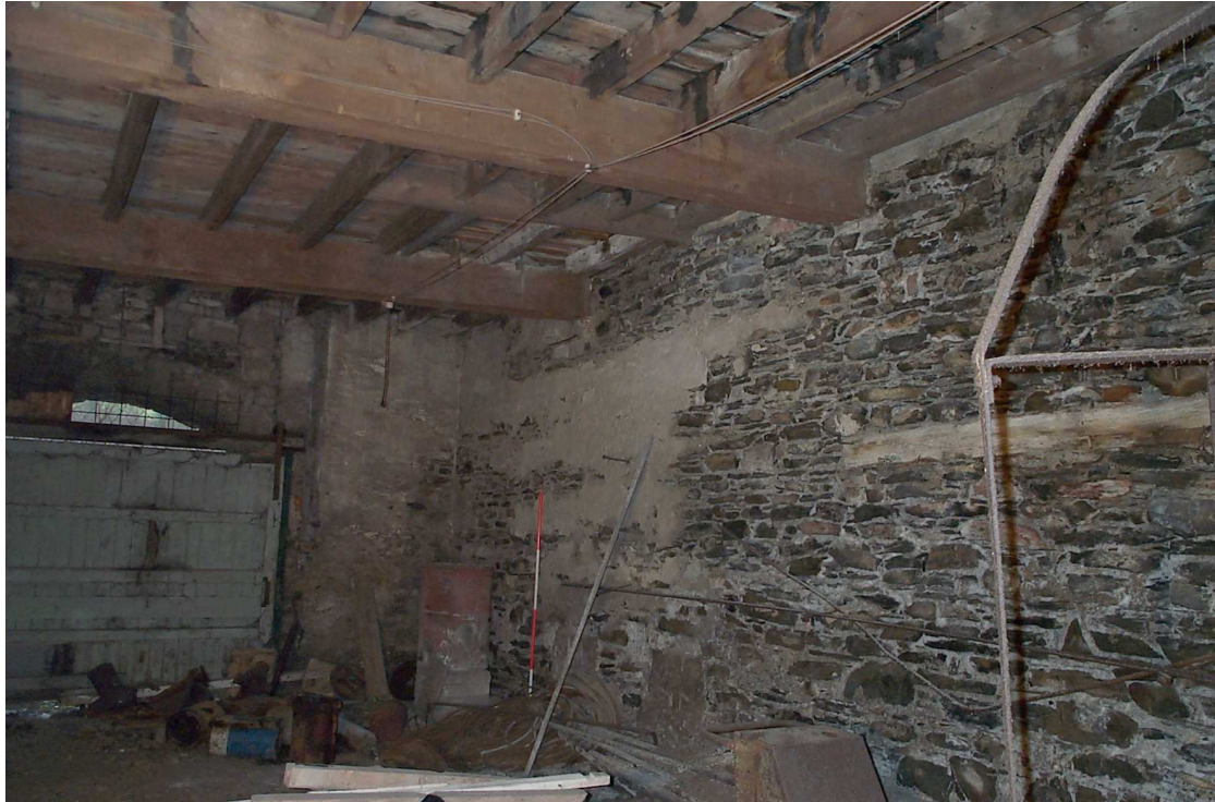
Plate 2: Ground floor room 1 (GF1) showing the western wall
