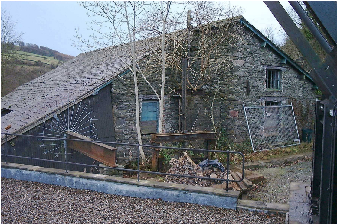
Plate 7: North facing elevation
