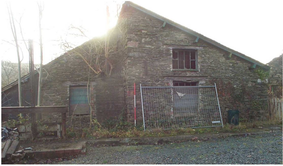
Plate 9 North facing elevation
