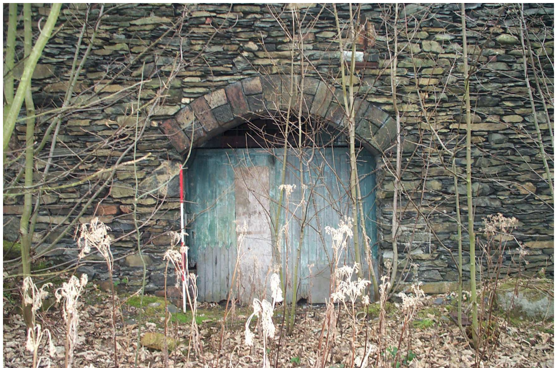
Plate 8 South facing entrance to the mill
