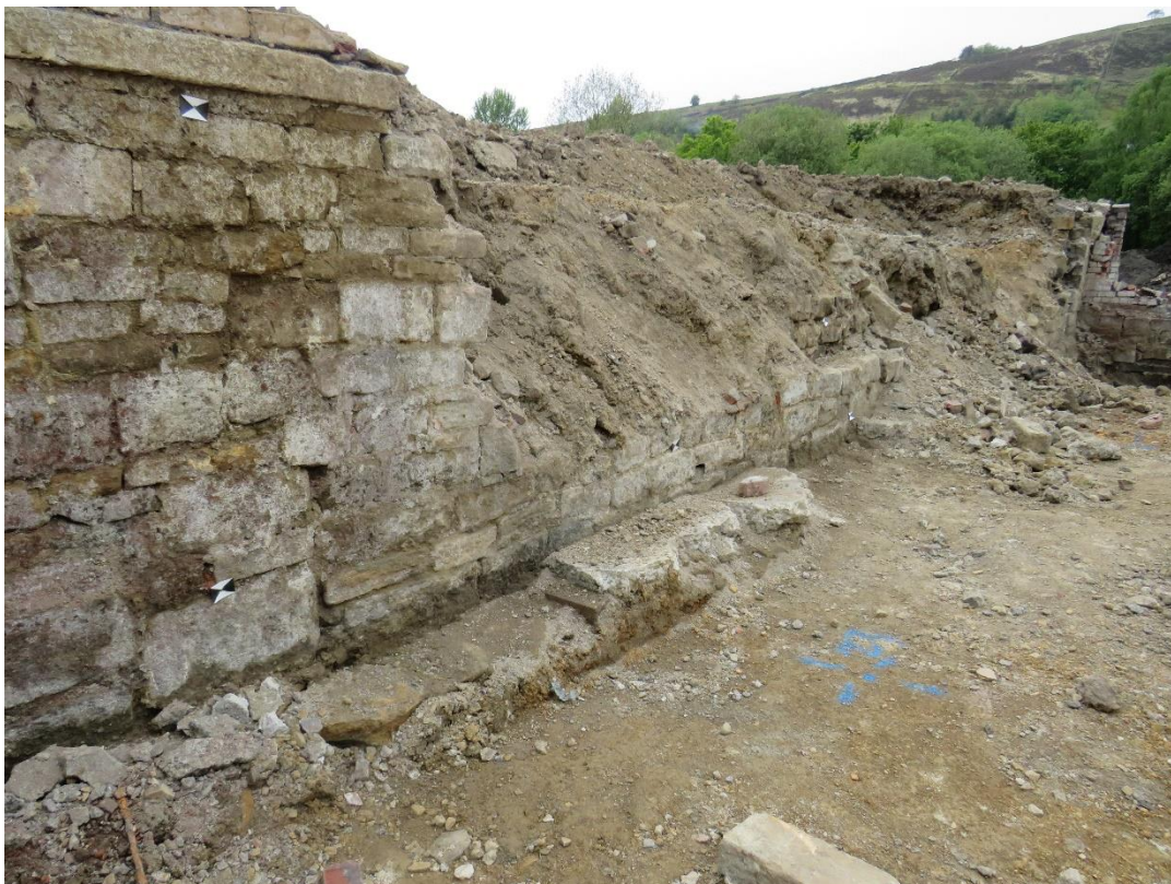
Plate 30: North-east-facing elevation of the south-western wall, facing south-west, with a window lintel (left) and the remnants of a floor (centre)
