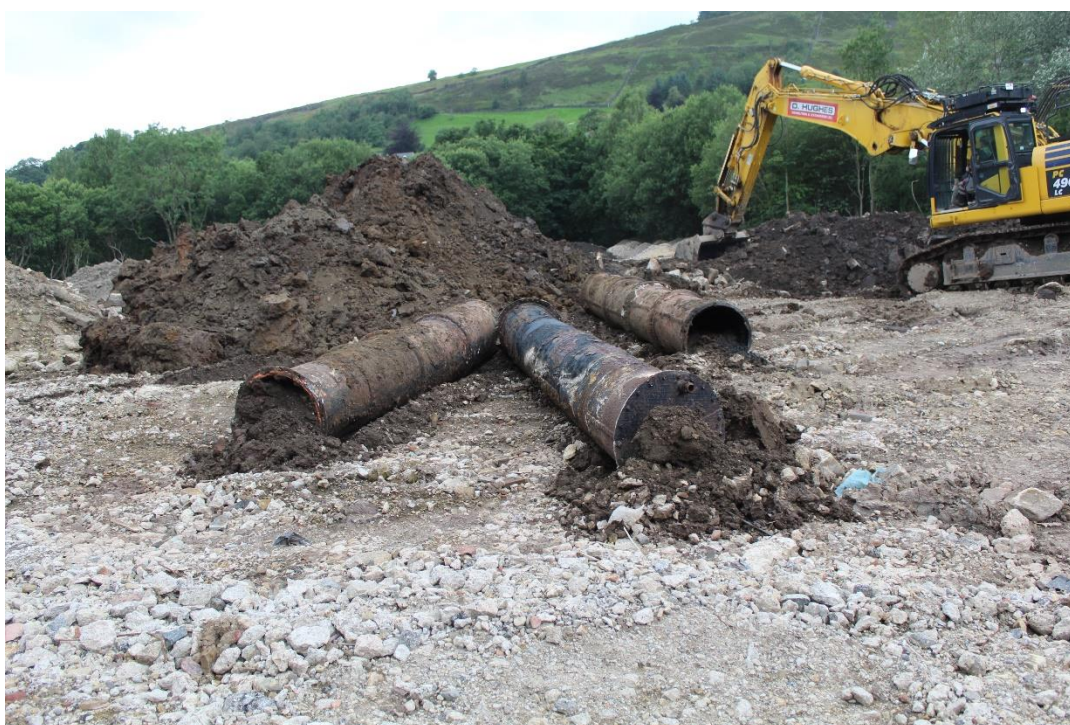
Plate 45: The removed pipework associated with the demolition of the retaining wall
