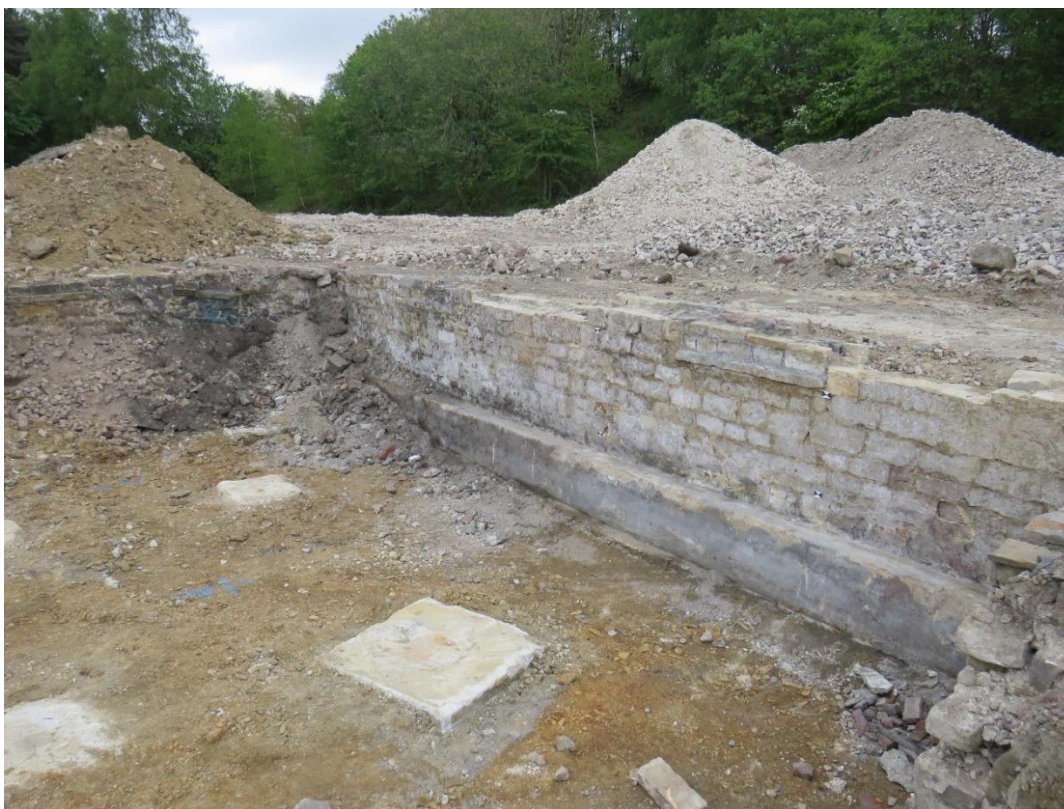
Plate 29: The south-eastern wall of Wrigley Mill, facing north
