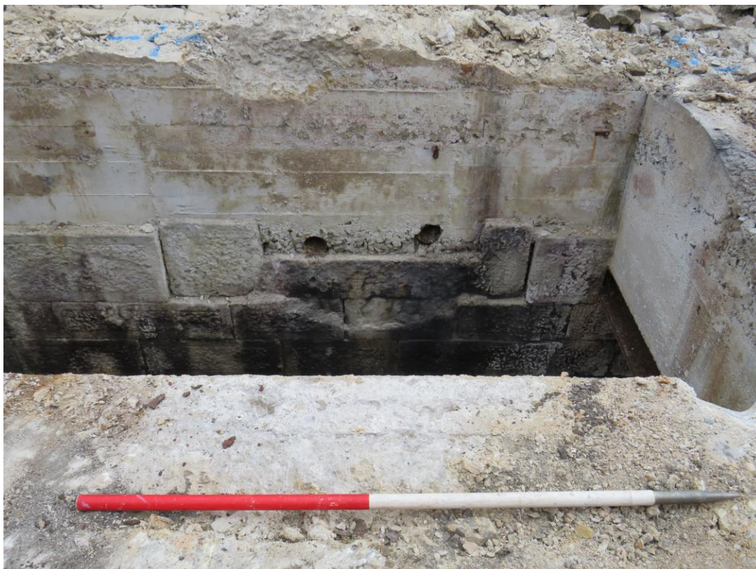
Plate 40: Recess for the waterwheel bearing below the axle-mounting point, facing south-east (with 1m scale)
