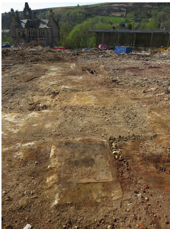
Plate 16: Rectangular pads to the north of engine house, facing west, with iron staining to the upper surface
