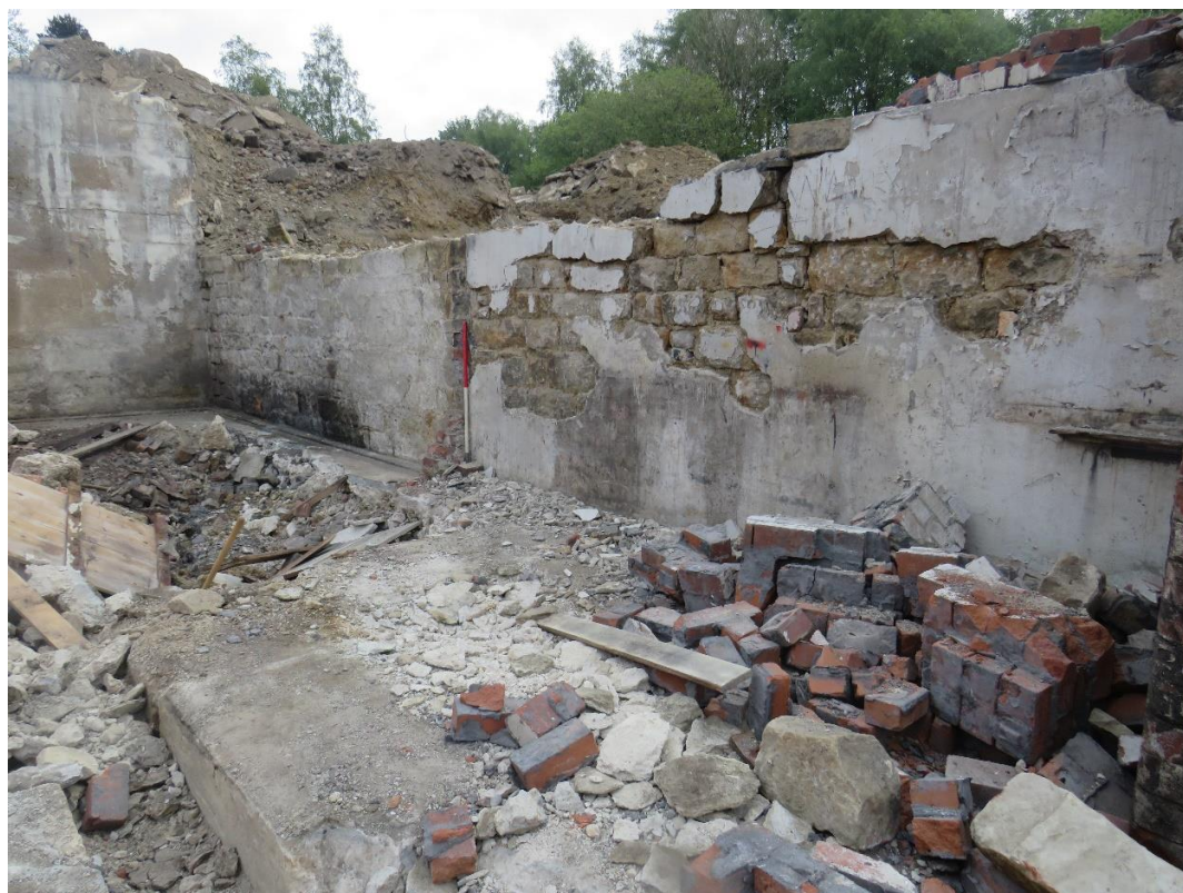
Plate 27: Wall 303, facing north-east (with 1m scale), following the removal of the later brick wall from above
