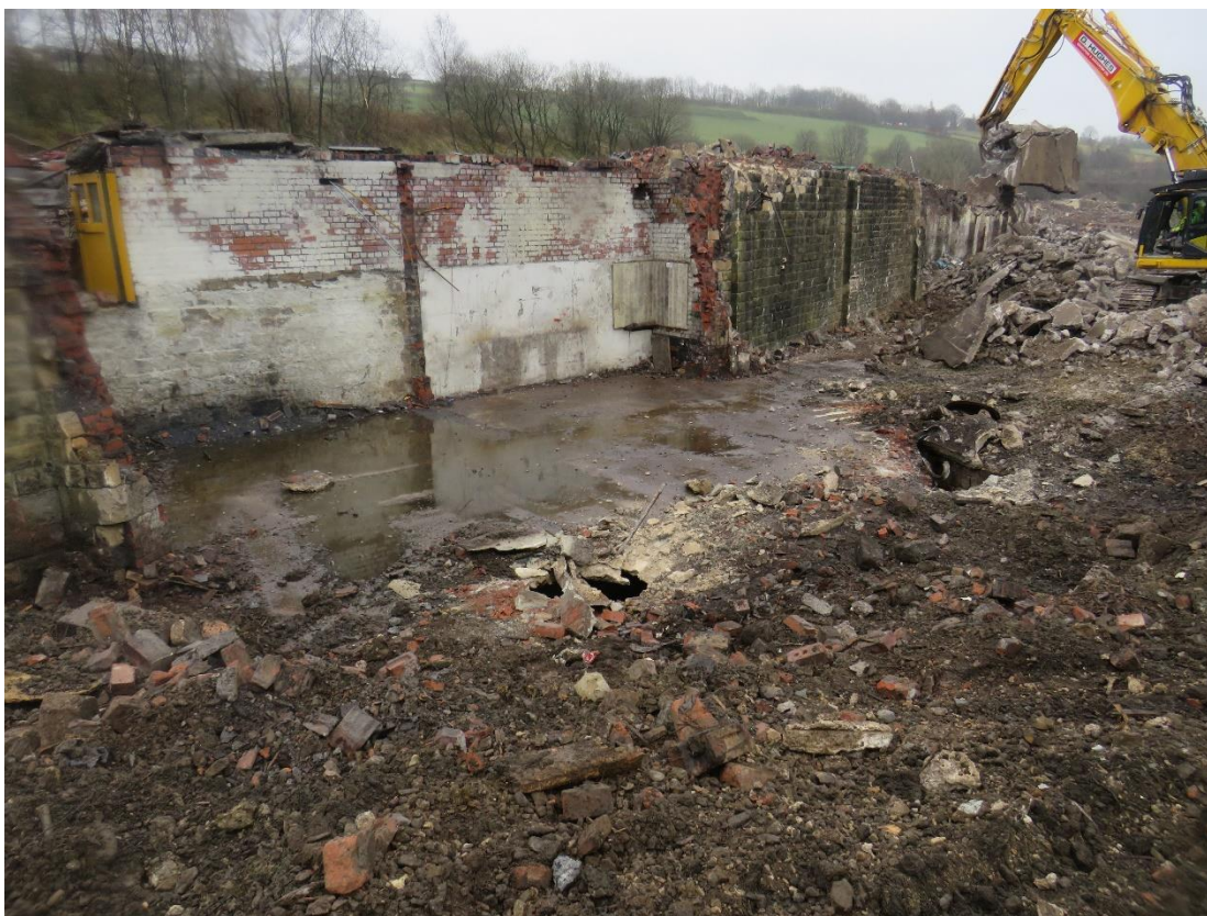
Plate 6: Area 3 during removal of the concrete slab, facing south-east, with voids appearing in the centre ground, denoting the position of the subterranean chamber
