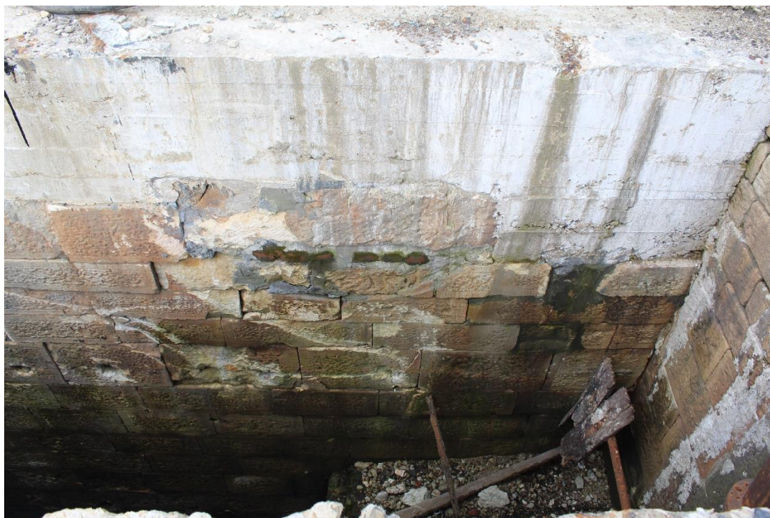
Plate 41: Recess for possible spur gear on the north-western wall
