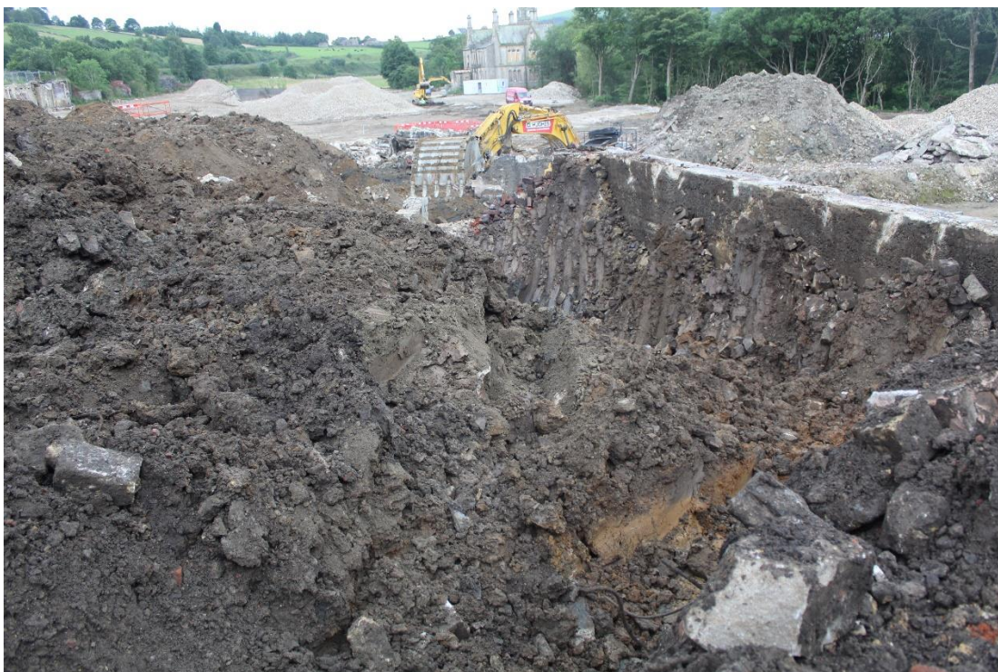
Plate 44: The demolition of the retaining wall and removal of pipework entering the waterwheel pit, from the north-west, facing south
