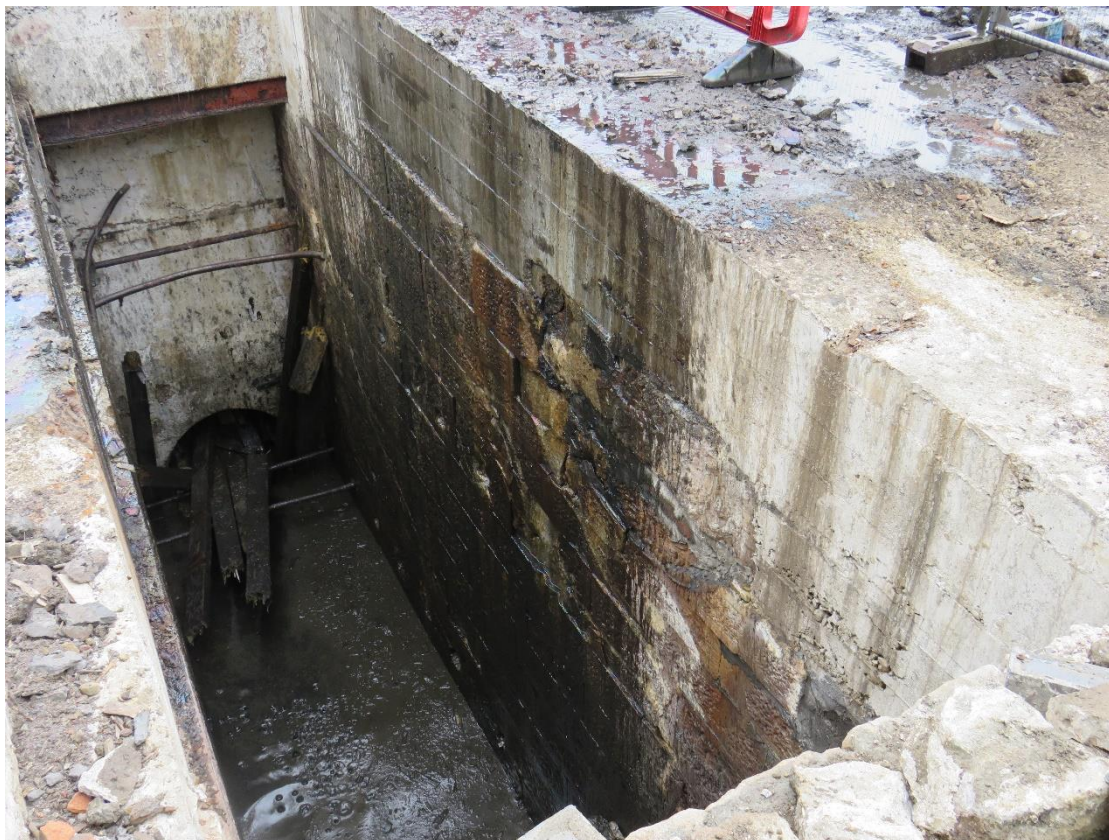
Plate 35: The waterwheel pit, facing south
