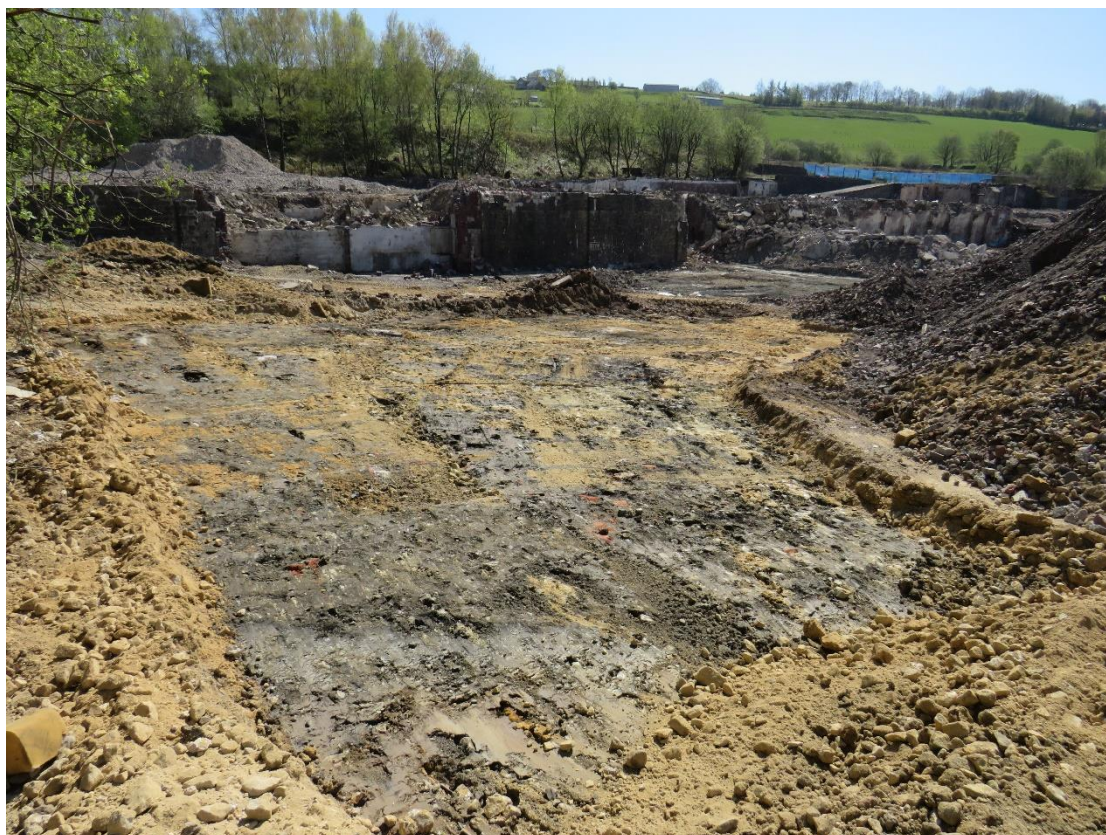
Plate 46: The reduction in levels across the western part of Wrigley Mill revealed no trace of the earlier mill
