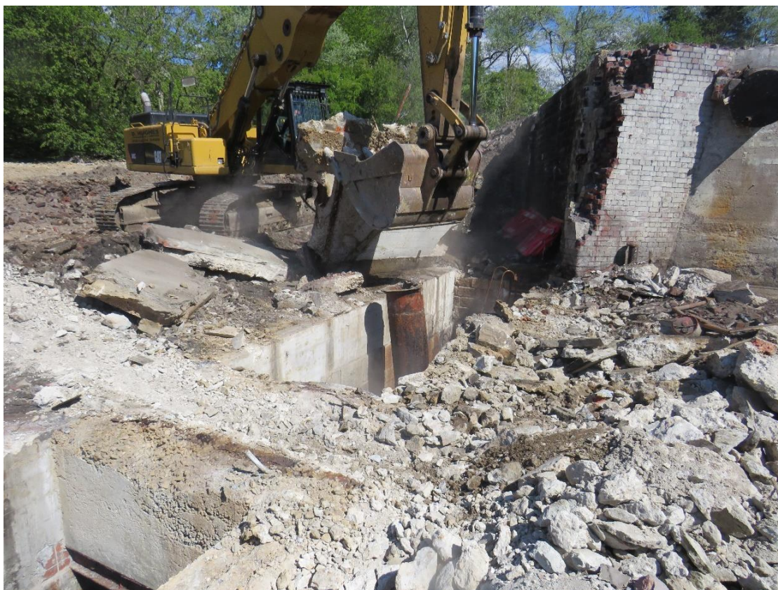
Plate 34: The subterranean chamber, during the removal of the concrete slab, facing north
