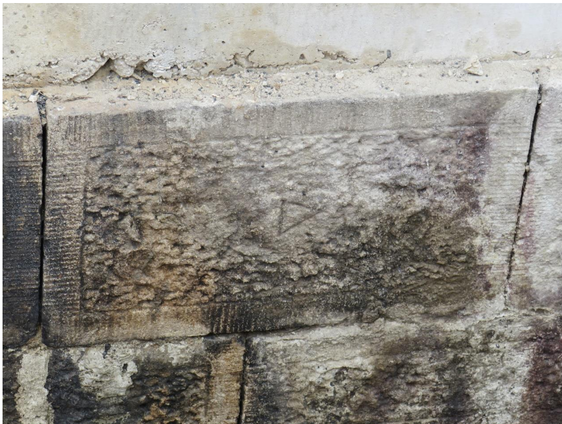
Plate 42: Possible assembly mark, indicating the centre line of the waterwheel
