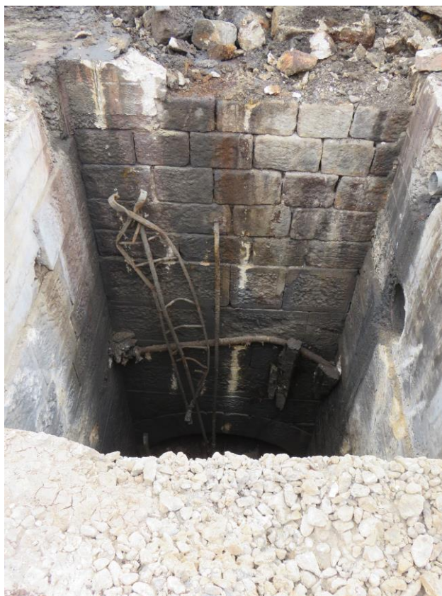
Plate 38: Coursed sandstone blocks at the south-western end of the wheel pit
