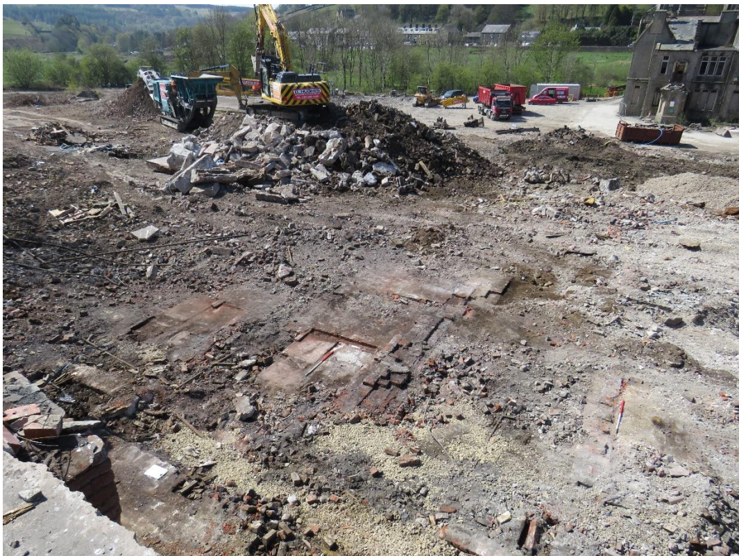
Plate 5: Area 2, during removal of the overburden, exposing brick structures, facing west (1m scale)
