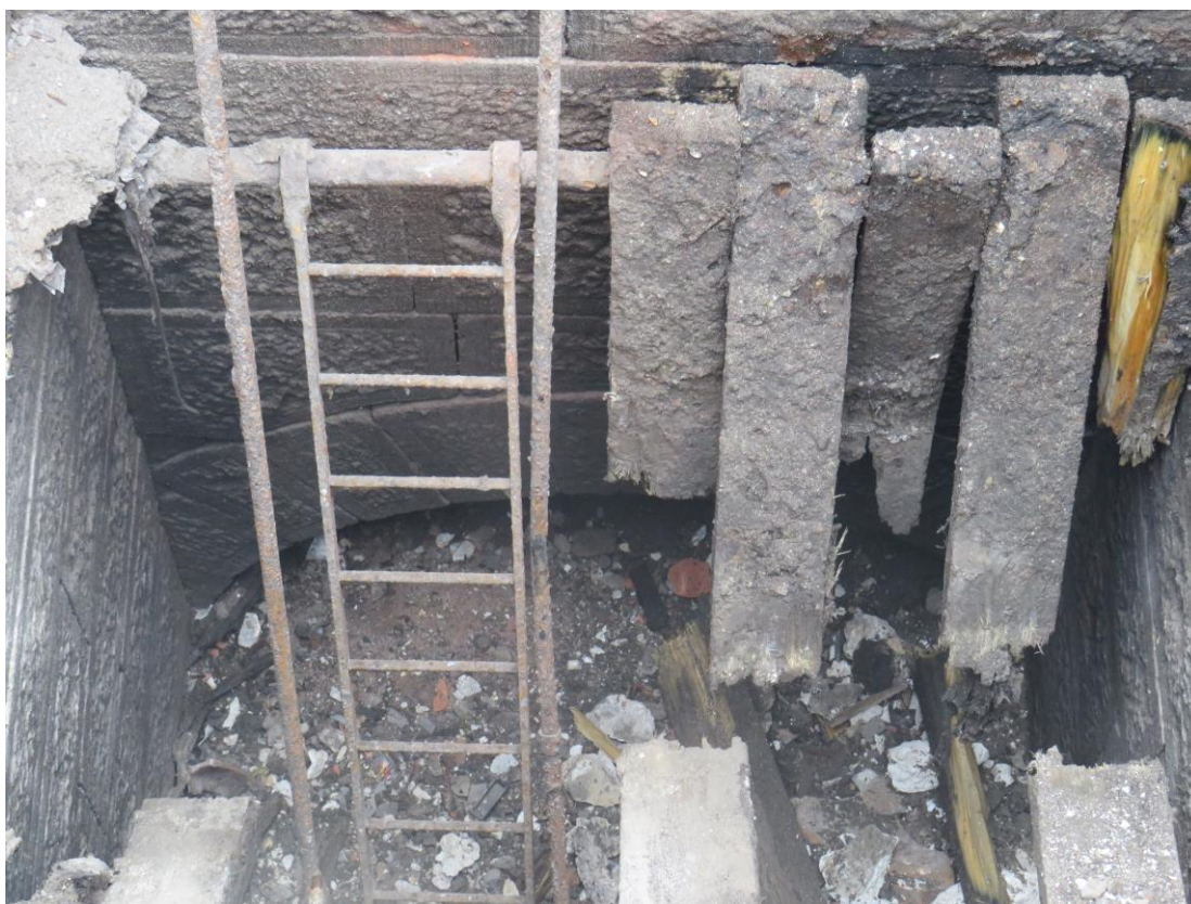
Plate 39: Semi-circular arch at the south-western end of the wheel pit
