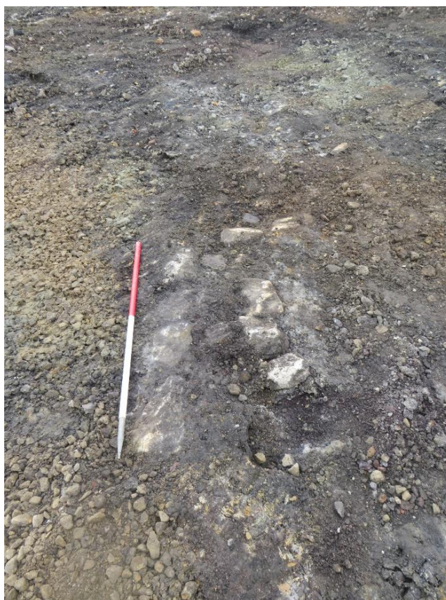
Plate 49: Wall 310 , facing south (with 1m scale)
