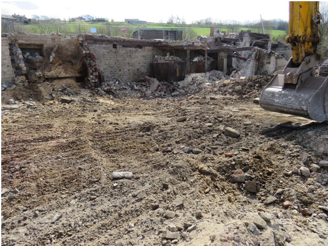
Plate 4: Removal of the concrete slab from above Area 1, exposing mixed rubble levelling adjacent to the retaining wall, facing south-east
