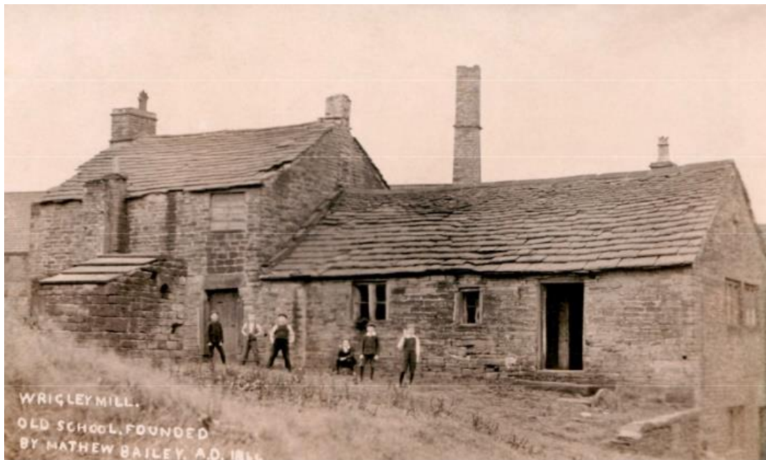
Plate 1: Nineteenth-century photograph of Wrigley Mill, possibly facing south (Saddleworth Museum Archive M/PDg/9; from SHSB 2015)
