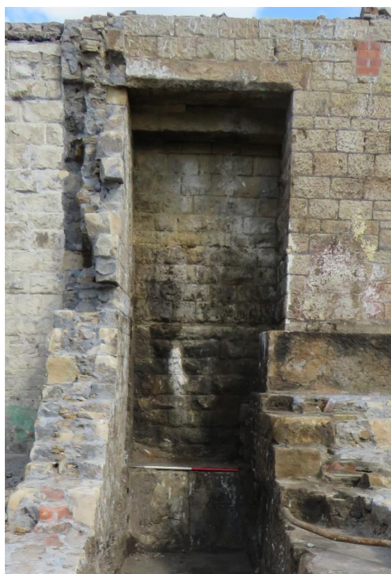
Plate 15: Recess at the northern end of the eastern retaining wall, facing east (with 1m scale)
