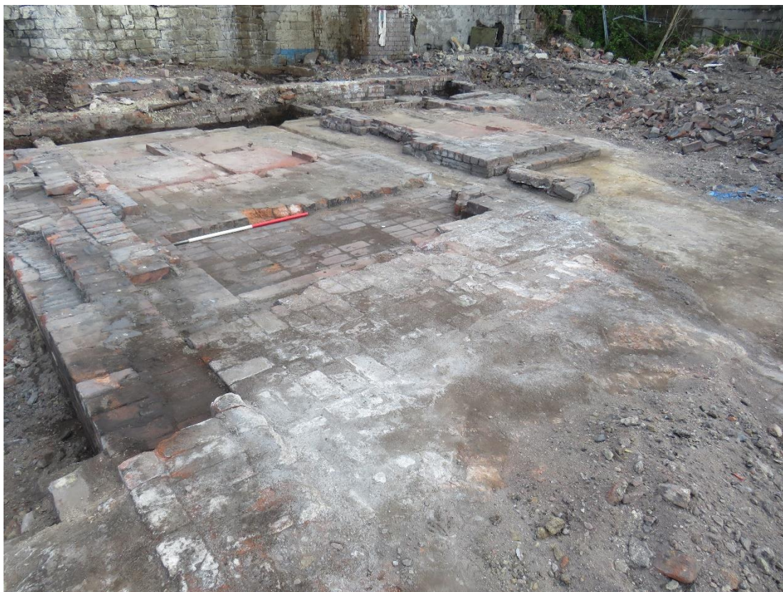
Plate 21: The northern brick structure ( 201 ), facing south-east (with 1m scale)
