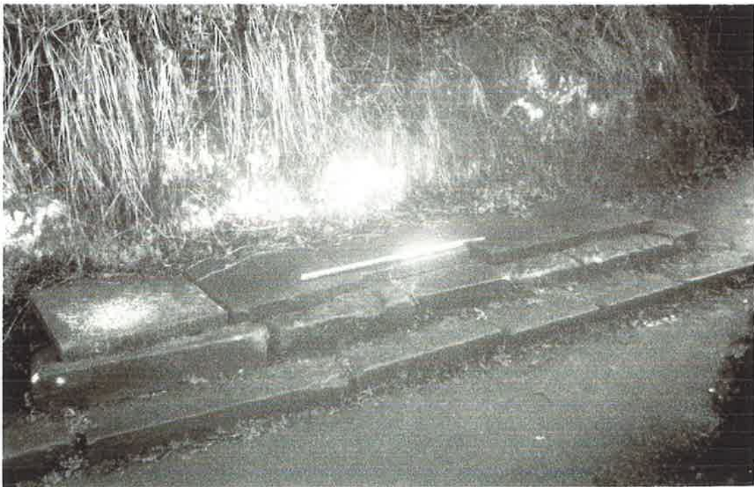
Plate 6 Dressed stones reused as a seat platform (20)
