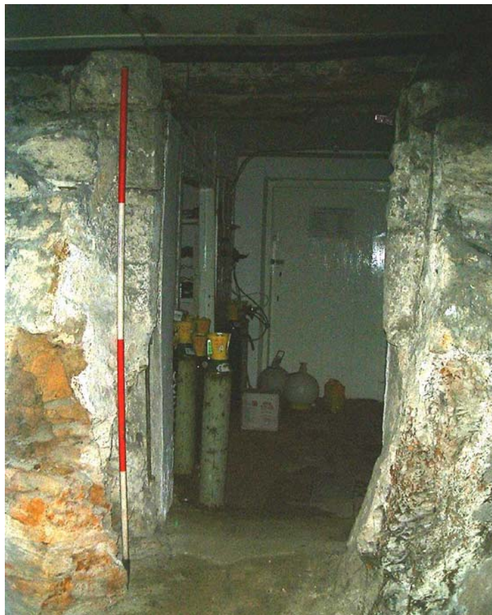
Plate 2: Early doorway in the basement of the present Henllys Hall
