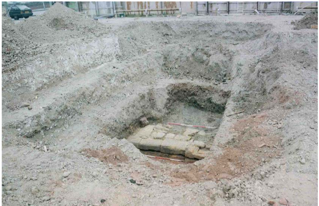
Plate 6 General view of stepped Trench 4 showing Dock Wall – looking south
