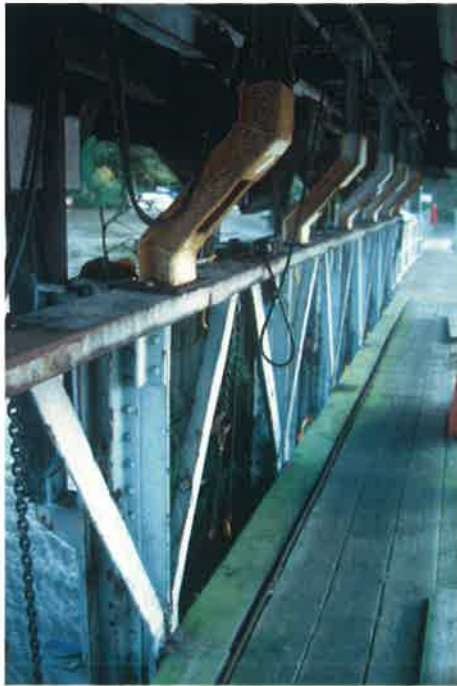
Plate 13: North-east view of buck gate weir gallery
