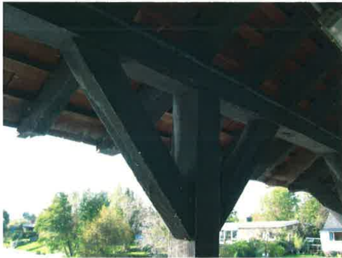
Plate 11: South-west view of the buck gate weir gallery roof
