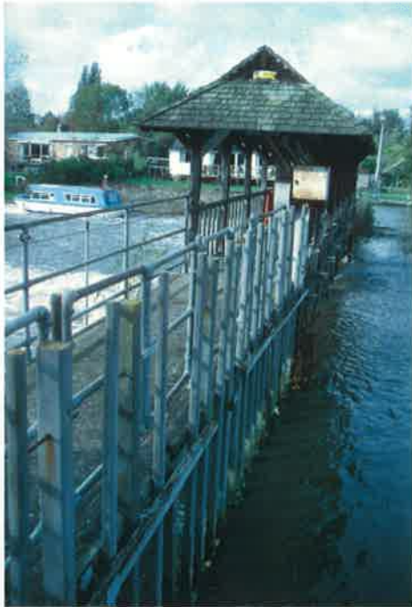
Plate 5: West view of east paddle and rymer bay
