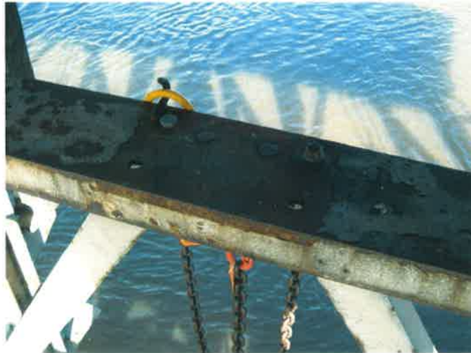
Plate 19: North view showing holes relating to former hand-winch system
