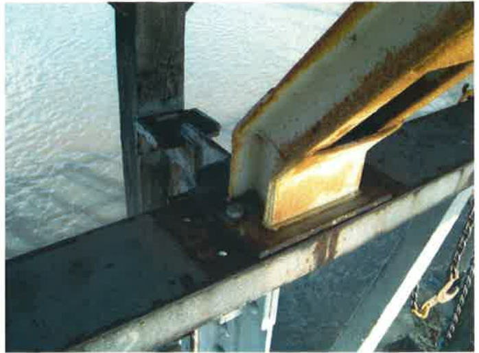
Plate18: North-east view showing holes relating to former hand-winch system
