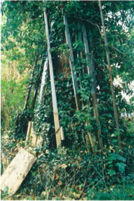
Plate 9: Former paddle rack east of 'B' weir
