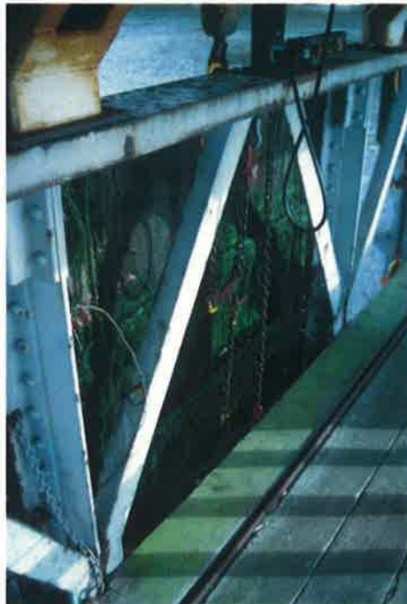
Plate 12: North-east view of buck weir gate
