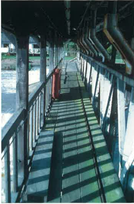
Plate 17: West view showing grooves in gangway floor for operation of hand-winch
