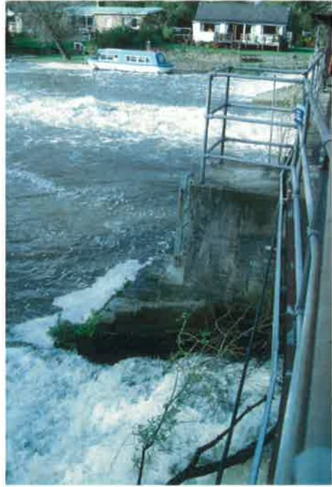
Plate 10: West view of masonry pier
