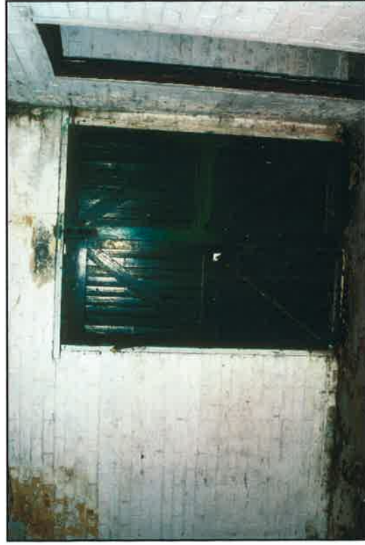
Plate 27: Internal door, east elevation, block A
