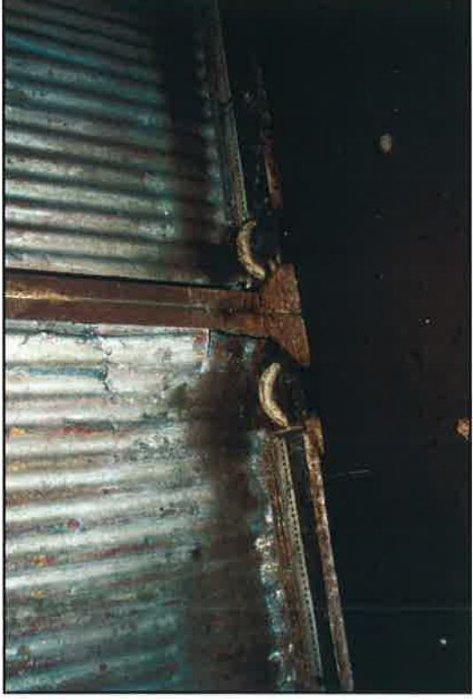
Plate 10: Rolling mechanism of sliding doors, north-east elevation
