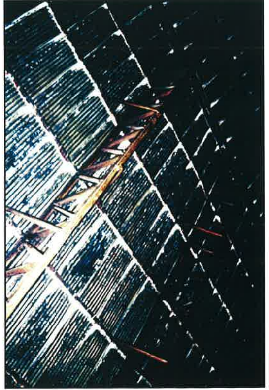
Plate 19: Internal west view of roof
