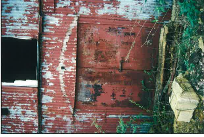
Plate 14: Doorway 2, south-east elevation
