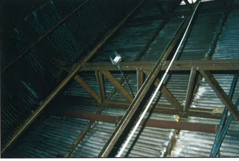
Plate 18: Roof truss, south-east elevation
