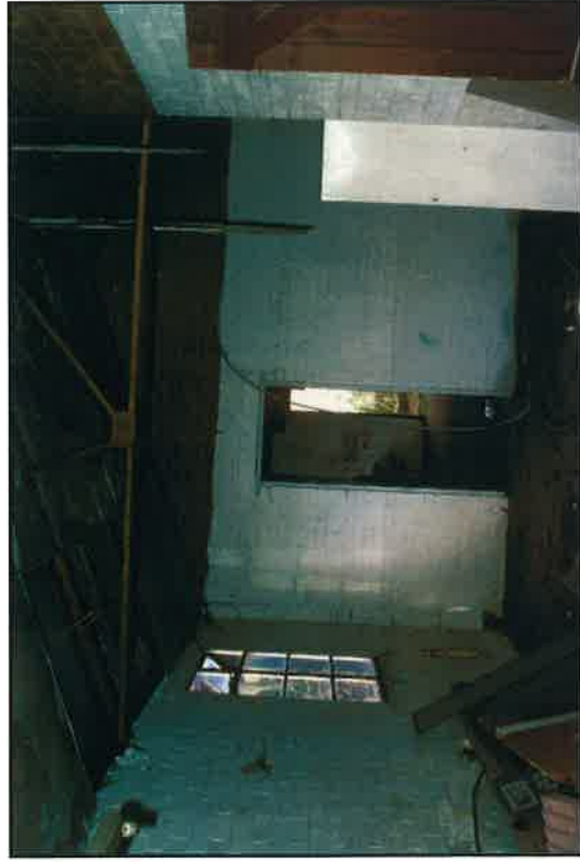
Plate 25: Internal south view of block A
