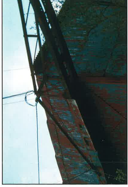
Plate 12: Overhang structure of sliding doors, south-west elevation
