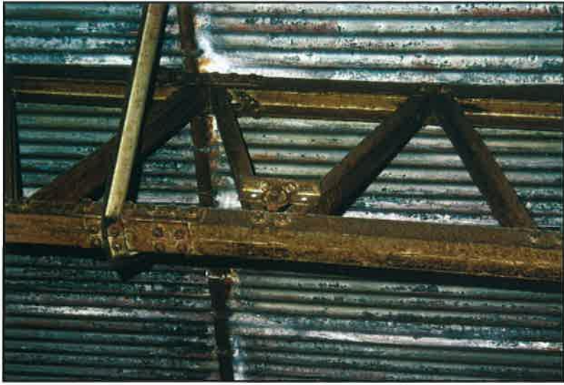
Plate 21: Detail of internal pulley mechanism, south-west corner
