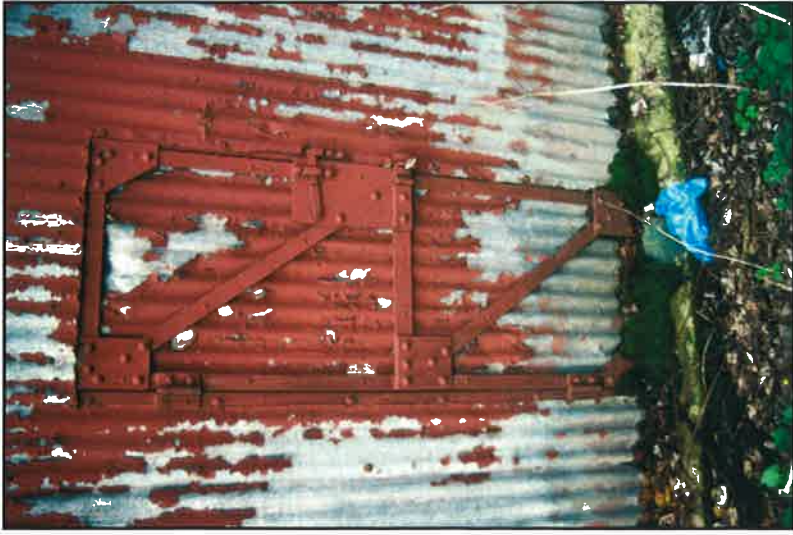
Plate 13: Doorway 1, south-east elevation
