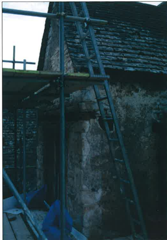
Plate 21: West elevation, third floor showing exposed timber
