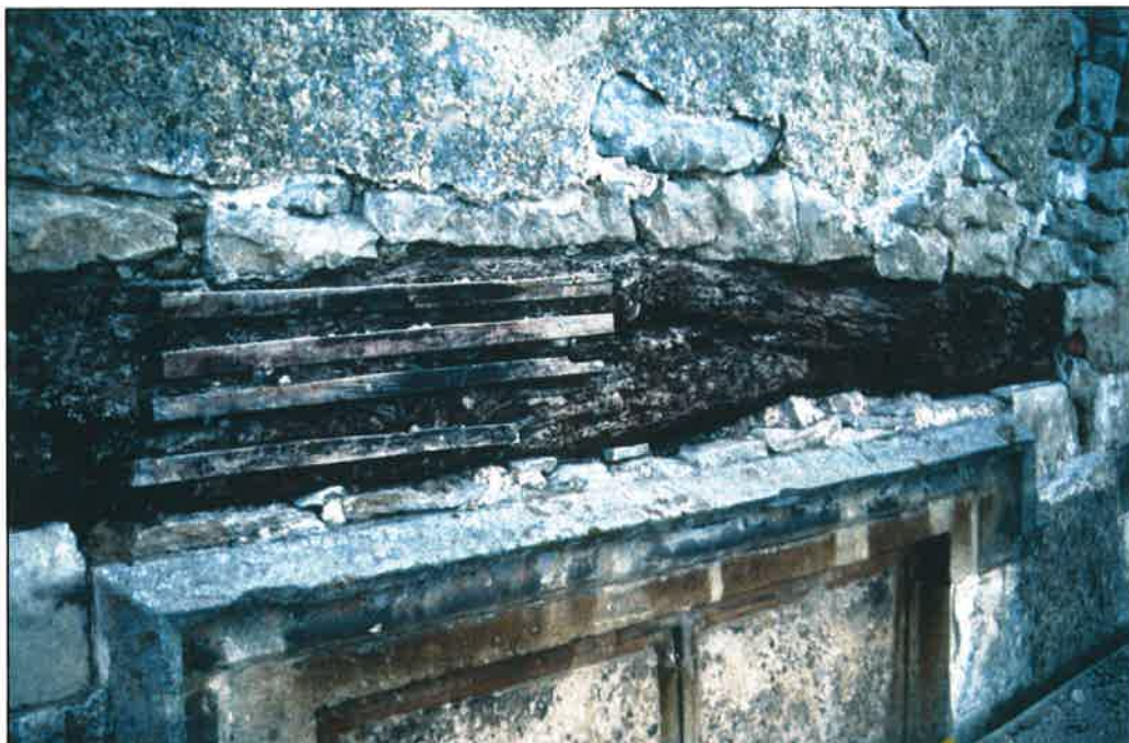
Plate 14: East elevation, third floor showing exposed timber
