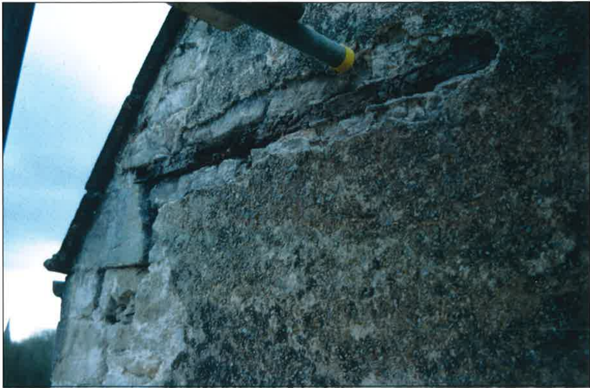
Plate 9: North elevation, third floor showing exposed timber
