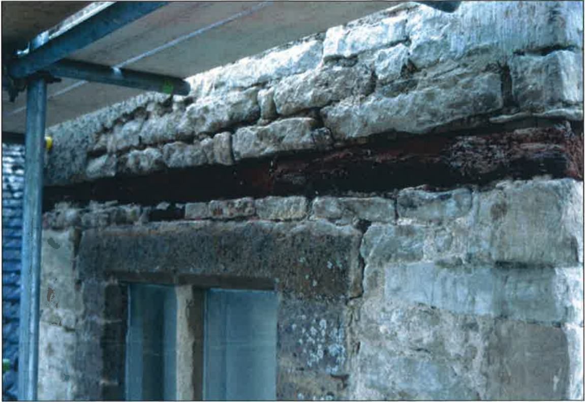
Plate 7: North elevation, third floor showing exposed timber
