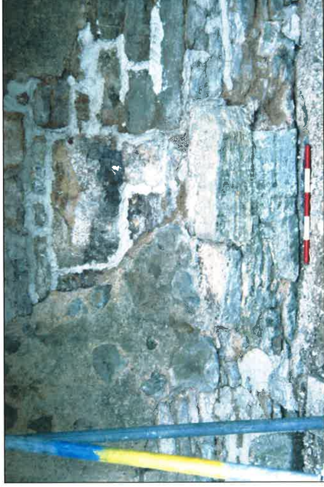
Plate 2: North elevation, ground floor showing plinth and infill
