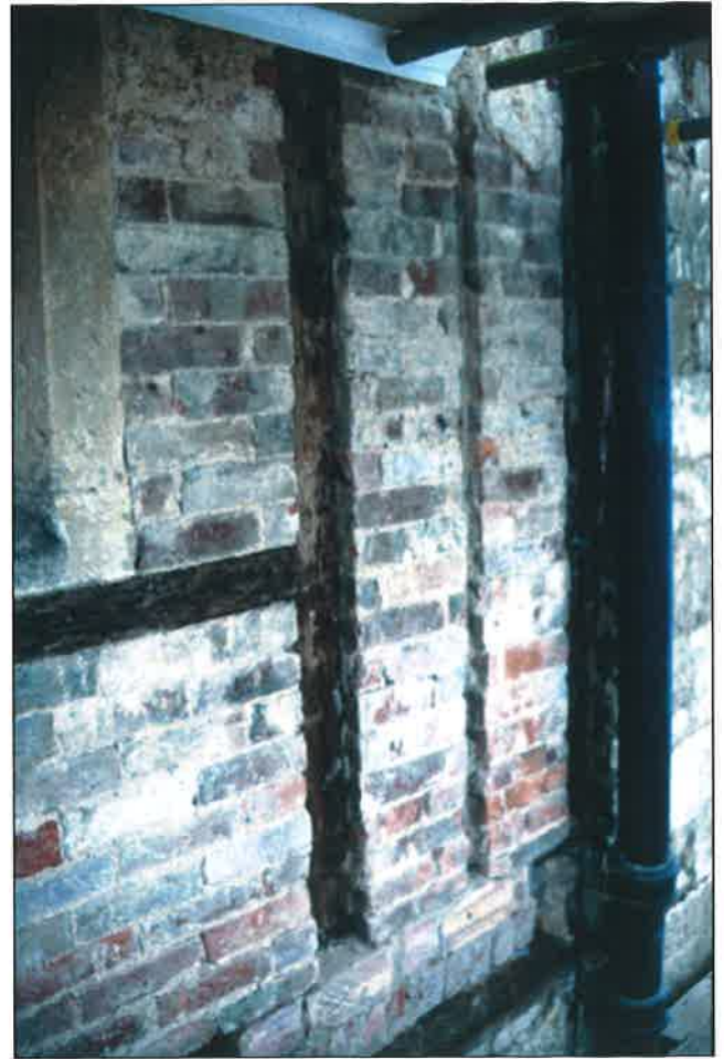
Plate 18: West elevation, first floor showing exposed timber
