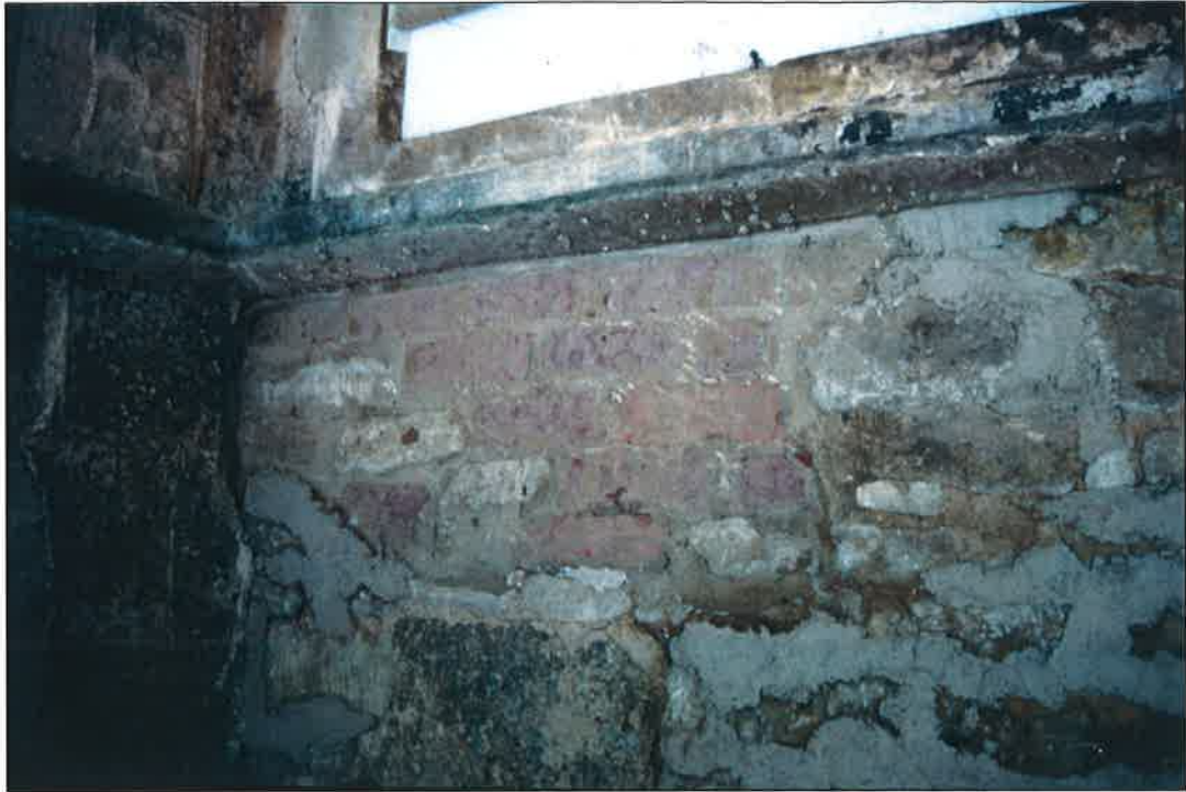
Plate 11: East elevation, first floor showing exposed red brick
