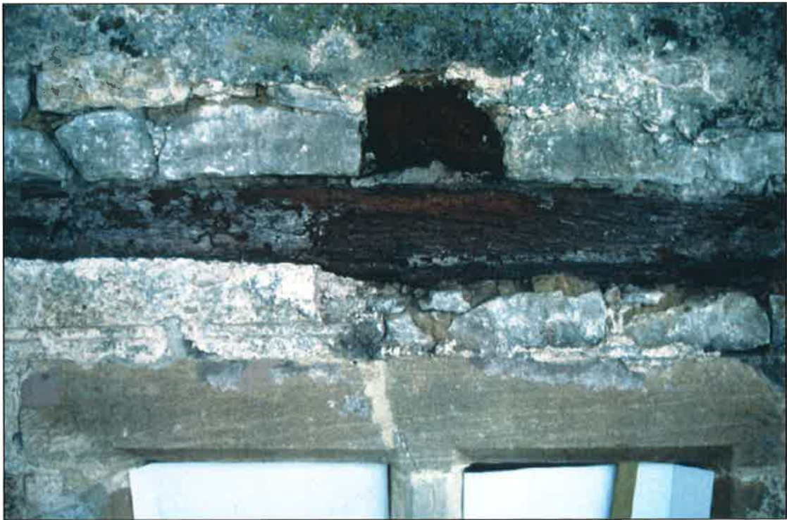
Plate 8: North elevation , third floor showing exposed timbers
