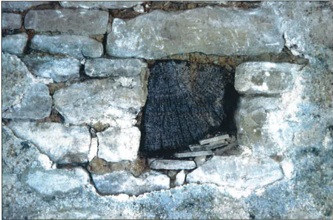
Plate 5: North elevation, first floor showing exposed cross timber
