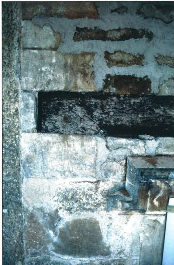
Plate 12: East elevation, first floor showing exposed timber
