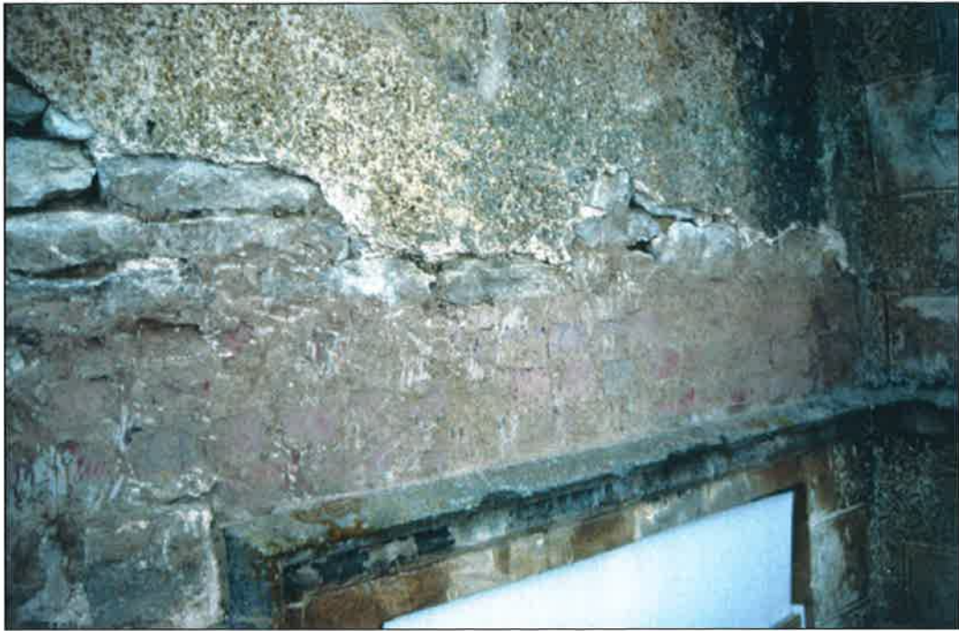
Plate 15: East elevation, third floor showing red brick repair
