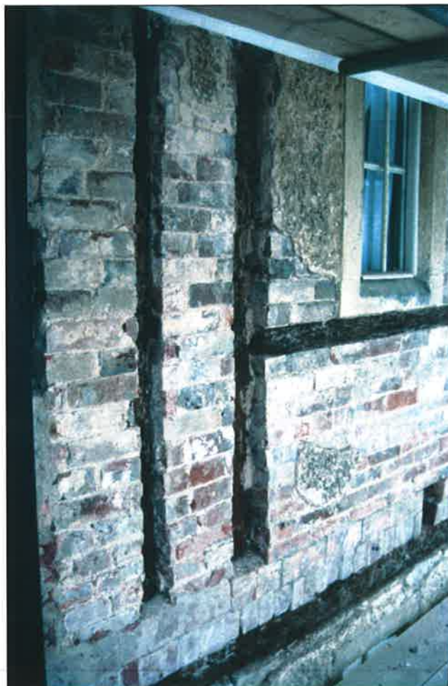
Plate 19: West elevation second floor showing exposed timbers to south
