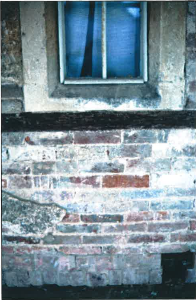
Plate 17: West elevation, first floor showing red brick repair and exposed timber
