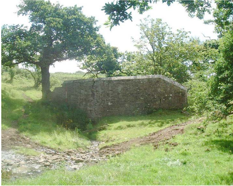
Plate 1: Scalegill Bridge (Site 11), north facing elevation
