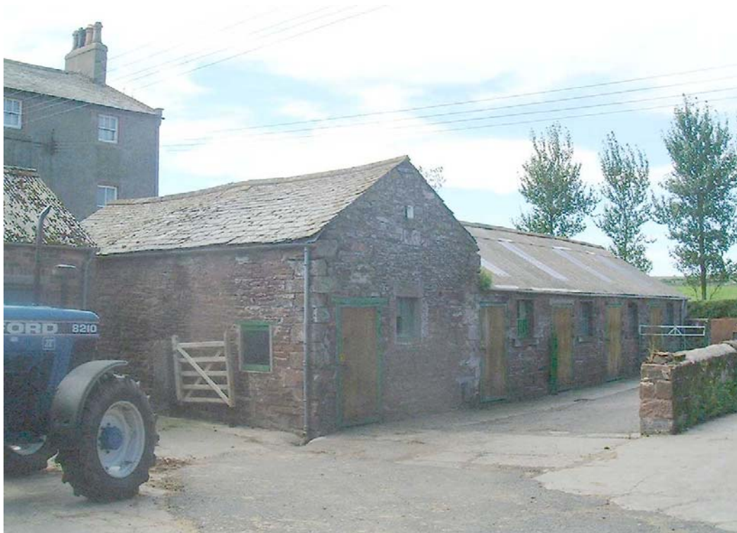
Plate 7: Low Hall Farm Stable Block (Site 10) from the north-east
