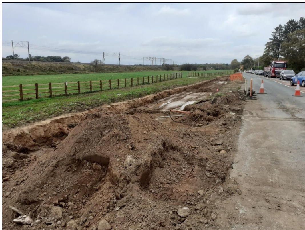
Plate 2: Location of permanent highway fence line with Asset 35 behind
