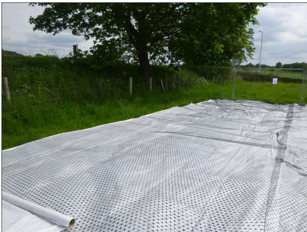
Plate 1: Geogrid and terram covering
