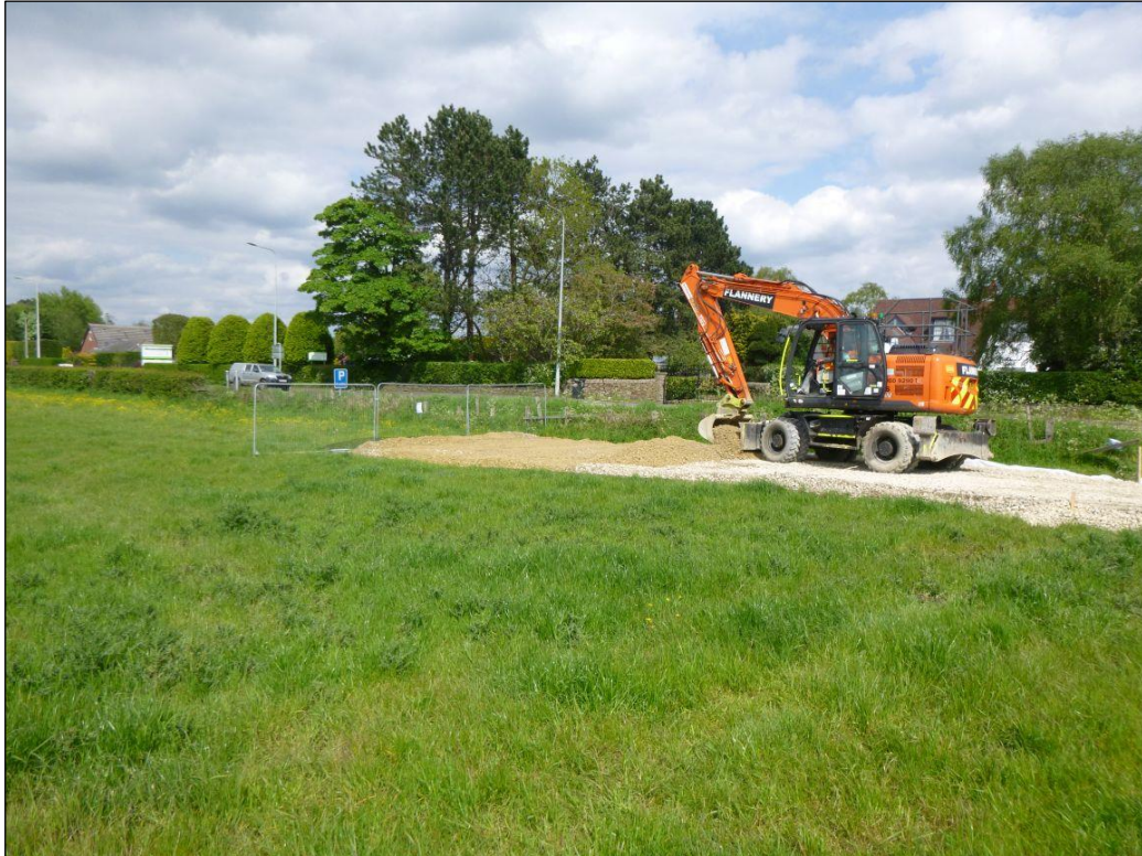
Plate 2: Stone covering being laid
