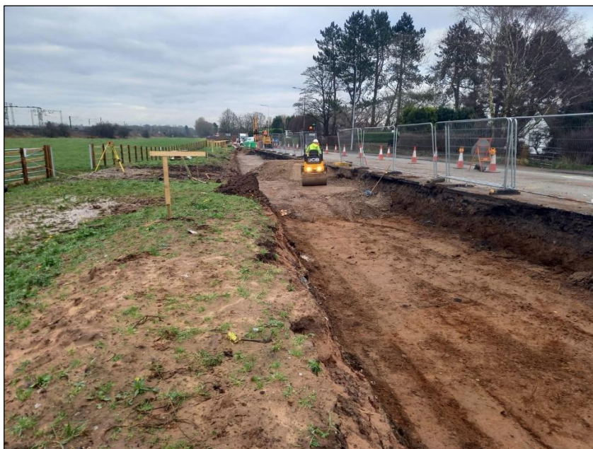
Plate 9: Excavations complete and building the level back up with crushed and compacted stone
