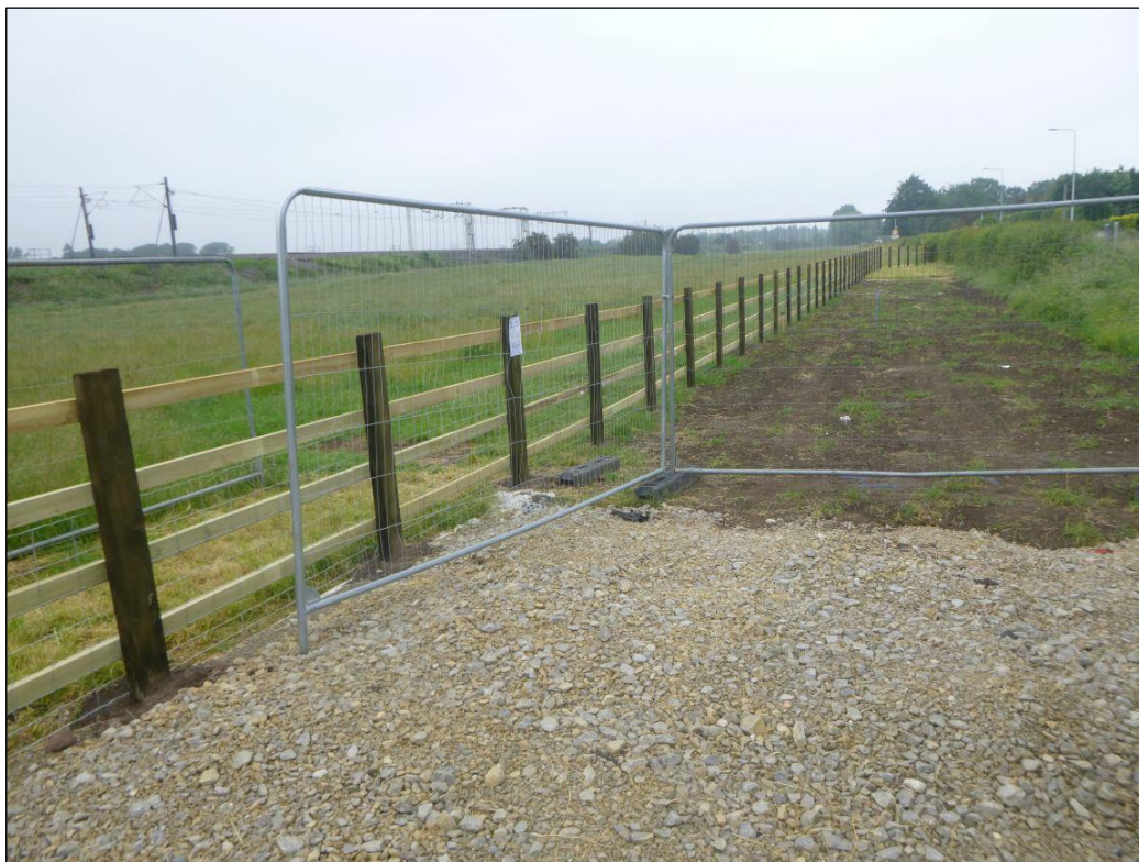
Plate 4: Fencing installed, looking north-east
