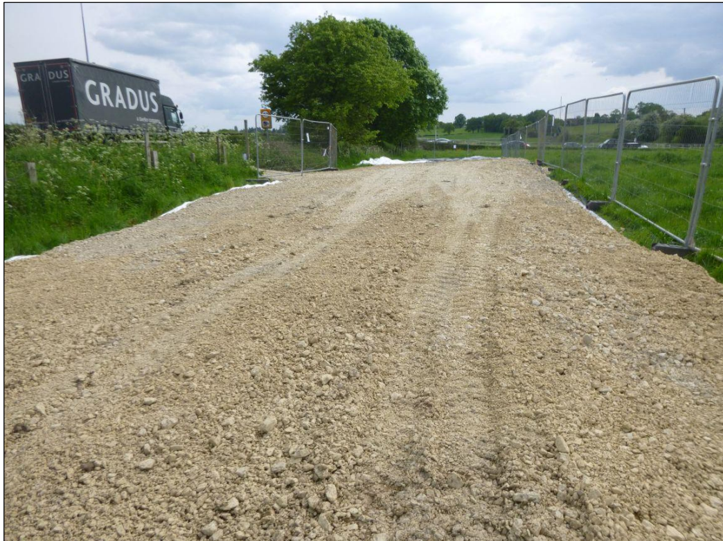
Plate 3: Covering of the monument completed
