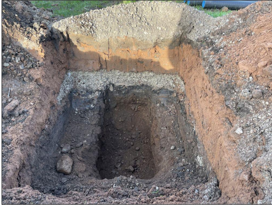
Plate 11: East-facing section of northern lamp post pit
