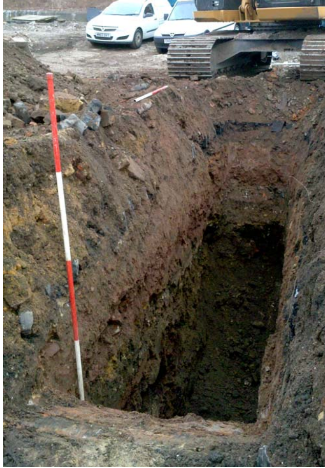
Plate 32: Area C Crane Trench 2C
