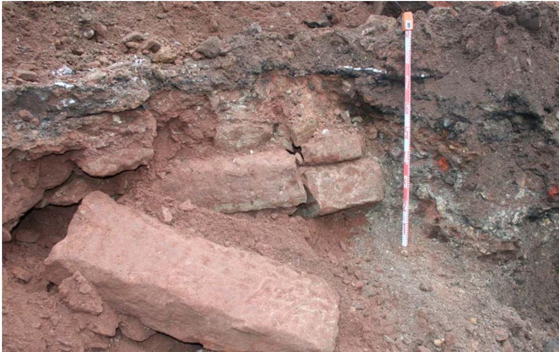
Plate 6: Sandstone retaining wall 011 at the north-eastern side of Area A
