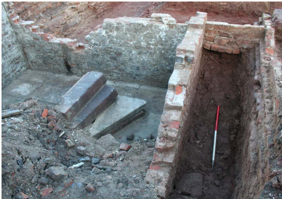
Plate 19: East-facing view across the cellar area showing walls 135 , 136 and 137
