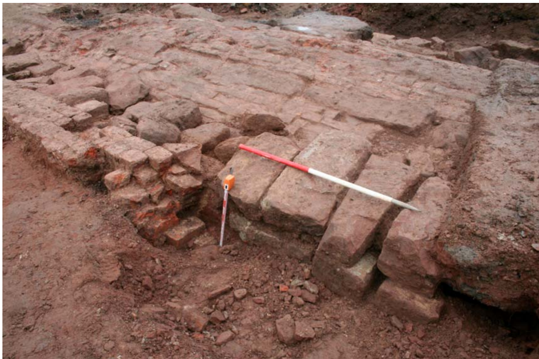
Plate 15: Sandstone levelling, 123 , placed along the extrados at the southern side of Tunnel 1, 125
