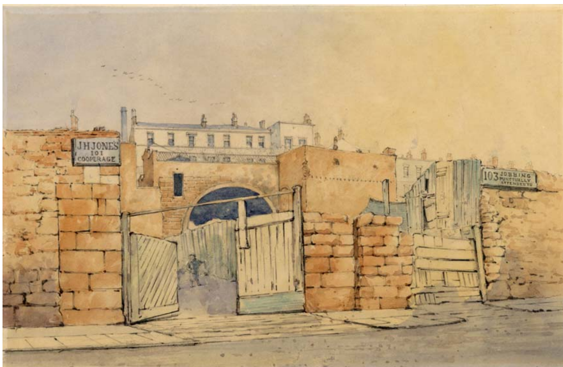
Plate 5: Painting by William Gawin Herdman showing the gates to the Cooperage with the triple decker tunnel and Mason Street in the background c 1837 (LRO)
