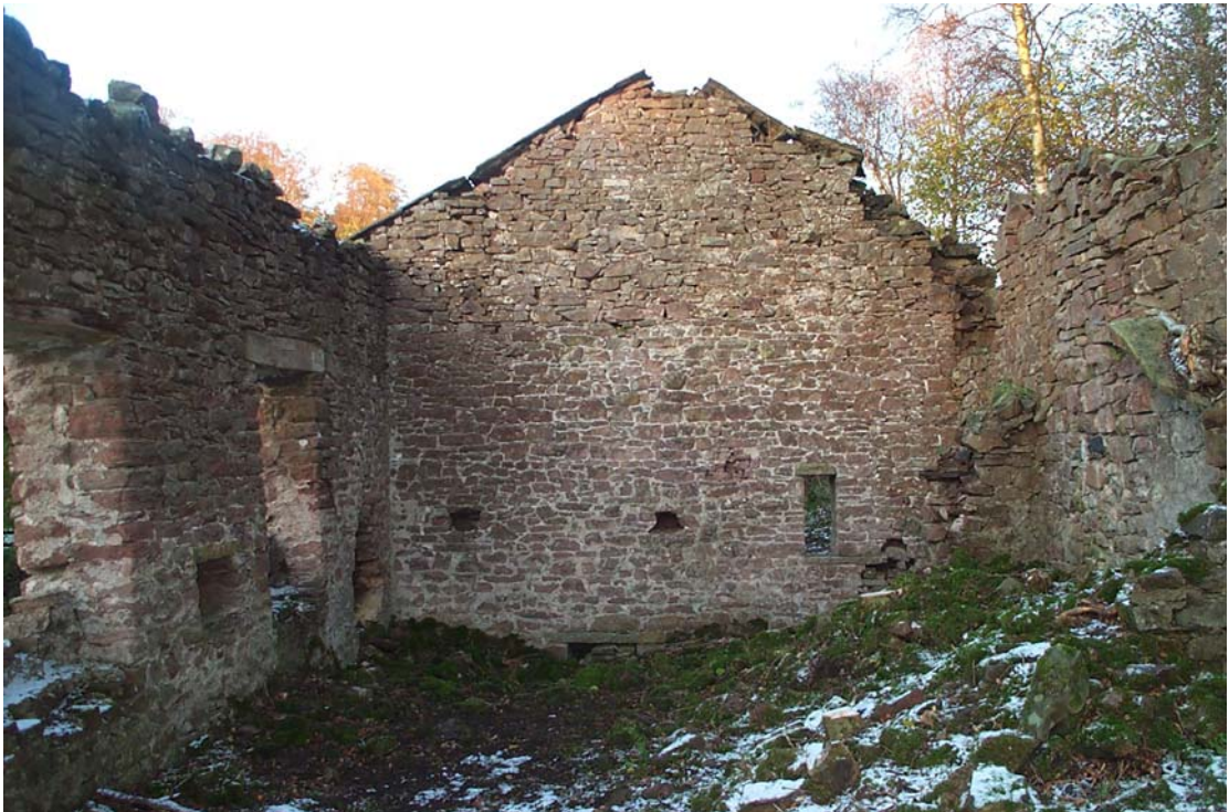
Plate 8: North Internal Elevation, Room 1
