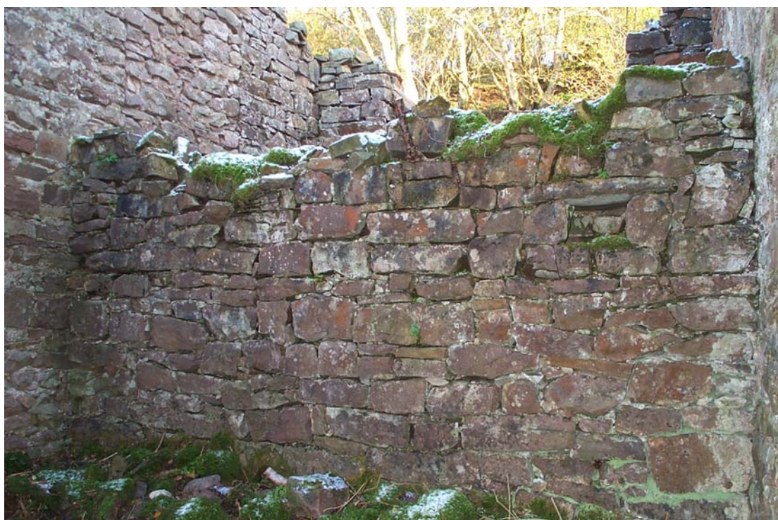
Plate 6: Partition Wall in Room 2 looking North-East
