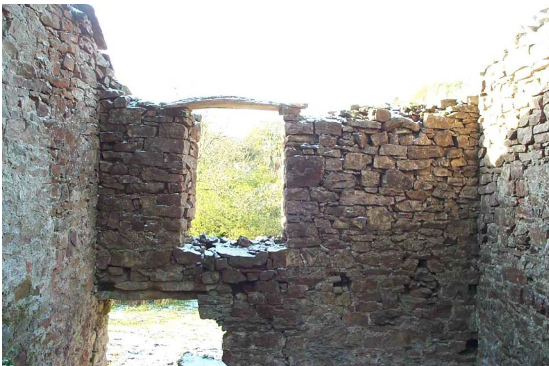
Plate 10: West Internal Elevation, Room 2
