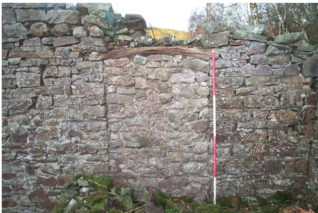
Plate 4: Blocked Doorway Between Rooms 1 and 2
