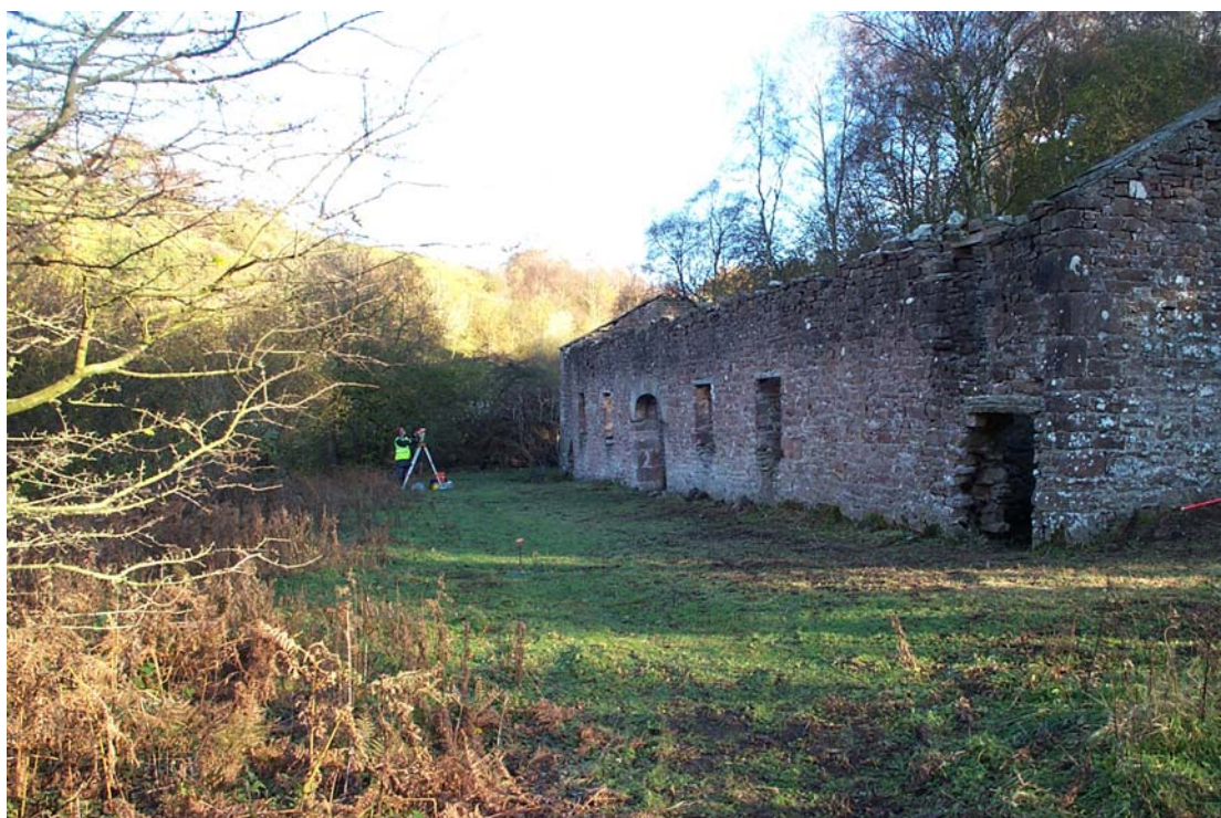
Plate 2: General View of Smelt Mill looking North-East
