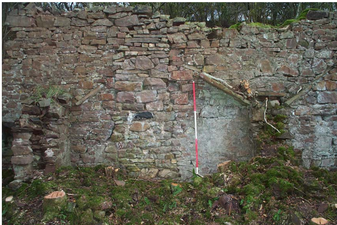
Plate 5: Blocked Hearth in the East Internal Elevation
