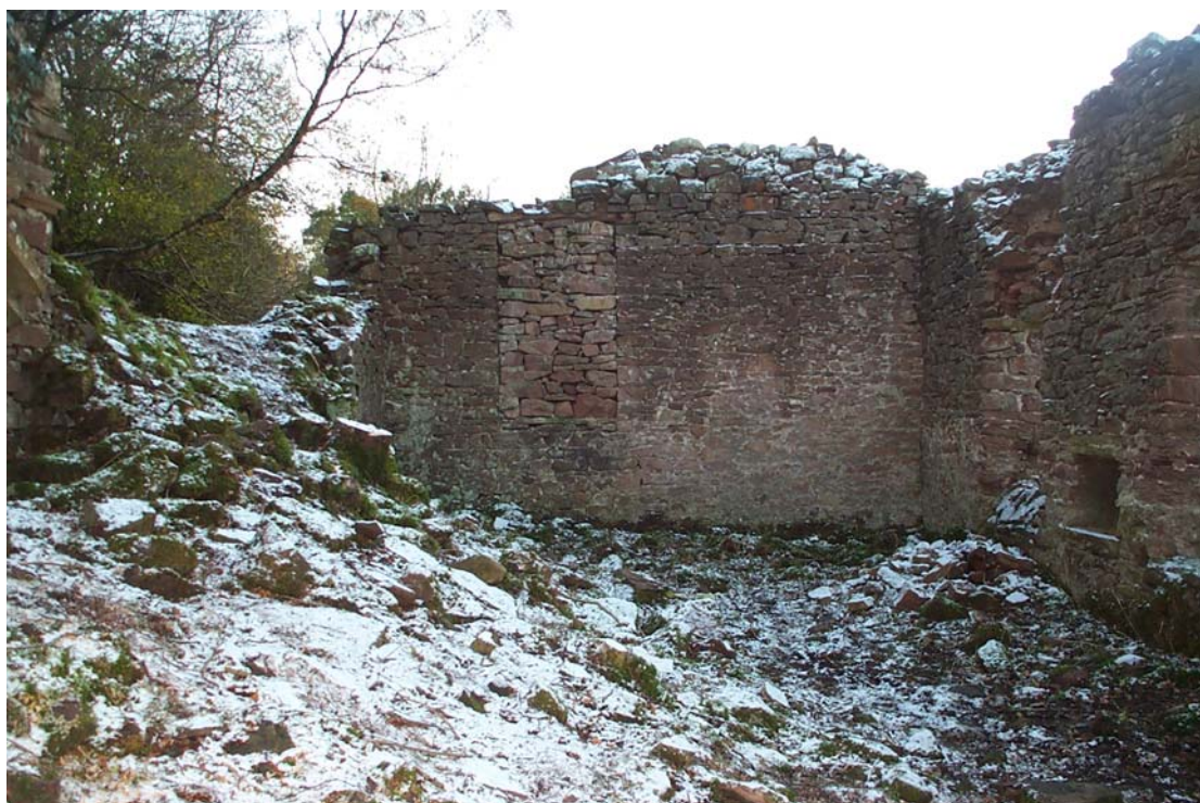
Plate 9: South Internal Elevation, Room 1
