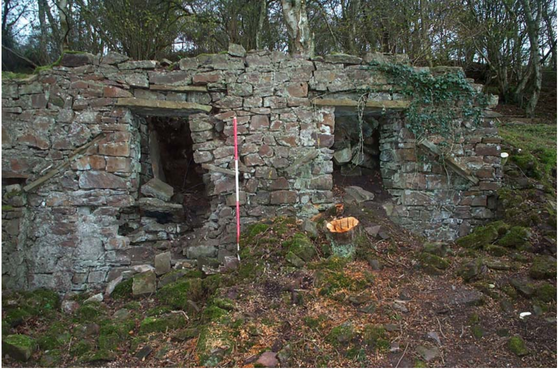
Plate 7: The Two Surviving Hearths in the Internal East Elevation
