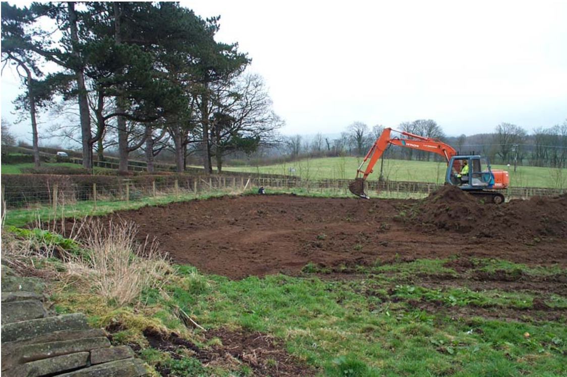
Plate 1: General view of topsoil stripping, looking south
