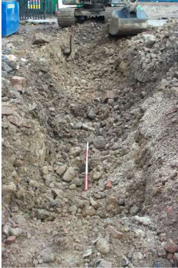
Plate 3: Cobble Backfill in piling trench north of Blocks 31-34
