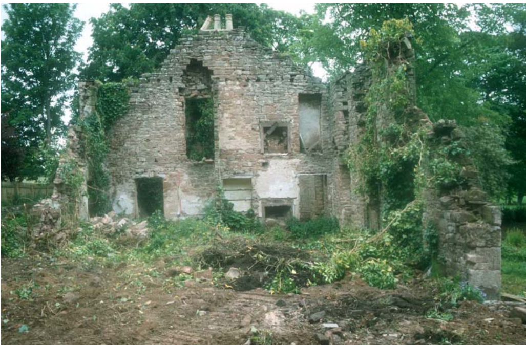
Plate 2: Internal cross wall [3] following selective removal of the ivy
