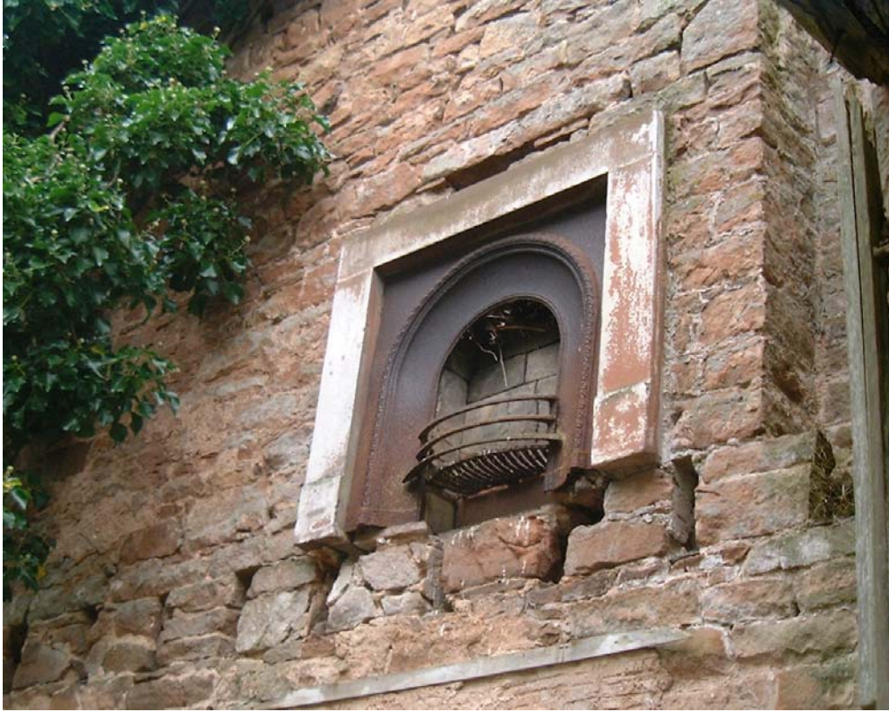
Plate 3: First floor fire place on the North Wall [2]
