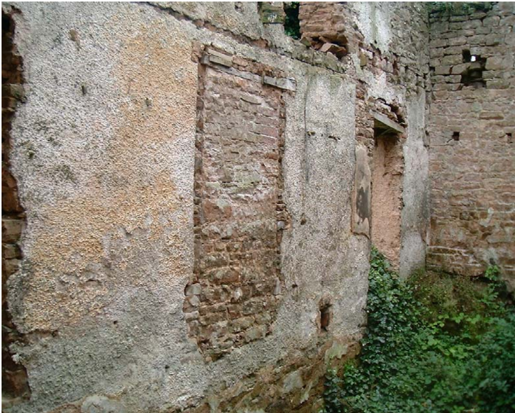
Plate 4: Northern face of the internal cross wall [3]
