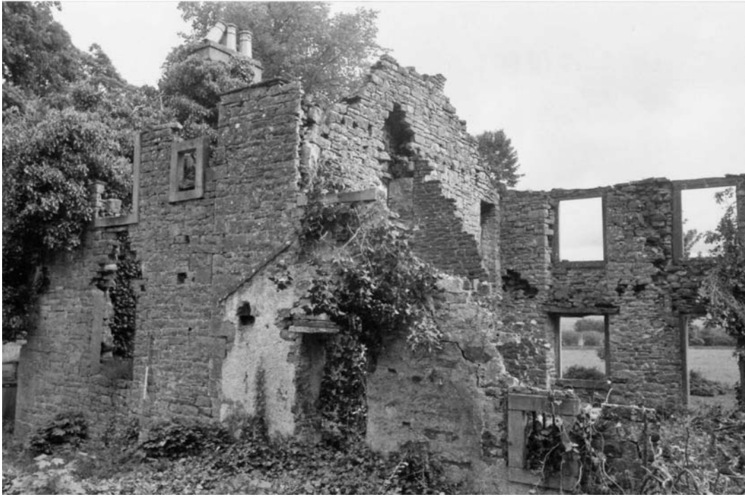
Plate 5: General view of the mansion looking north-east
