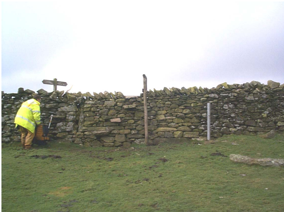
Plate 4: Site 11 Blocked gateway (looking west)
