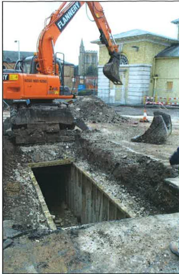
Plate 1: External north-east view of northern shelter and library.
