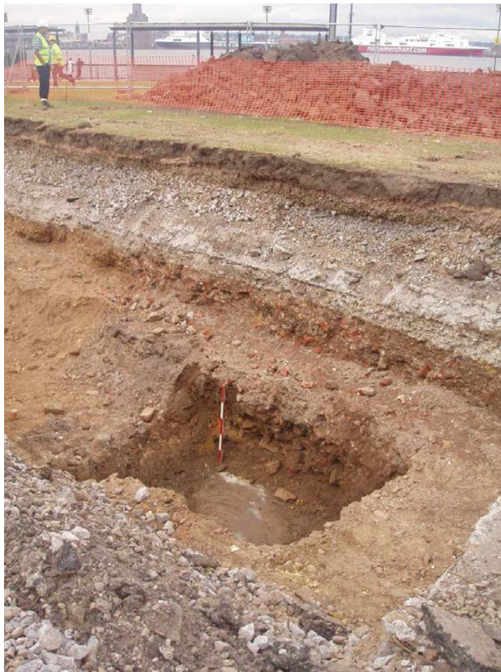
Plate 14: Trench 406, showing the large cut feature 3040 , with the concrete 3068 visible at the base, looking south-west
