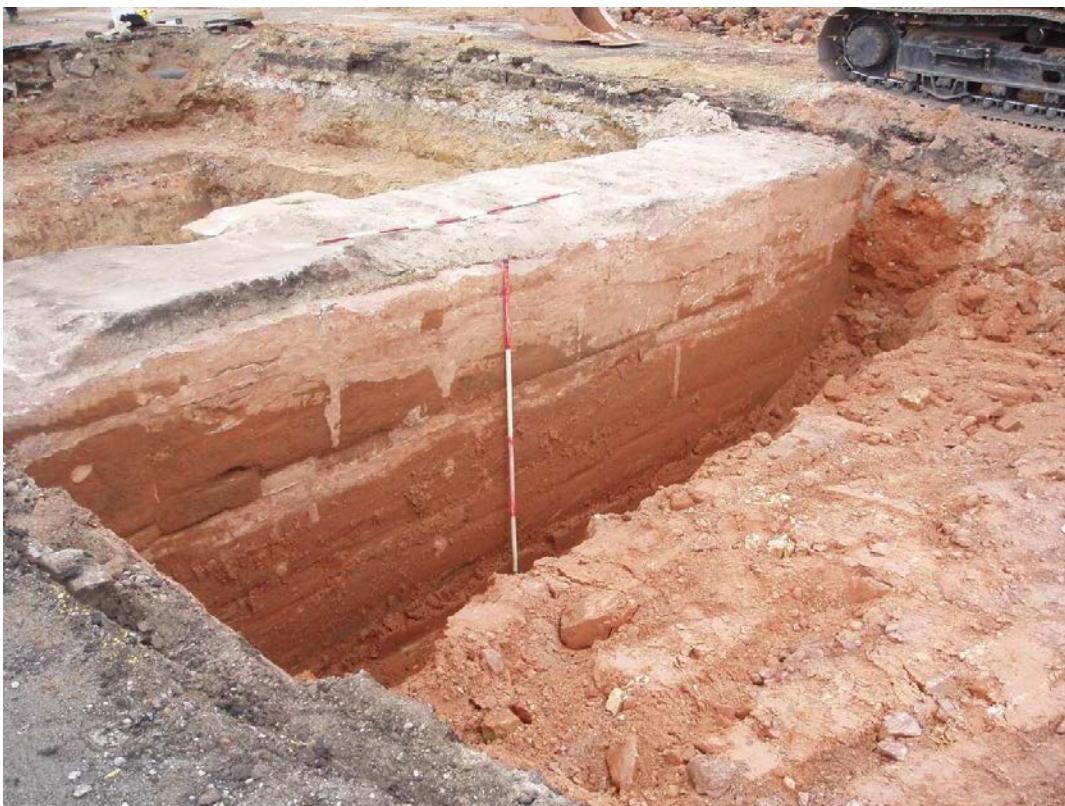
Plate 8: Trench 403, showing the front face of the north wall of Manchester Dock, 3000 , looking north-east
