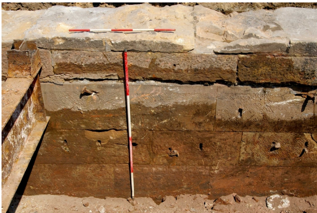
Plate 4: View of Trench 401 showing the front western face of Manchester Dock wall, 3109 , with part of the girder structure 3121 , looking east
