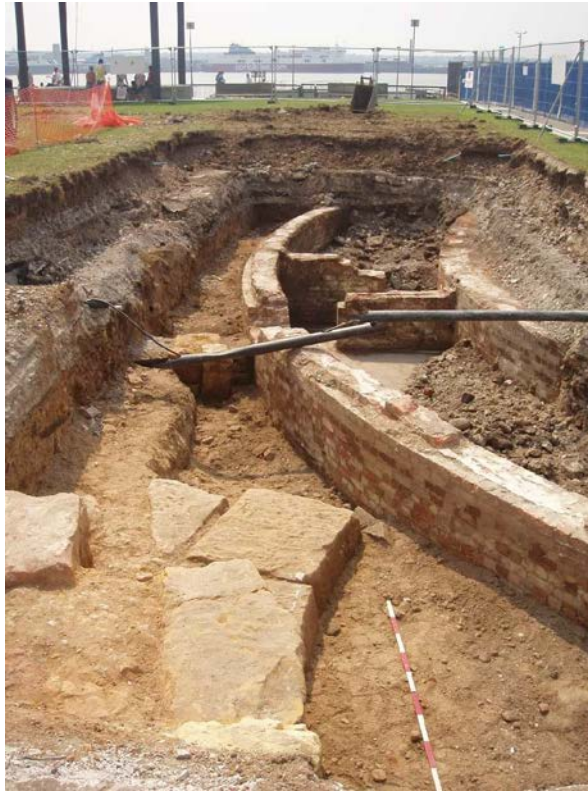
Plate 15: Trench 407, showing the curving sandstone wall 3015 of George's Basin and the later curved brick walls 3024 and 3030 , looking west
