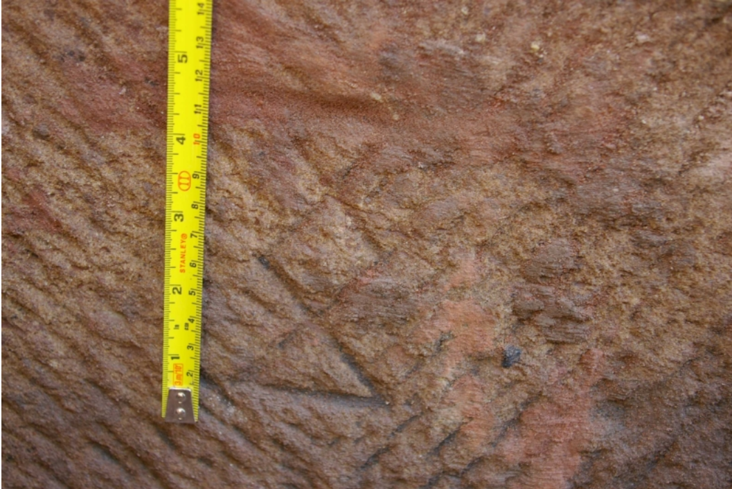
Plate 5: View of Trench 401 showing a close up of a mason's mark on the western face of Manchester Dock wall, 3109 , looking east
