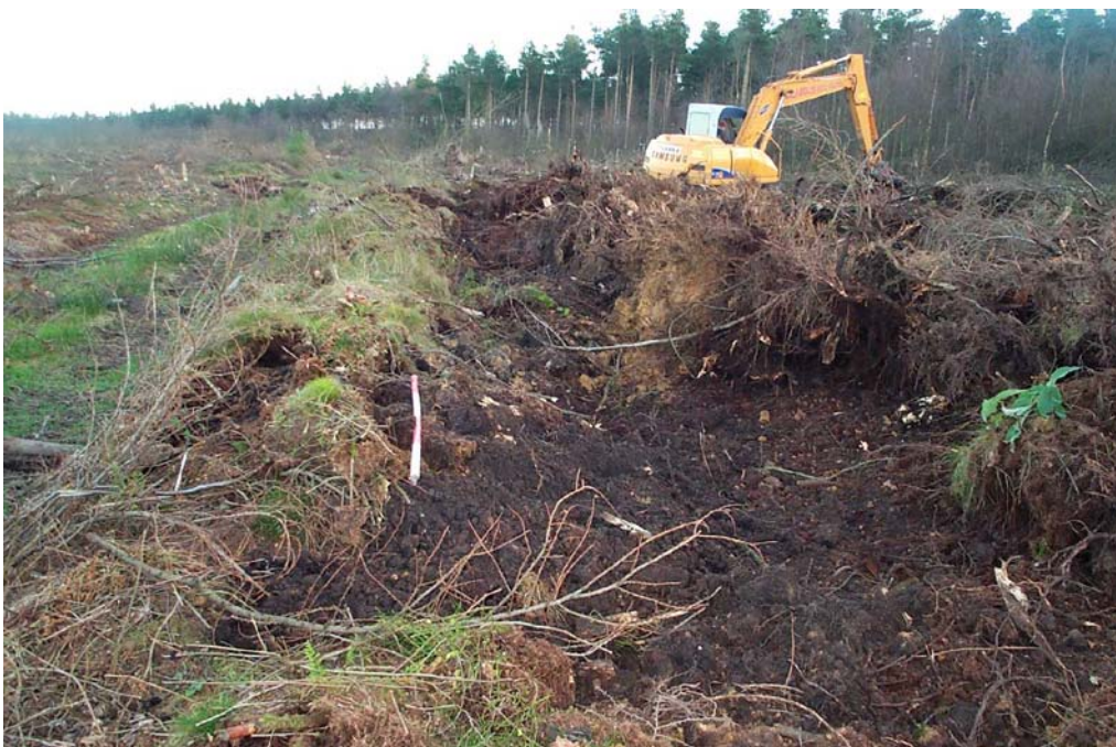
Plate 4: Excavation of tree stumps adjacent to the central ride, looking north
