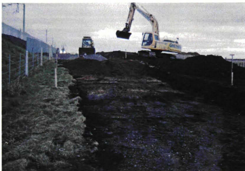
Plate 1: Topsoil stripping, haul road 5
