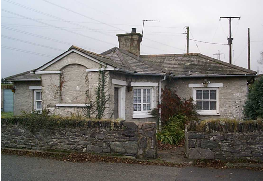
Plate 1 Lon Isa toll house looking west
