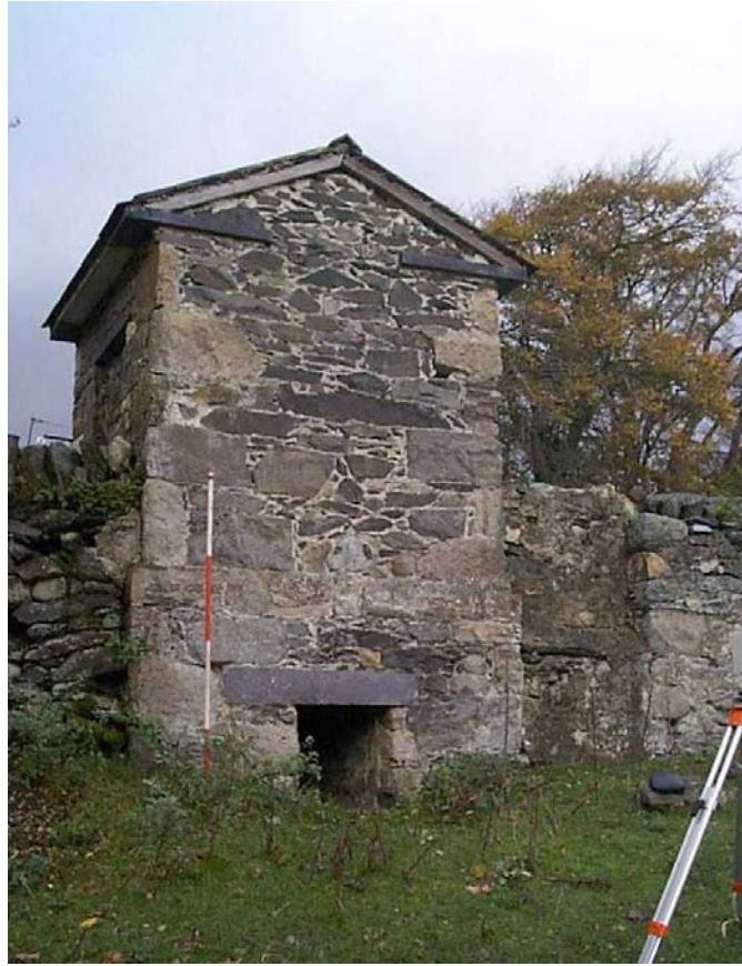
Plate 3 Rear of Lon Isa weigh house – looking west
