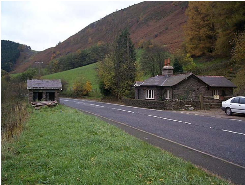
Plate 4 Ty Isaf toll house and weigh bridge
