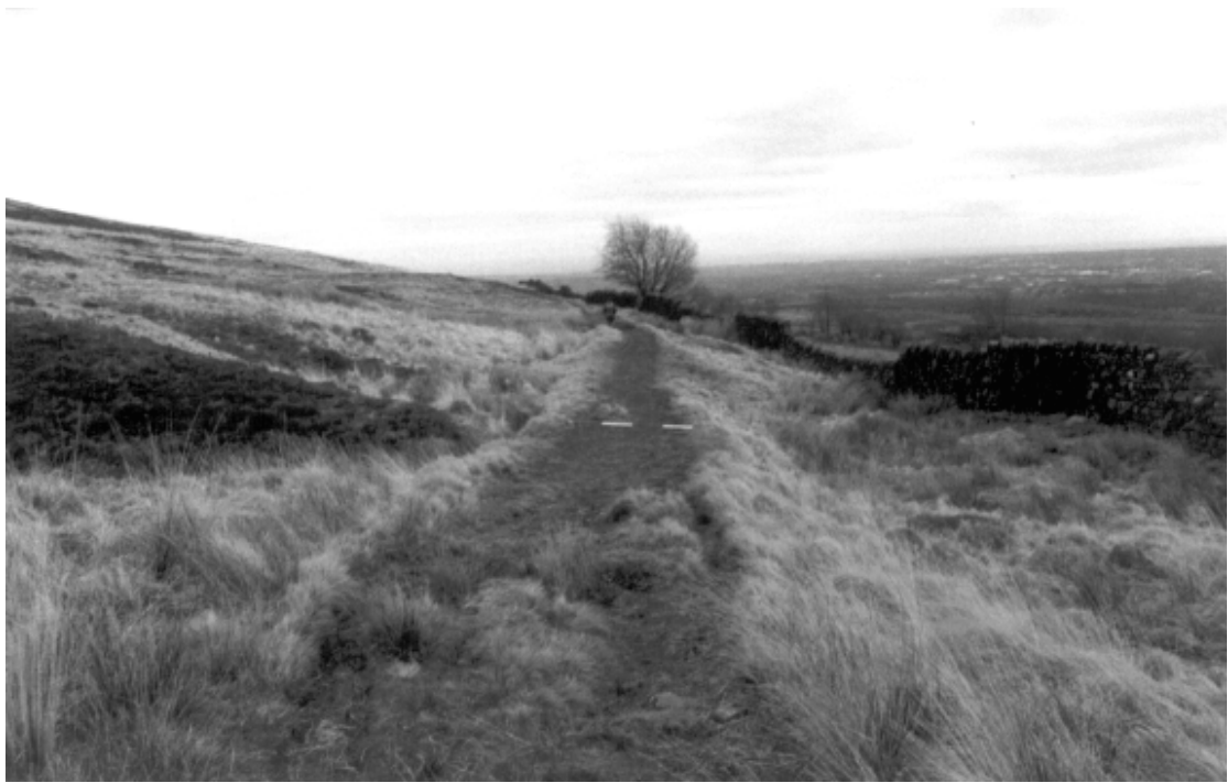
Plate 5: Site 19, probable tramway looking south-east
